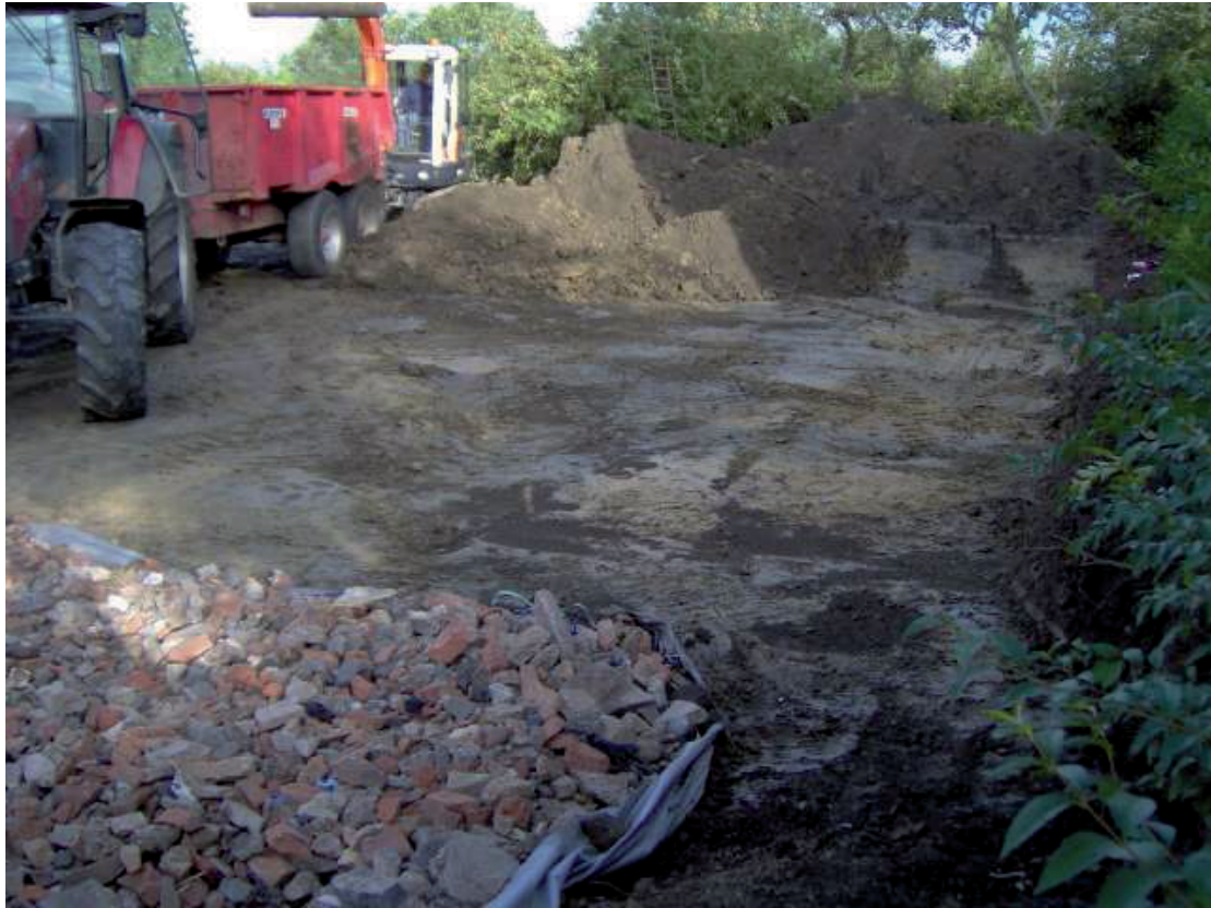
Plate 1: Site after stripping to natural, looking north west
