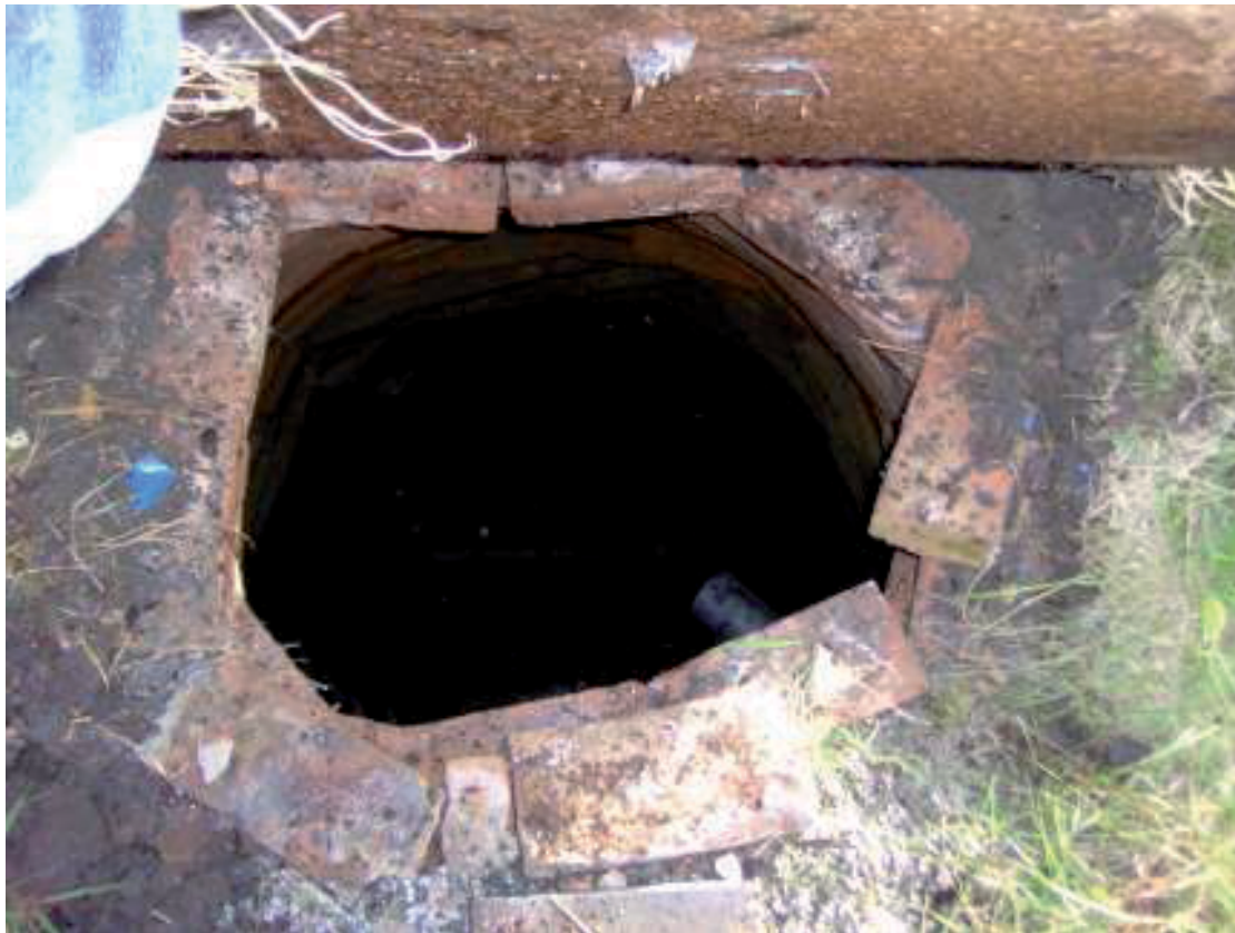
Plate 4: Brick well close to current building
