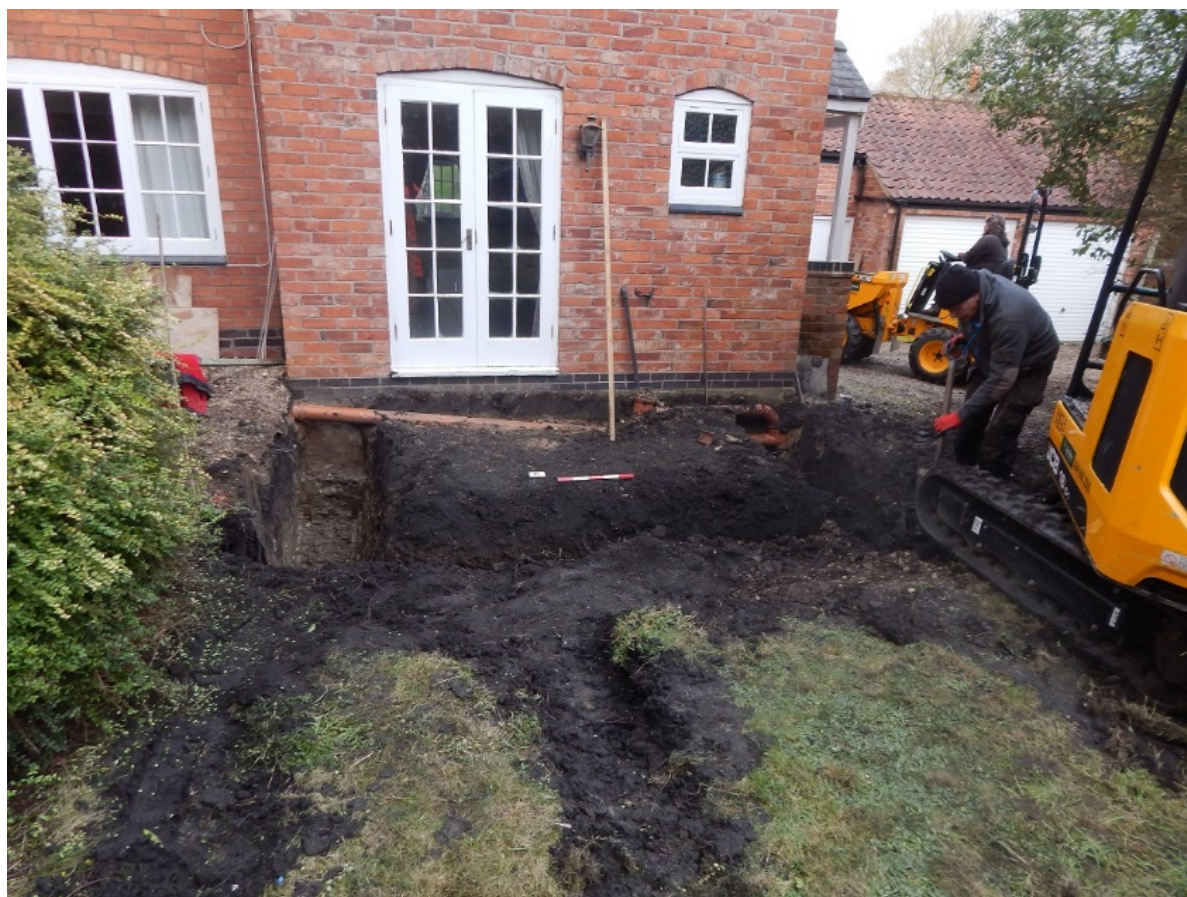
Figure 9: Trenching complete, looking north-east
