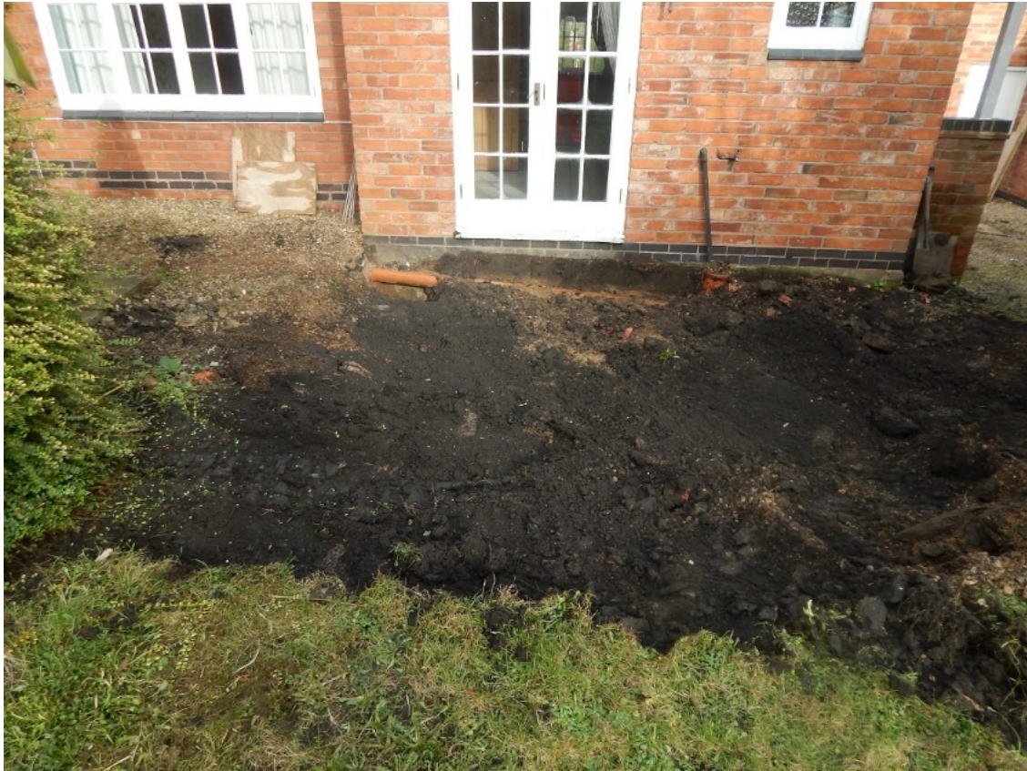
Figure 6: Extension area stripped, looking north-east
