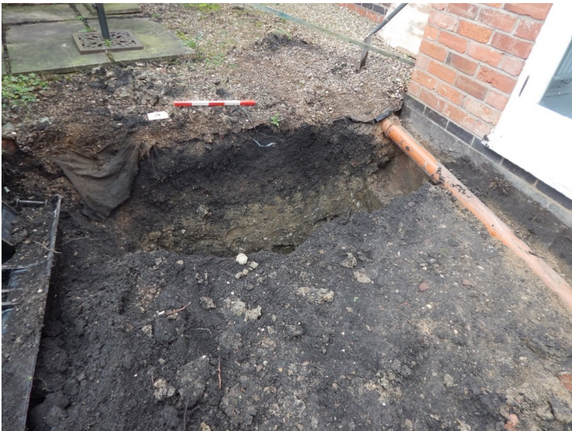
Figure 7: Western trench, post excavation, looking north-west
