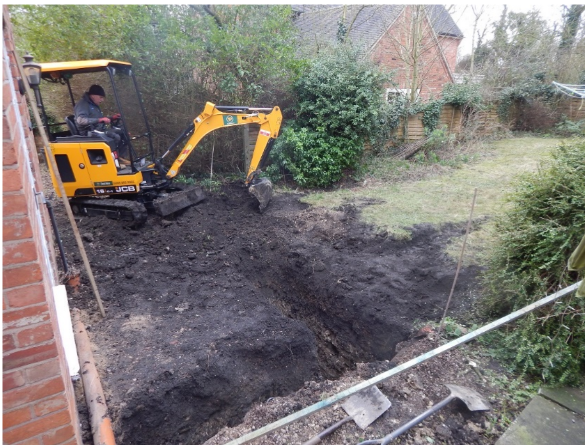
Figure 5: Work in progress, looking south-east
