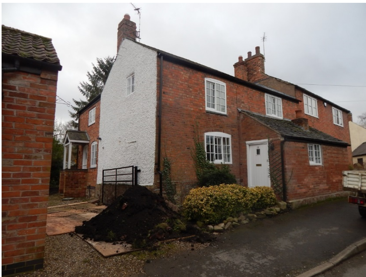
Figure 3: Bakers Cottage from King Street, looking south-west
