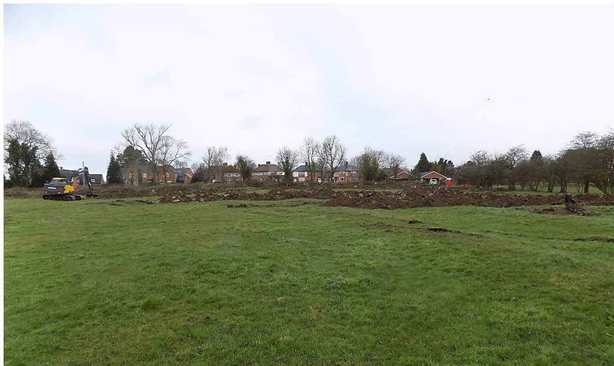
Figure 4: Machining in progress: view north
