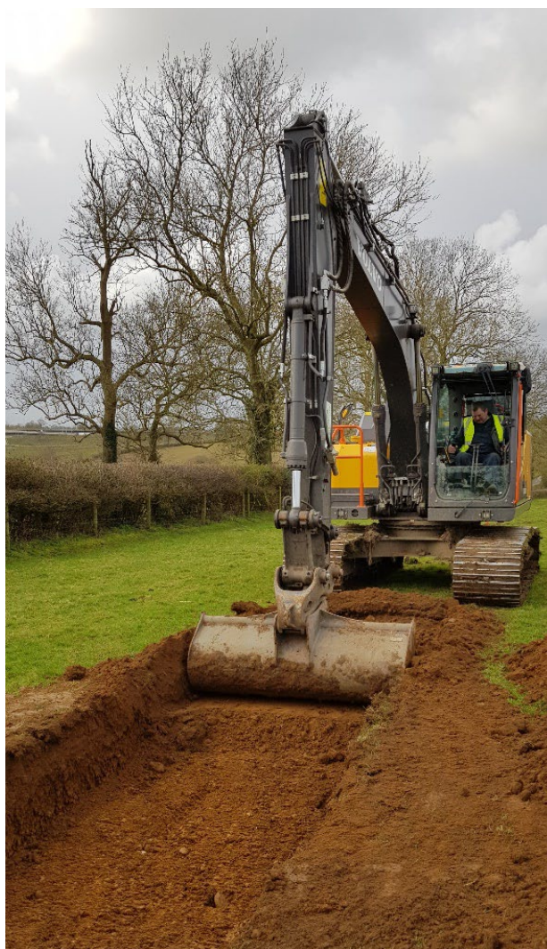
Figure 4: Machining in progress: view north
