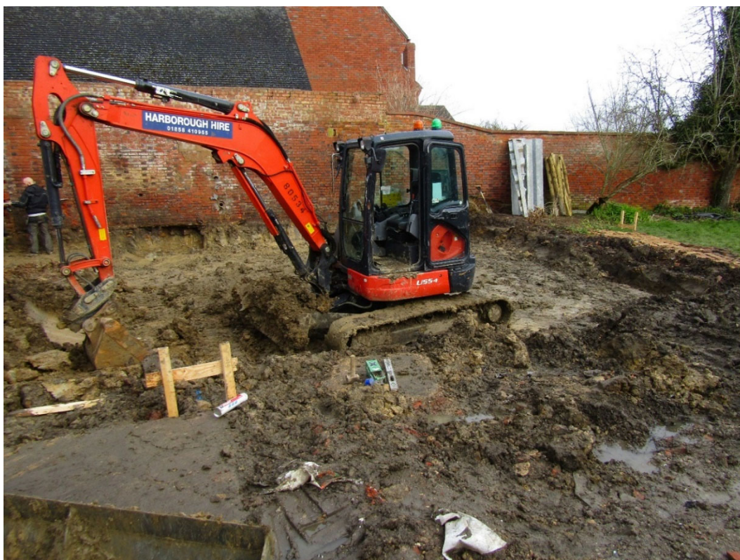
Figure 4: Extension area stripped of hard standing, looking north
