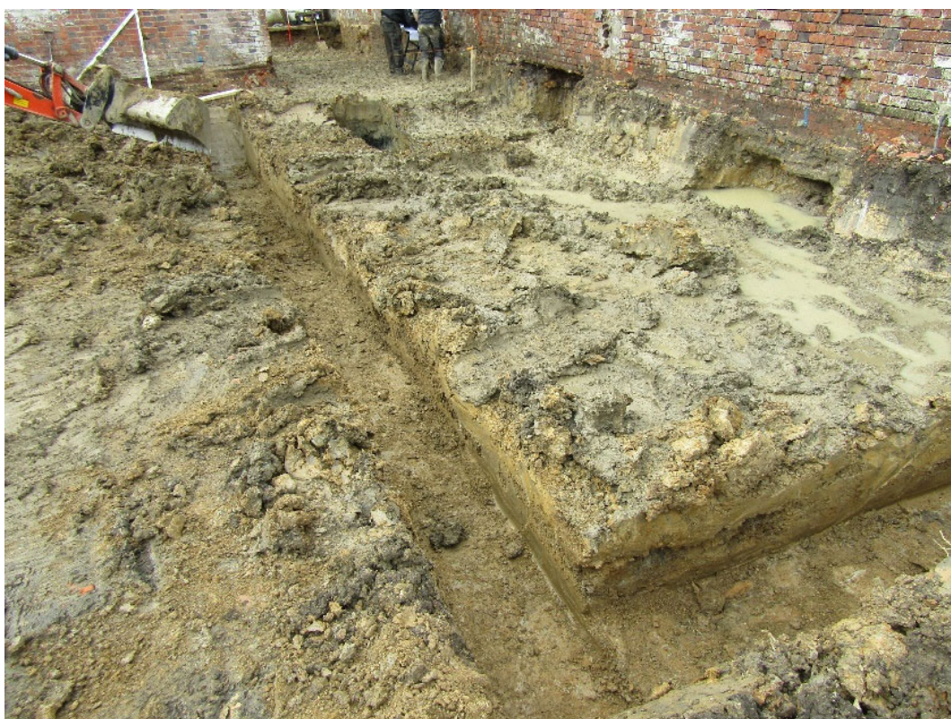
Figure 7: Foundation trenches at the centre of the site looking west
