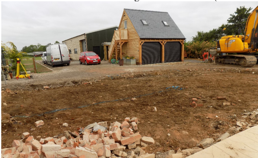
Figure 5: Looking north across the site, prior to excavation
