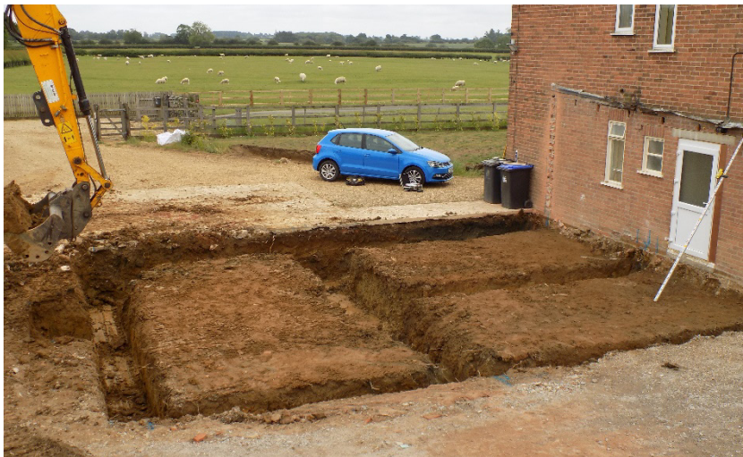
Figure 9: Looking south over the completed foundation trenches
