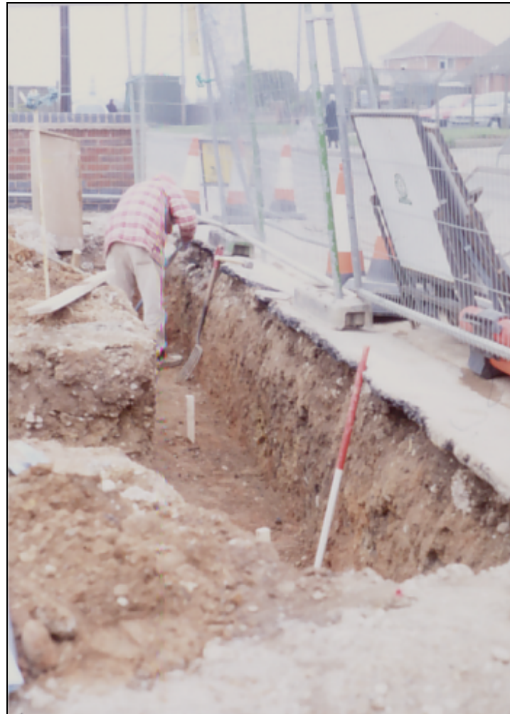
Plate 1 showing feature located during Phase C next to Mill Lane
