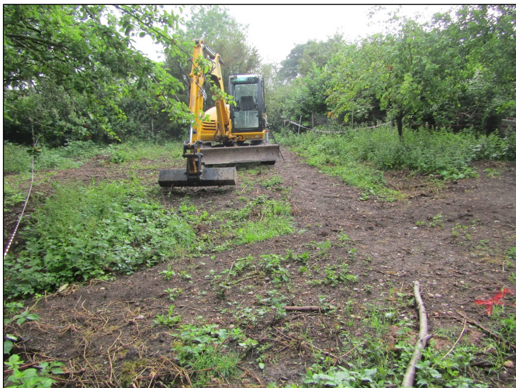
Figure 3: Development area looking north east, prior to excavation.
