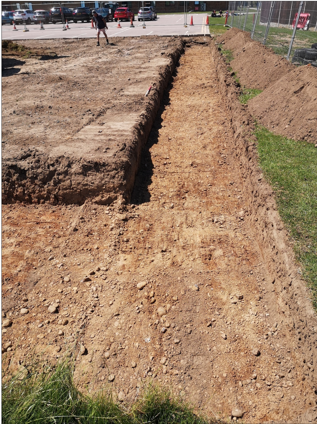
Fig. 7: Trench 3 along north edge of site, looking west
