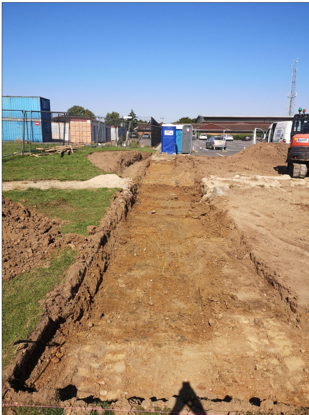
Fig. 6: Trench 2 along south edge of site, looking west
