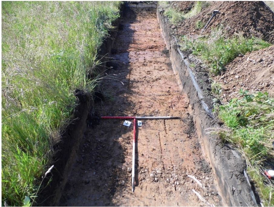
Figure 12: Trench 9 looking southeast
