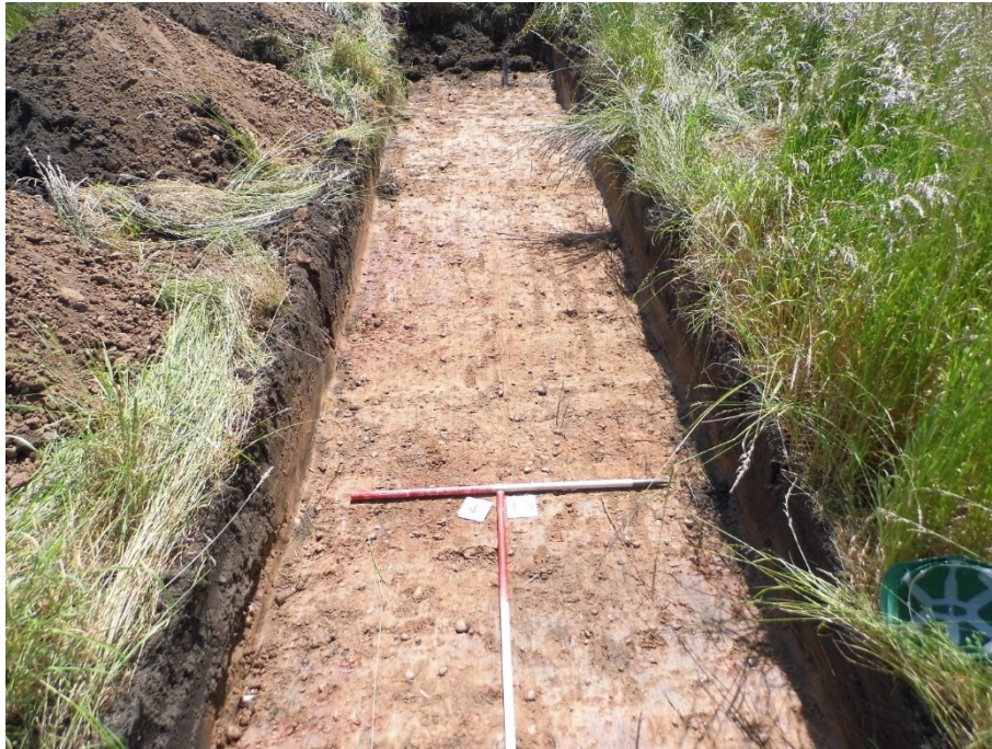
Figure 16: Trench 13 looking southeast
