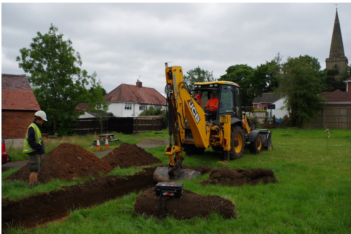
Figure 3: Machining Trench 1, looking south-east
