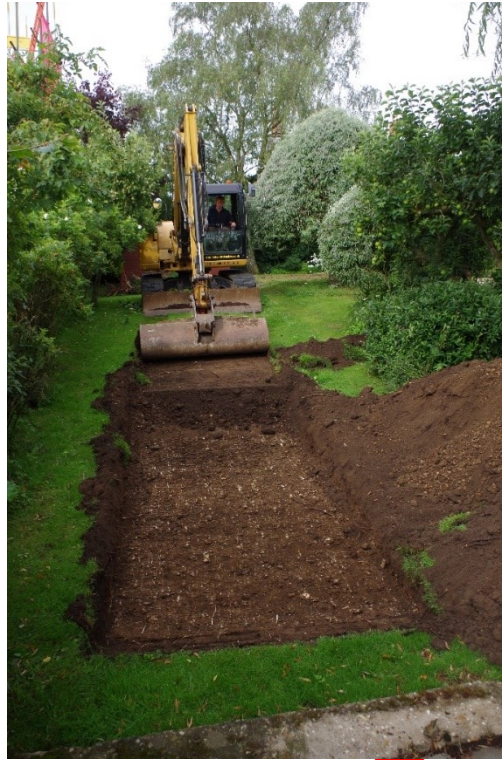
Figure 3: Machining Trench 01, looking west
