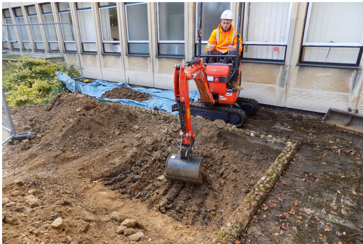
Figure 4: Work in progress excavating Trench 3.
