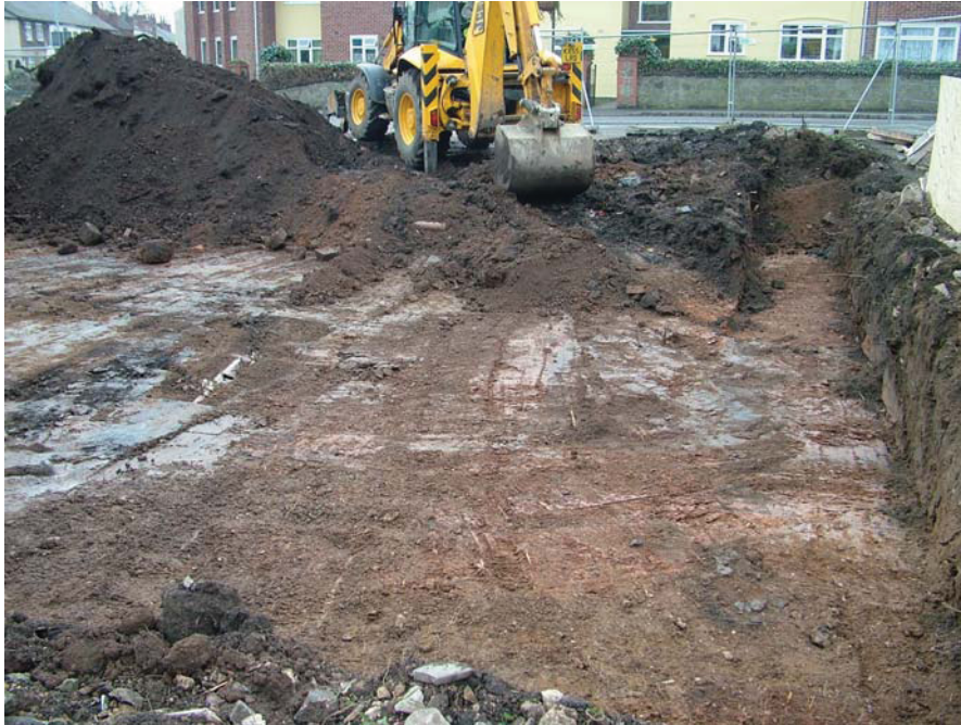
Colour Plate 1 Work In Progress.
