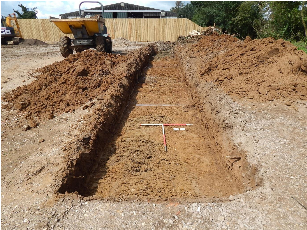
Figure 9: Trench 05, post excavation, looking west
