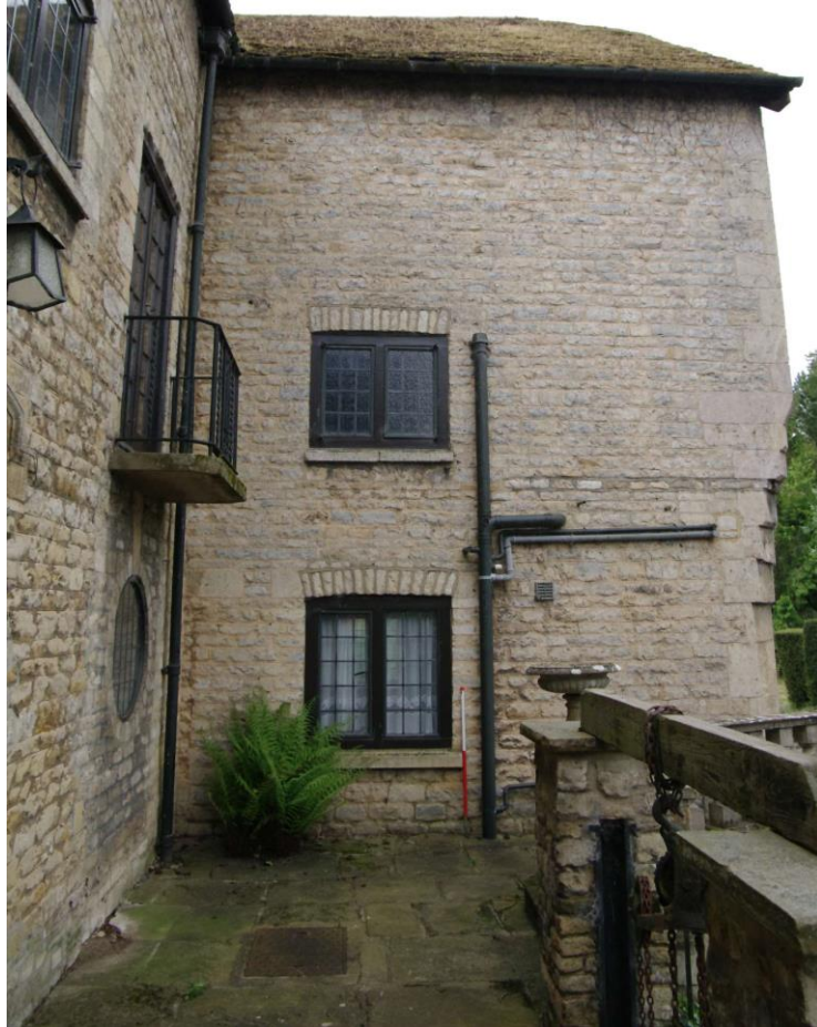
Figure 24: North-east facing end of first mill building Looking south-west. 1m scale. Sluice gate to internal wheel in foreground left
