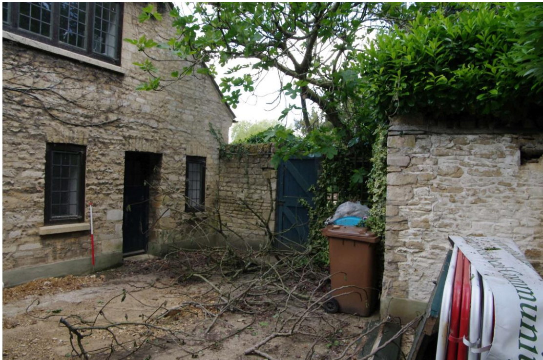
Figure 37: Roofless outbuilding seen from the inside Looking west. 1m scale
