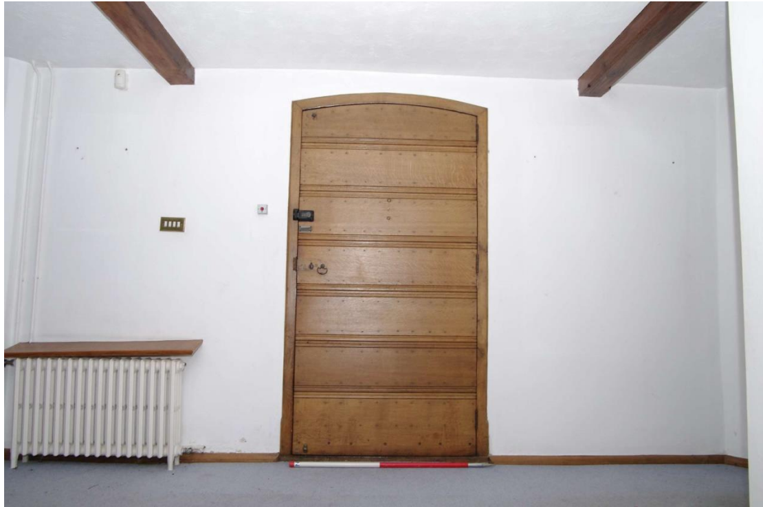
Figure 66: Room G3, front door detail Looking north-west. 1m scale
