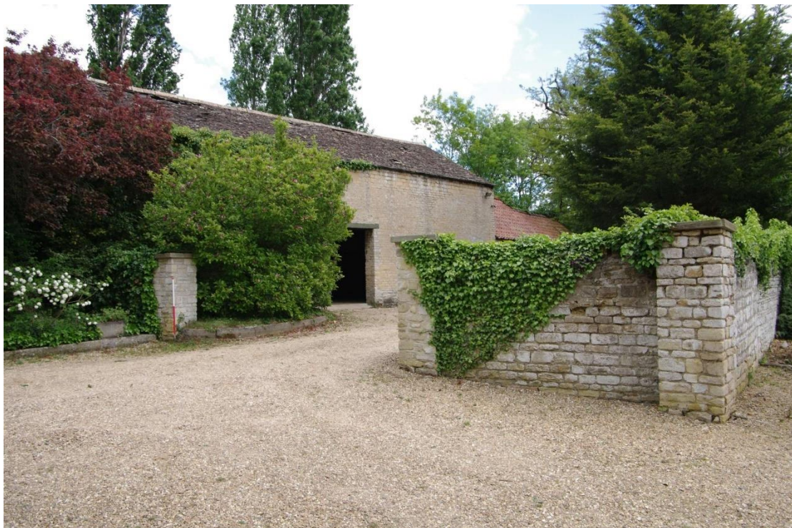
Figure 115: Courtyard entrance to barn and outbuildings Looking east. 1m scale. The mill buildings are out of shot to the right of the picture
