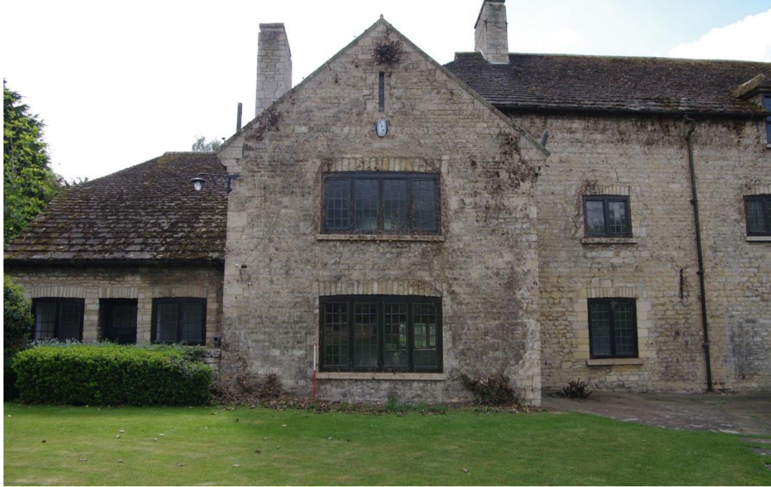
Figure 33: North-west facing elevation, north gable end Looking south-east. 1m scale
