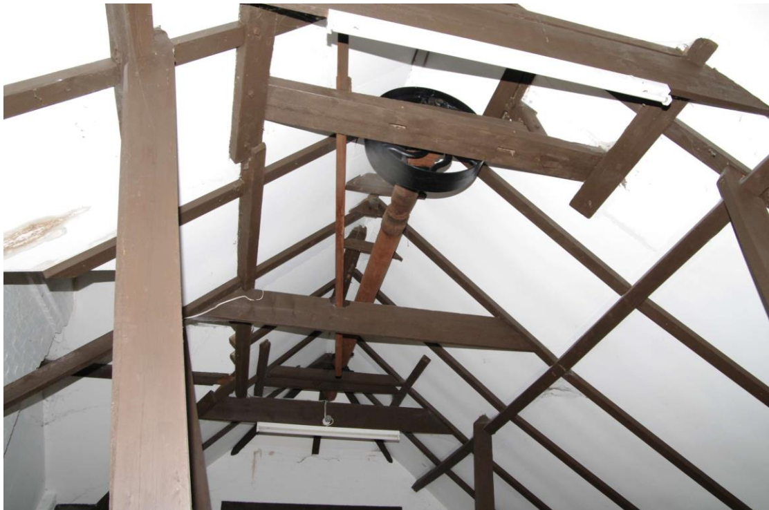
Figure 106: Room R1 sack hoist mechanism Looking north
