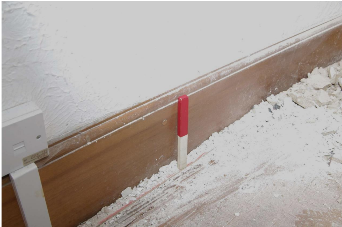
Figure 58: Room G1, skirting board detail 0.2m scale
