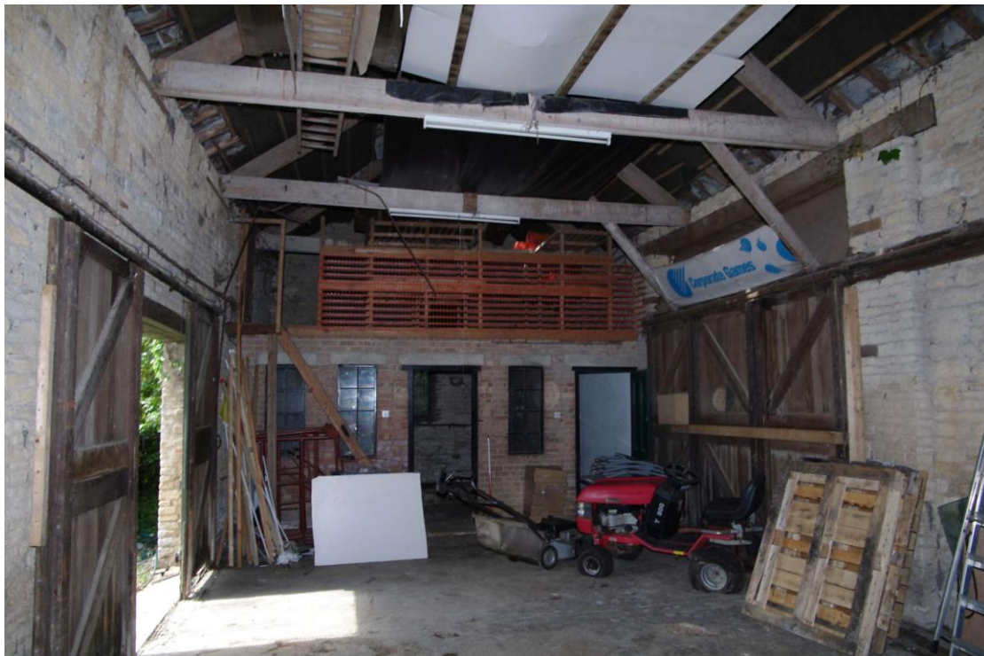
Figure 124: Barn interior Looking north-west. 1m scale
