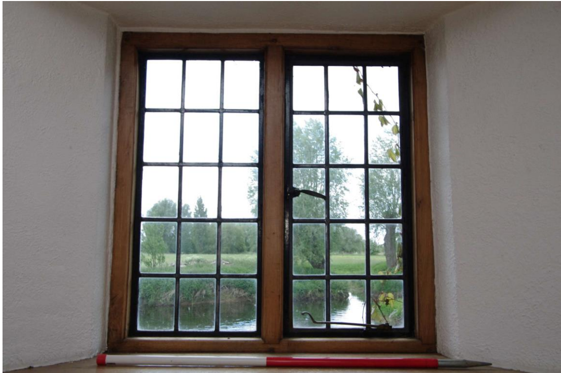
Figure 55: Room G1, south-west wall window detail 1m scale
