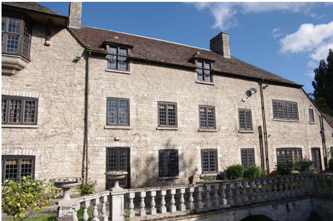
Figure 45: Central part of the south-east facing elevation Looking north
