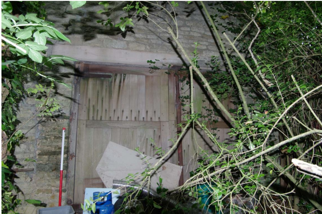
Figure 122: South-east facing elevation of outbuilding Looking north-west. 1m scale
