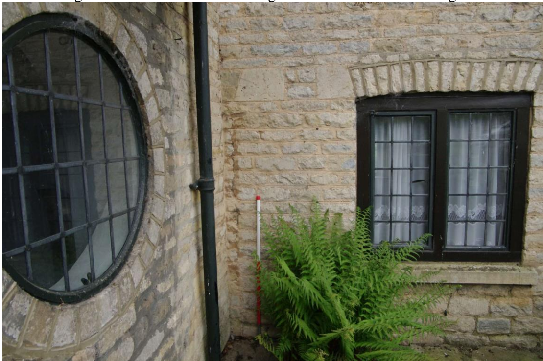
Figure 25: Blocked doorway on NE facing side of the first mill building Looking south-west. 1m scale. The blocked door and lintel are partially visible in the corner to the left of the scale
