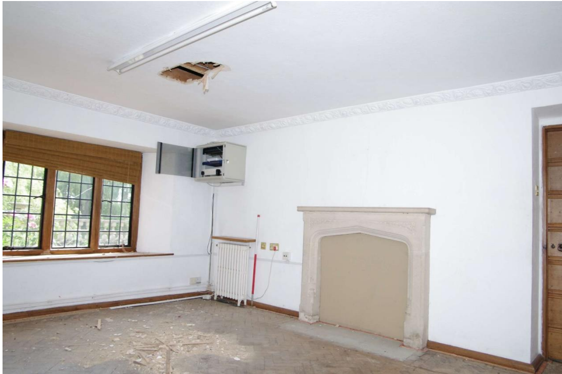
Figure 72: Room G7 Looking south. 1m scale. Door to G6 on right
