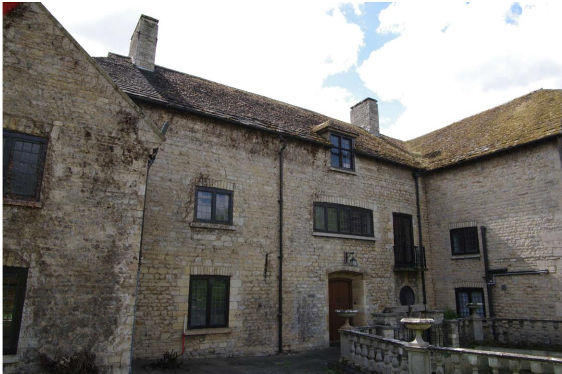
Figure 27: Central section of north-west facing elevation Looking south. First mill building on right. The 1729 datestone is above the ground floor window to the left of the door
