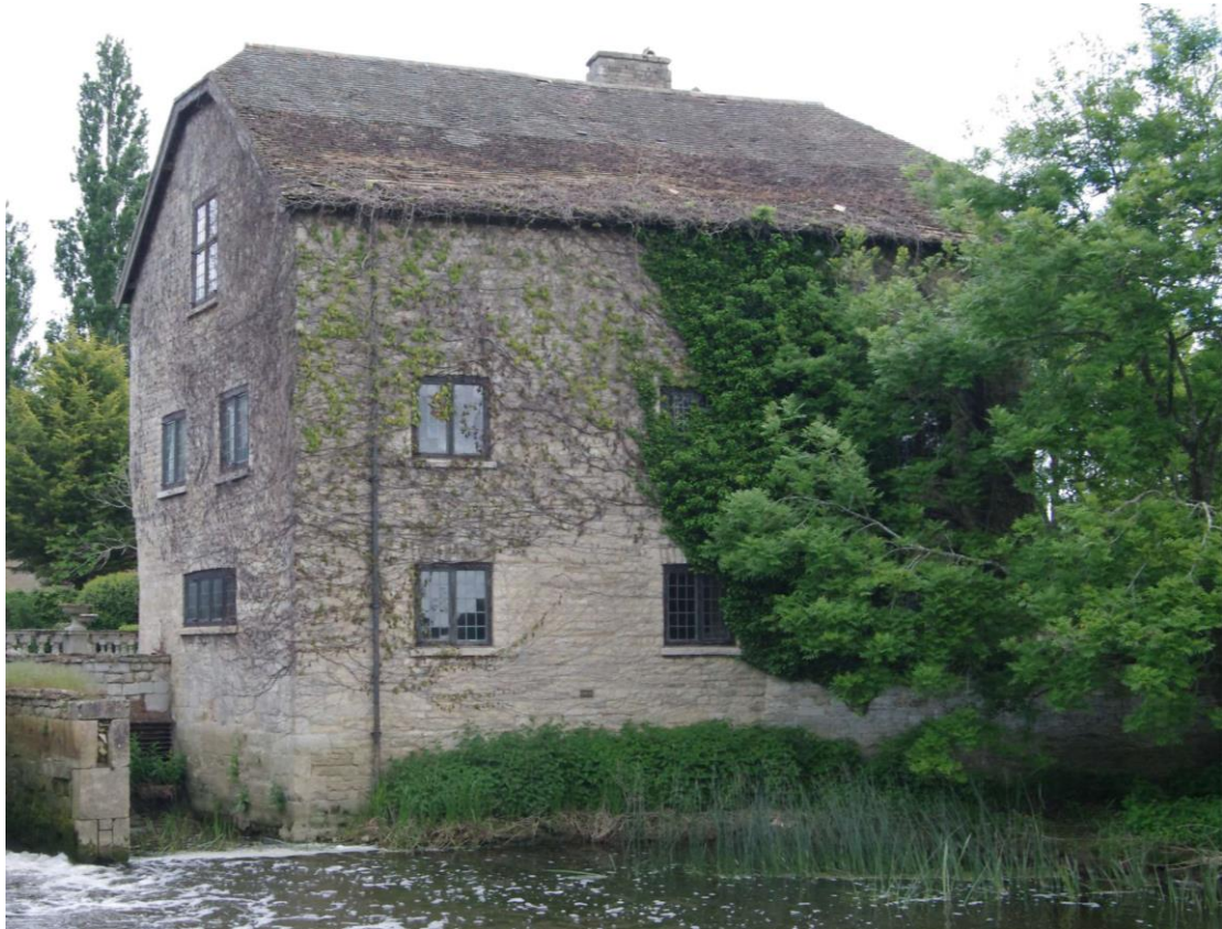
Figure 50: South-west facing elevation Looking north-east
