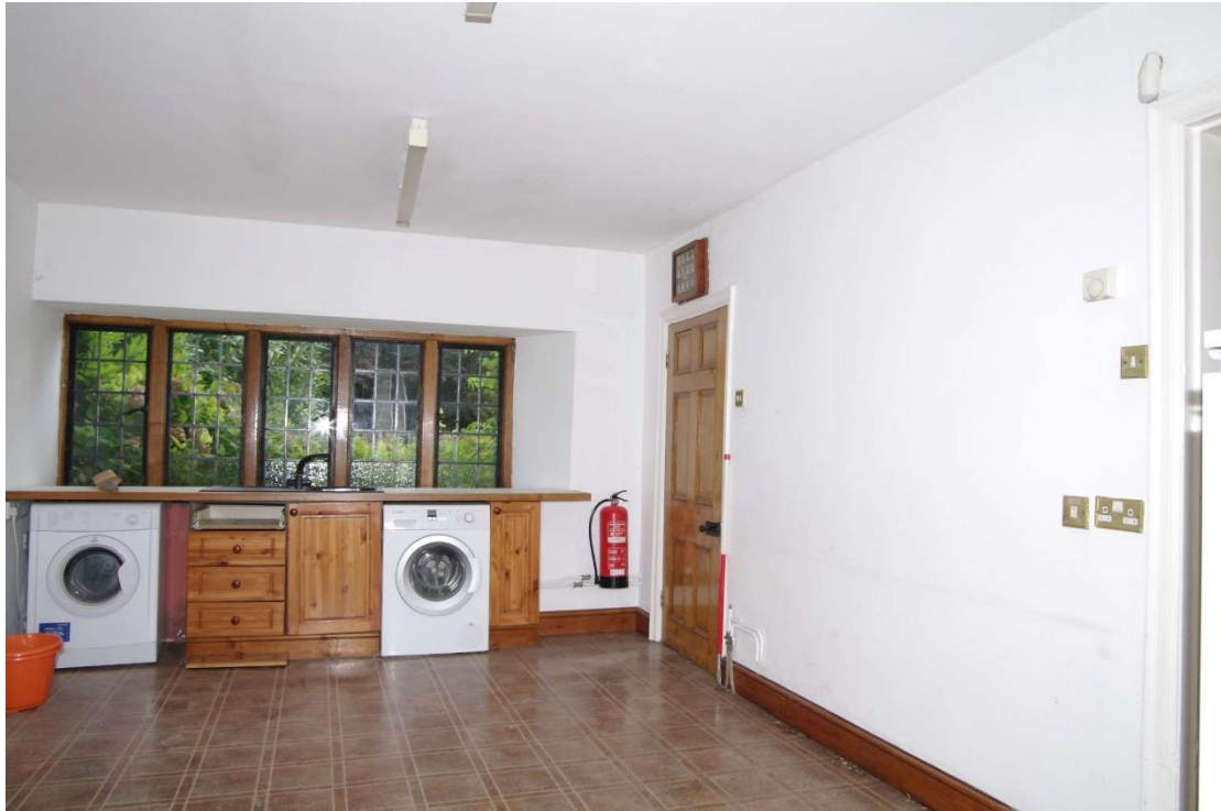
Figure 78: General view of Room G10 Looking south-east. 1m scale. Door on right leads to the service stairs G12. Note the bell panel above this doorway (see Fig. 80 below)
