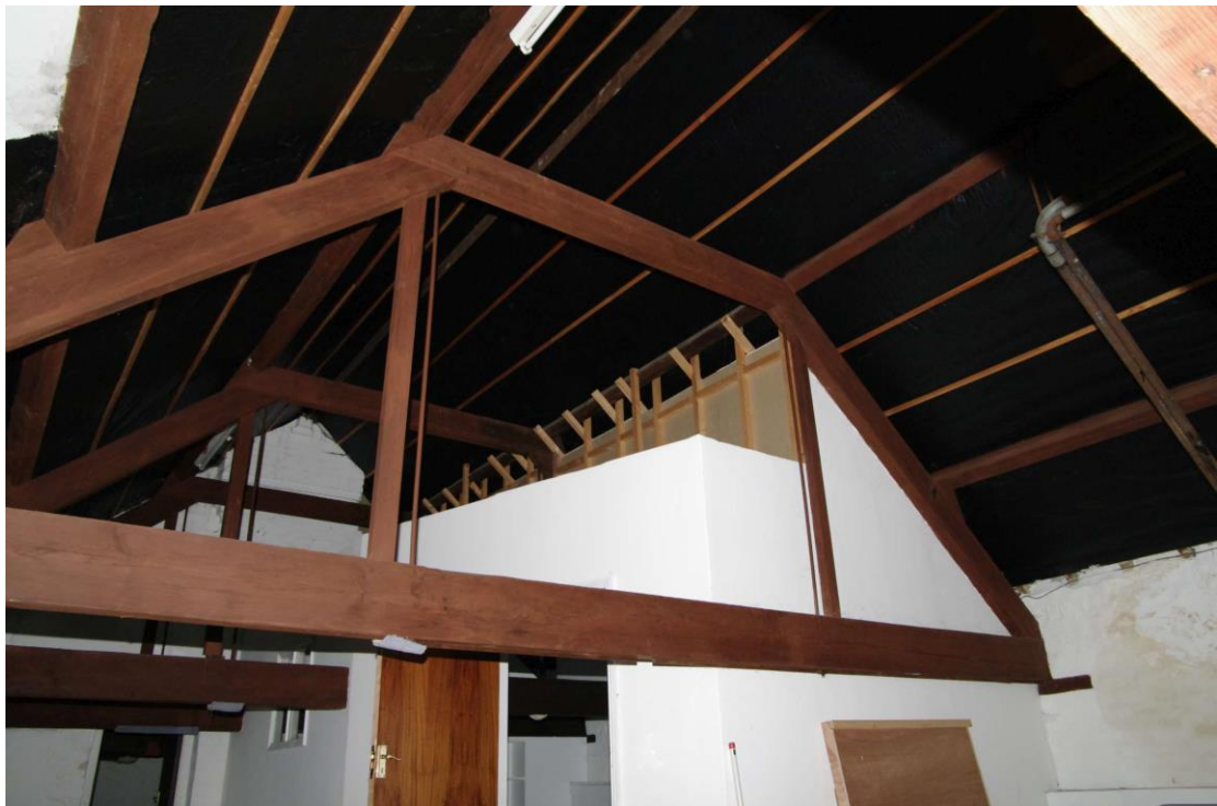
Figure 111: R2 roof structure Looking west
