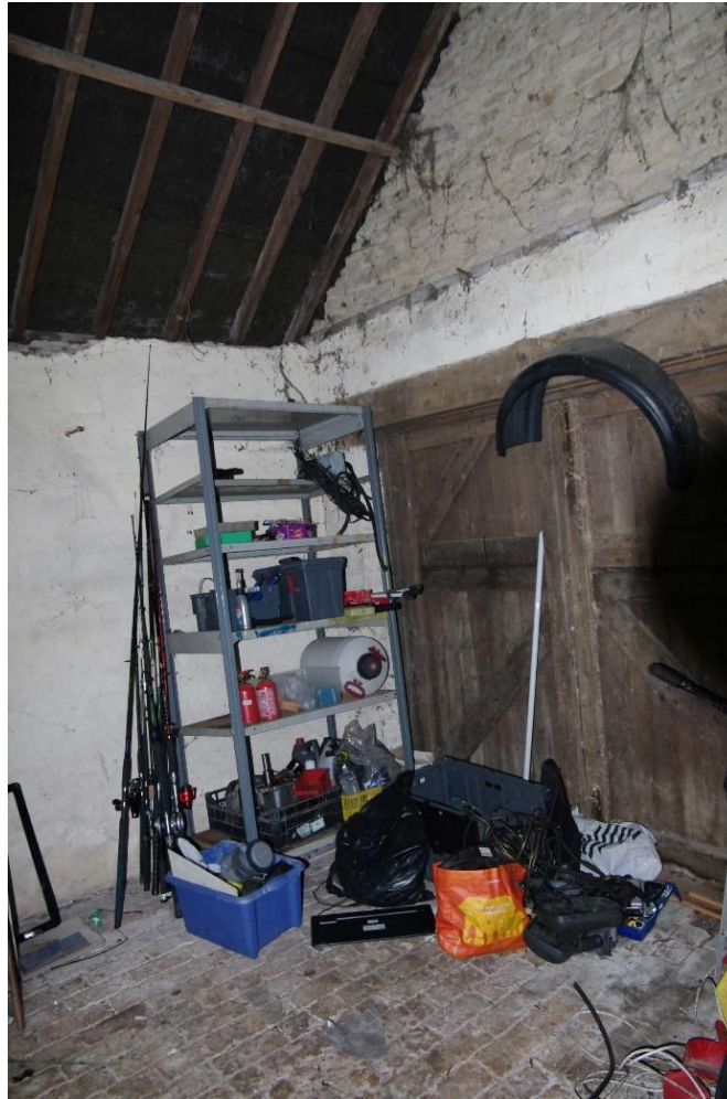
Figure 129: Interior of end outbuilding Looking south-east
