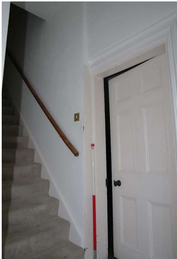
Figure 82: Room G12, service staircase Looking north. 1m scale. Door on right leads to G10
