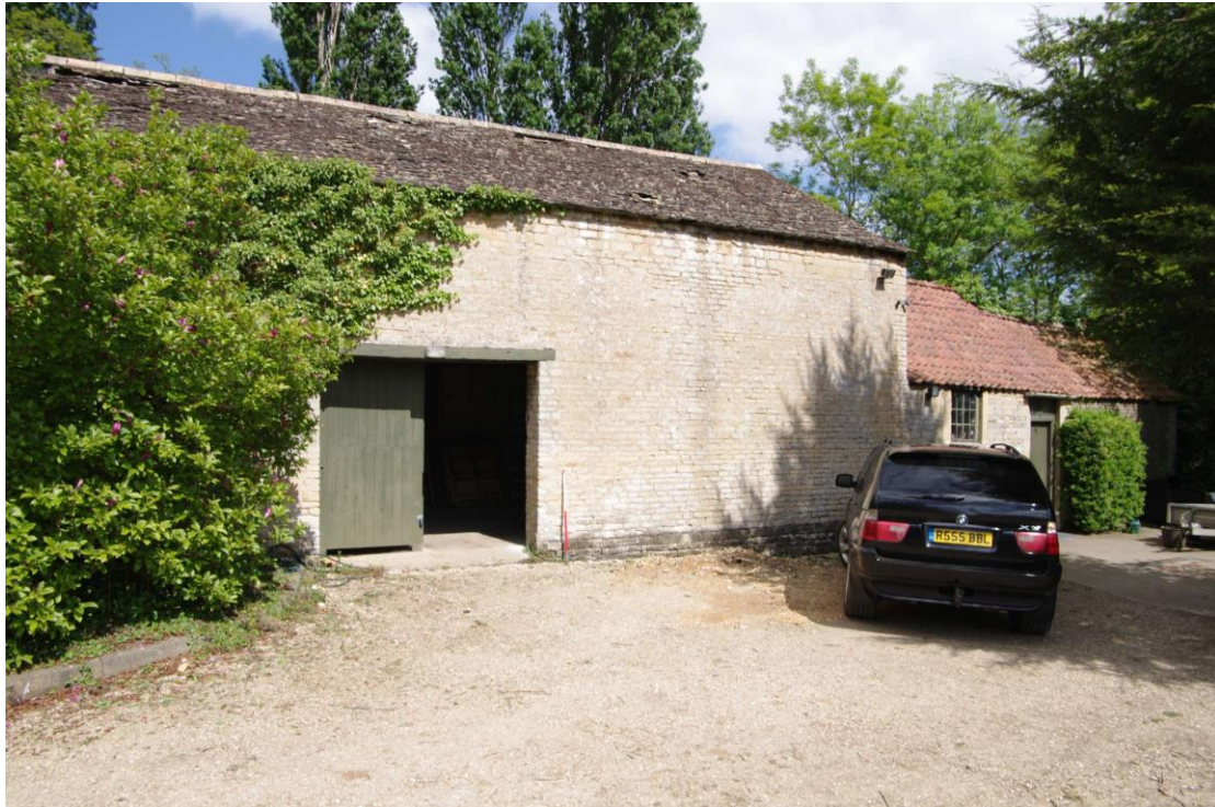
Figure 118: Barn, south-west facing elevation Looking east. 1m scale
