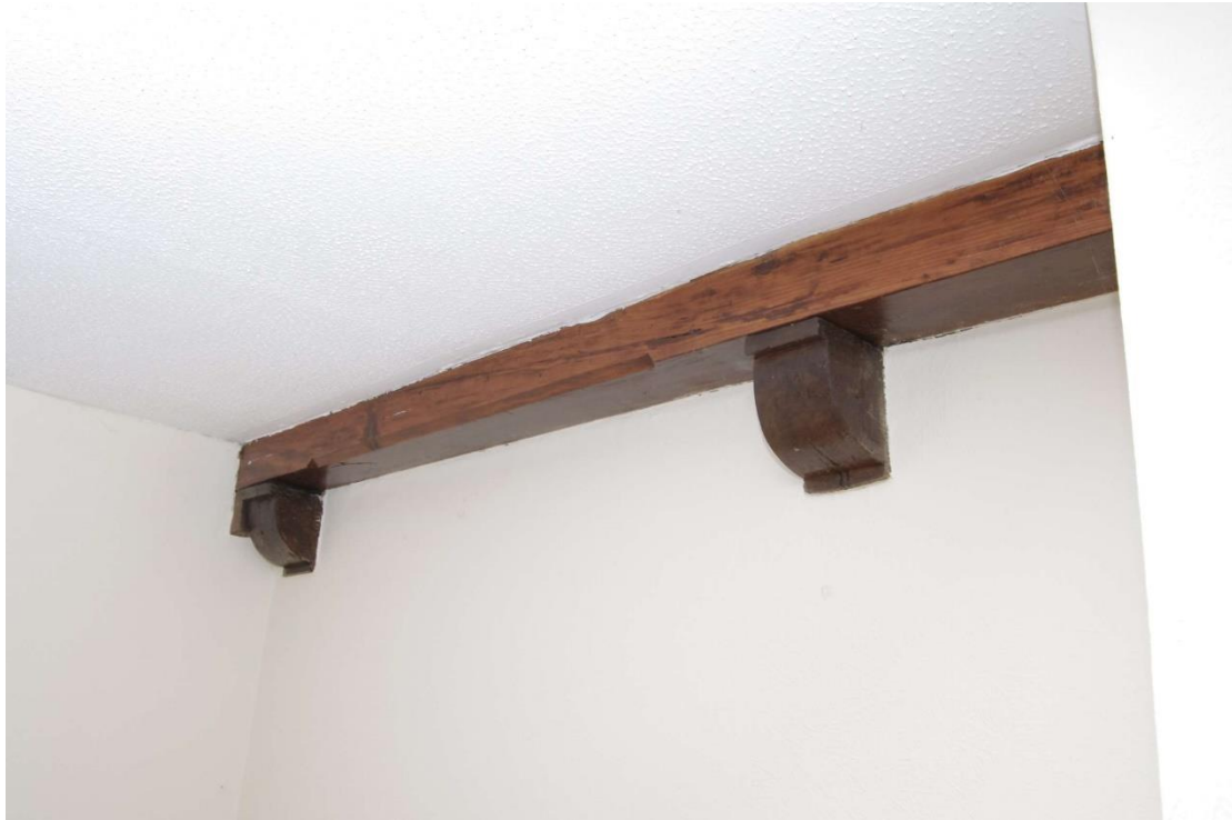
Figure 94: Room F6, beam detail on north-east wall
