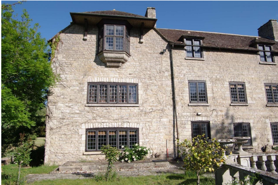
Figure 46: South-east facing elevation of first mill building Looking north-west. 1m scale
