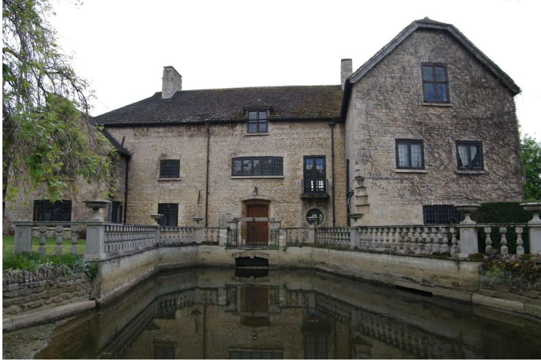
Figure 26: north-west facing elevation Looking south-east
