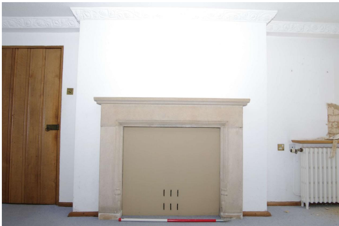
Figure 71: Room G6 fireplace
