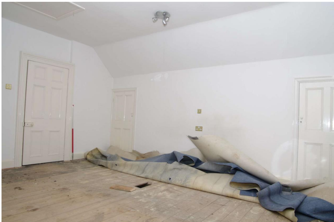
Figure 101: General view of Room F10 Looking west. 1m scale. The two low doors on the right lead into the eaves space
