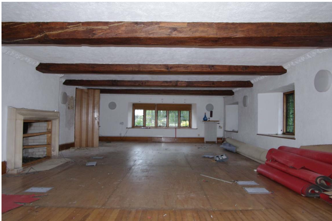
Figure 54: Ground floor G1 Looking south-east. 1m scale
