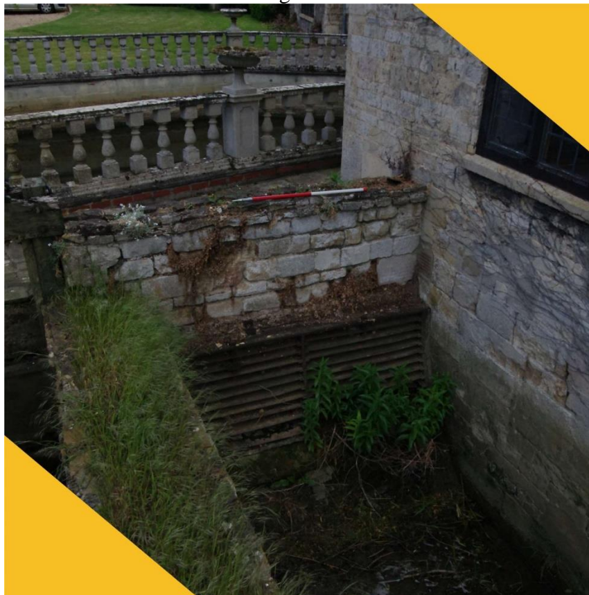
Figure 23: Close-up of wrought-iron grille in wheel pit Looking east. 1m scale
