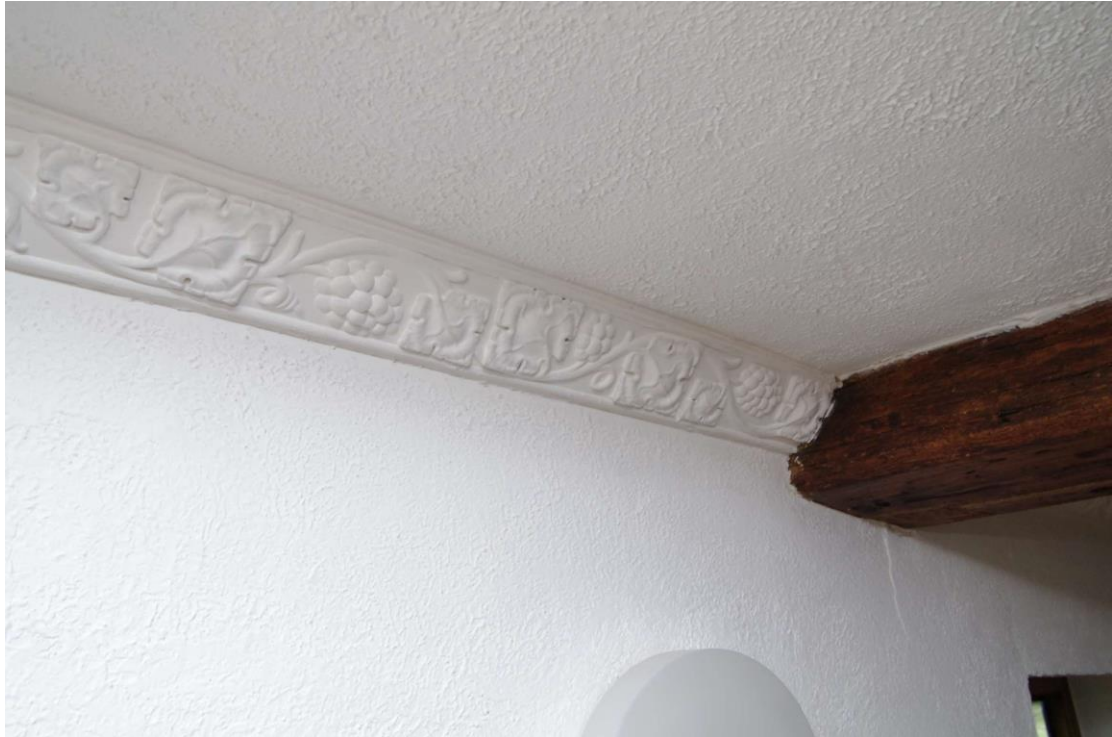
Figure 57: Room G1, plaster decorative detail
