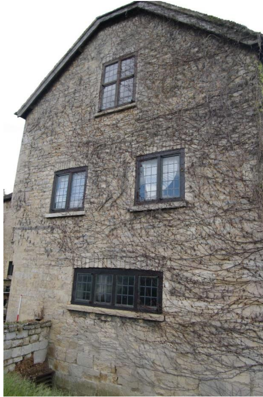
Figure 16: Western gable end of NW facing elevation Looking east. 1m scale
