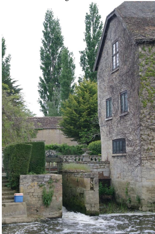
Figure 17: Western gable end of NW facing elevation and bypass sluice Looking north-east. The external mill wheel was located in front of the metal grille
