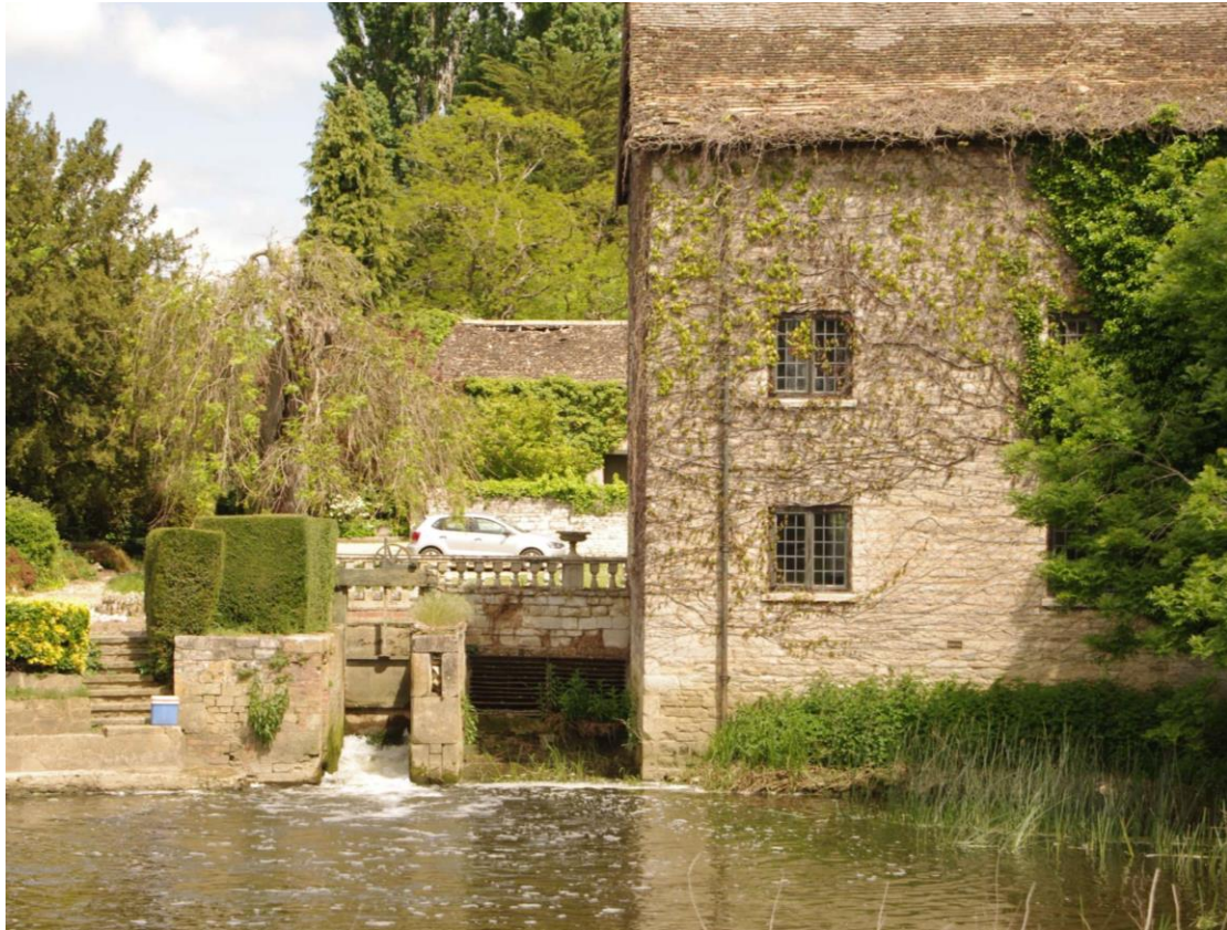
Figure 22: Bypass slice gate and location of former external wheel pit Looking north-east
