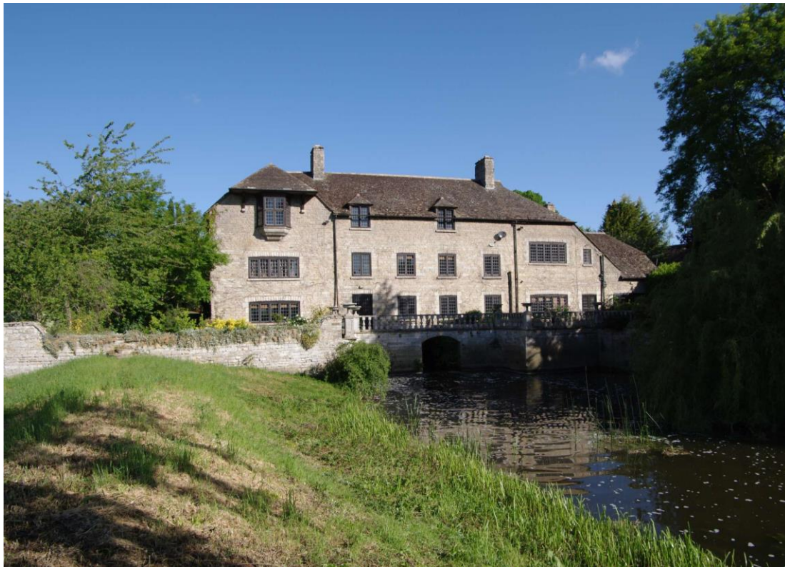
Figure 41: General view of south-east facing elevation Looking north. Taken from the same location as Figure 11
