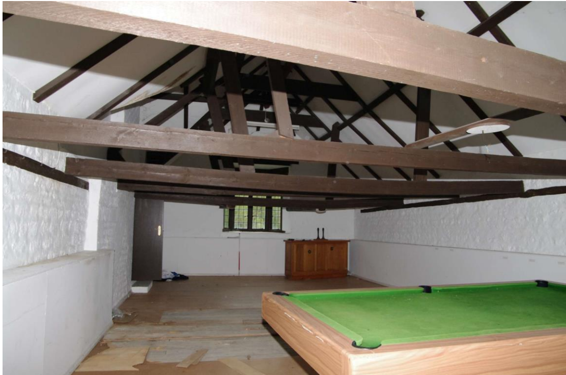
Figure 105: General view of R1 Looking south-east. 1m scale
