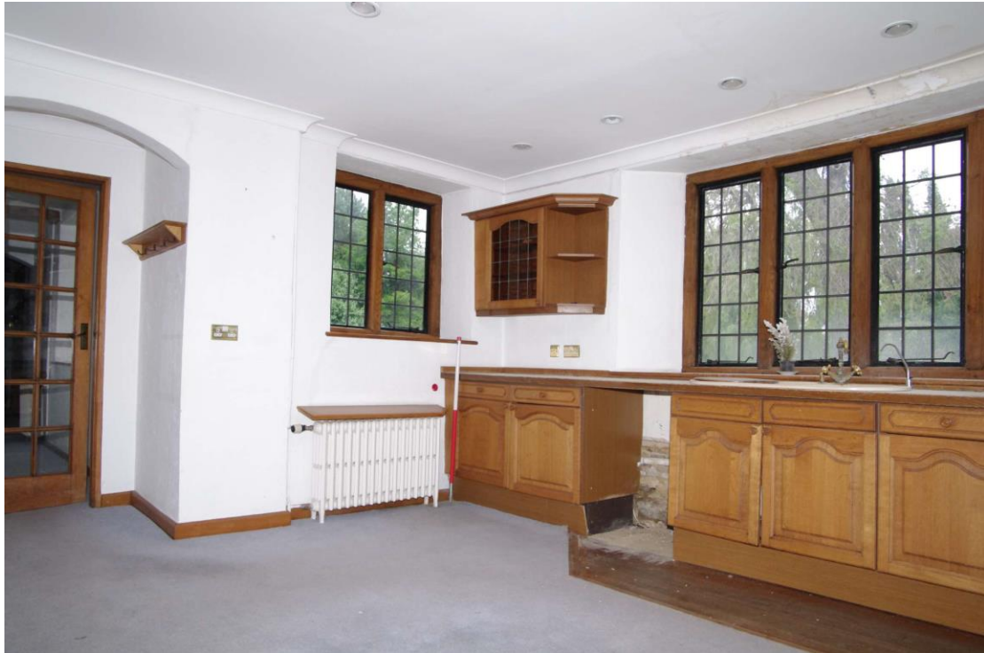
Figure 75: General view of Room G8 Looking west. 1m scale. Doorway to corridor G5 on left
