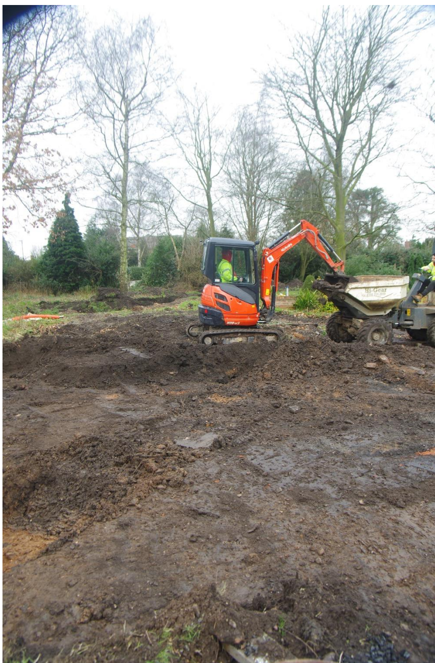
Figure 3 Topsoil stripping, looking north
