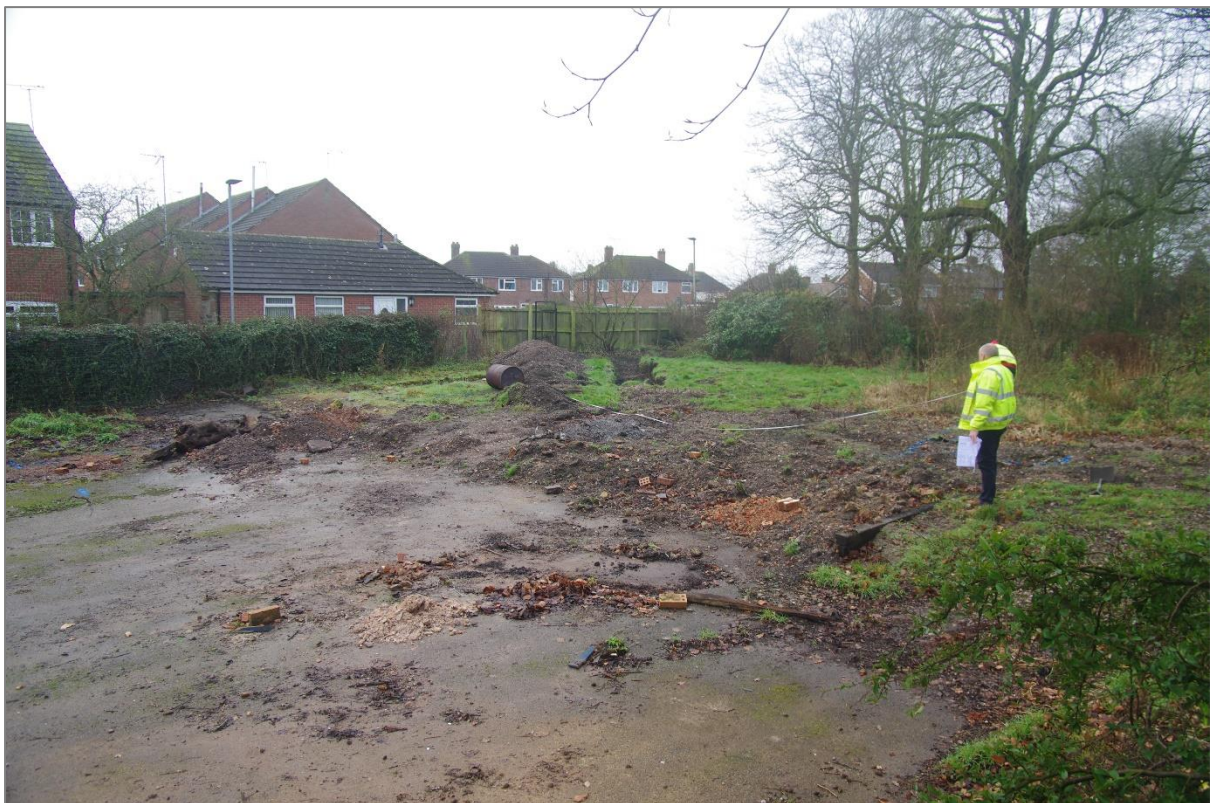
Figure 2 The area before stripping, looking south
