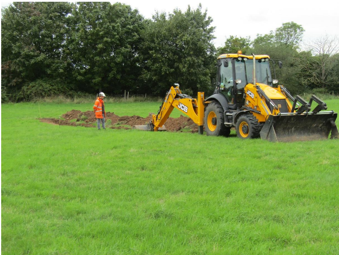
Figure 7: Working shot of trench being excavated
