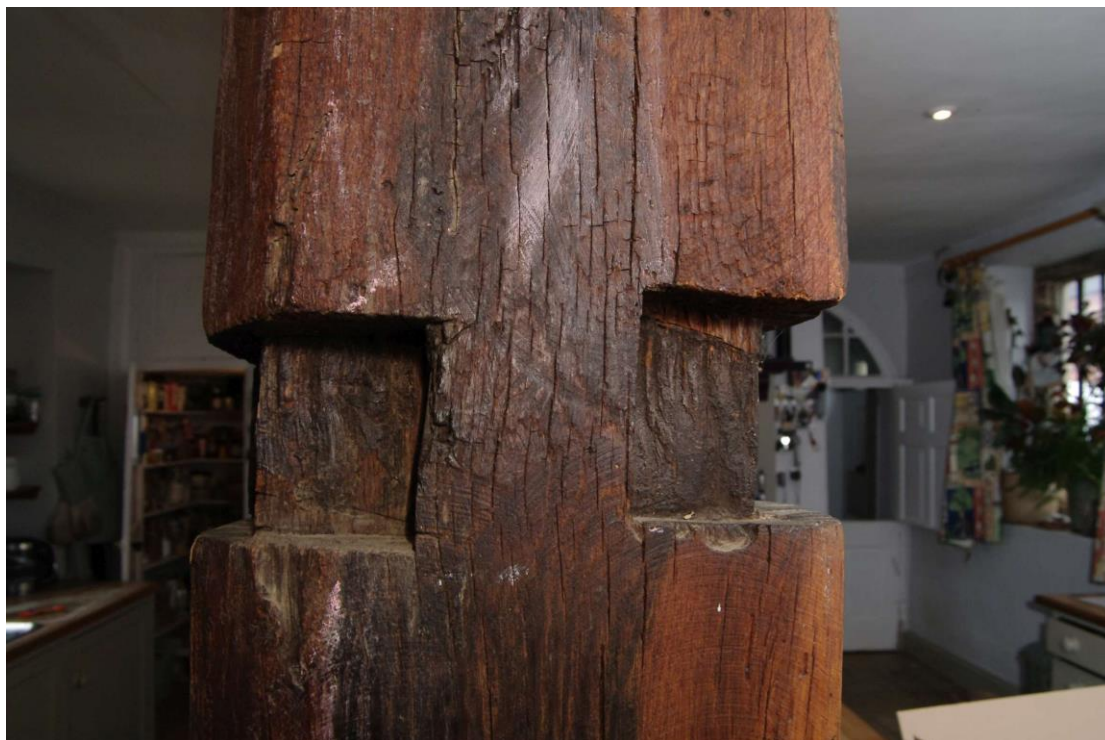
Figure 27 Timber post in kitchen socket detail
