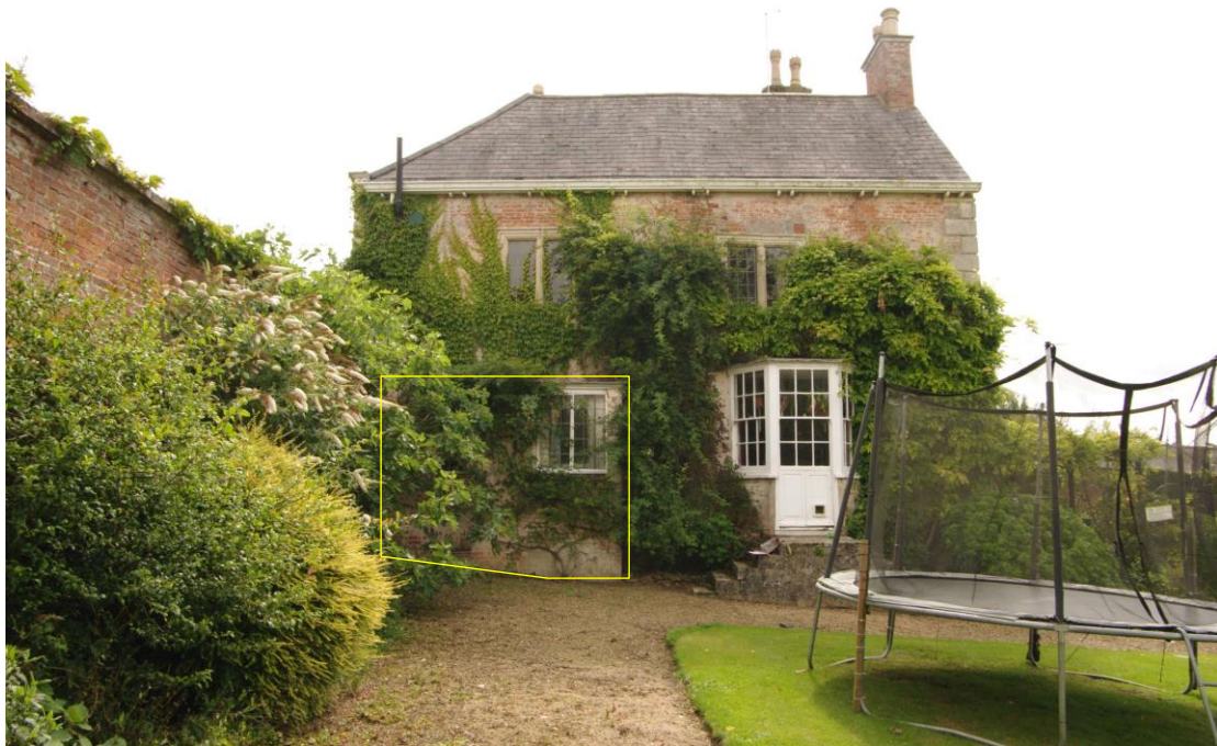
Figure 15 West facing elevation with single storey extension Looking east. The extension is outlined in yellow. The stairs to the right of the extension will be extended northwards
