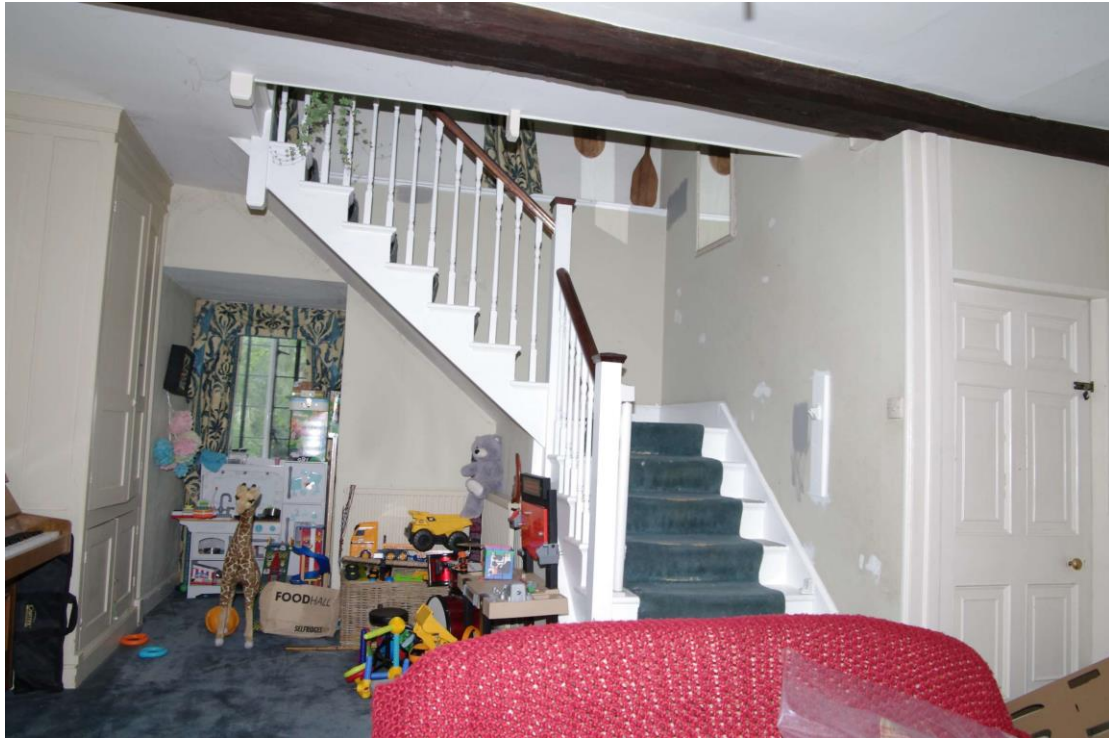
Figure 21 Ground floor stairs with single storey extension below Looking west. Doorway on right leads down to cellar and toilet seen in Fig. 20. The window beneath the stairs is the larger window seen in Fig. 16.
