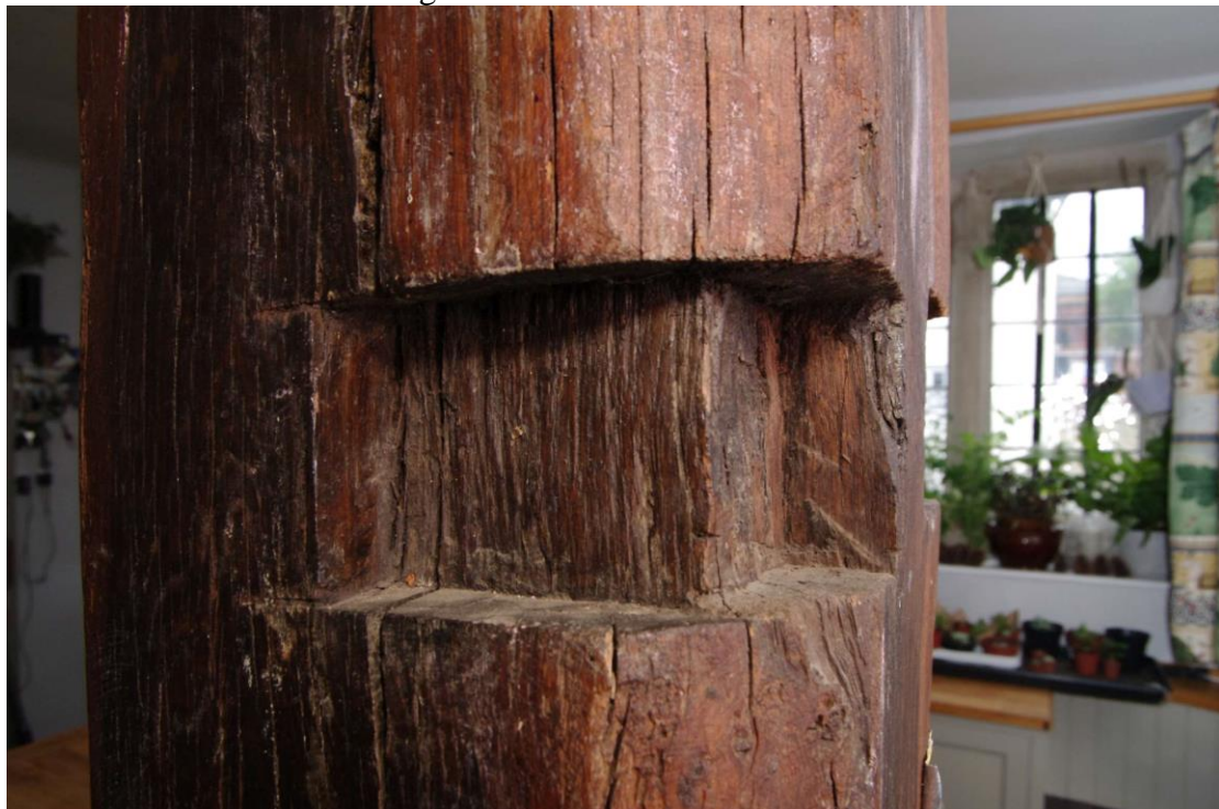
Figure 26 Timber post in kitchen socket detail
