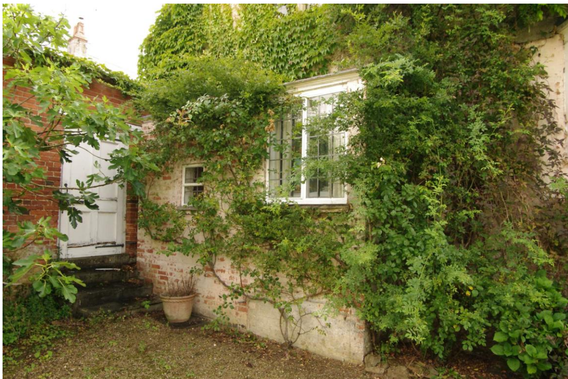
Figure 16 Single storey extension Looking north-east. The wall on the left is the boundary wall to Churchgate. The small window lights the inside toilet
