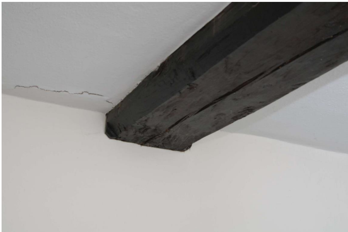
Figure 30 First floor landing, stop-chamfered beam end
