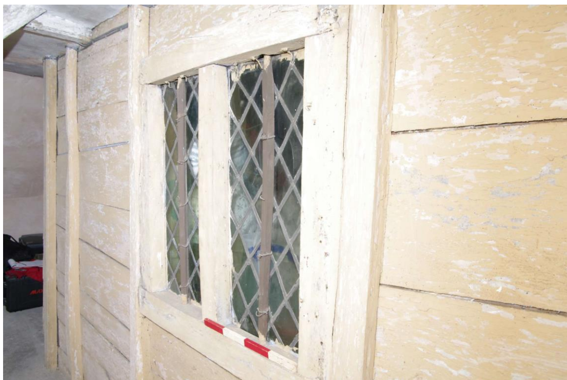
Figure 39 Leaded window in partition wall Looking south-east. 0.4m scale
