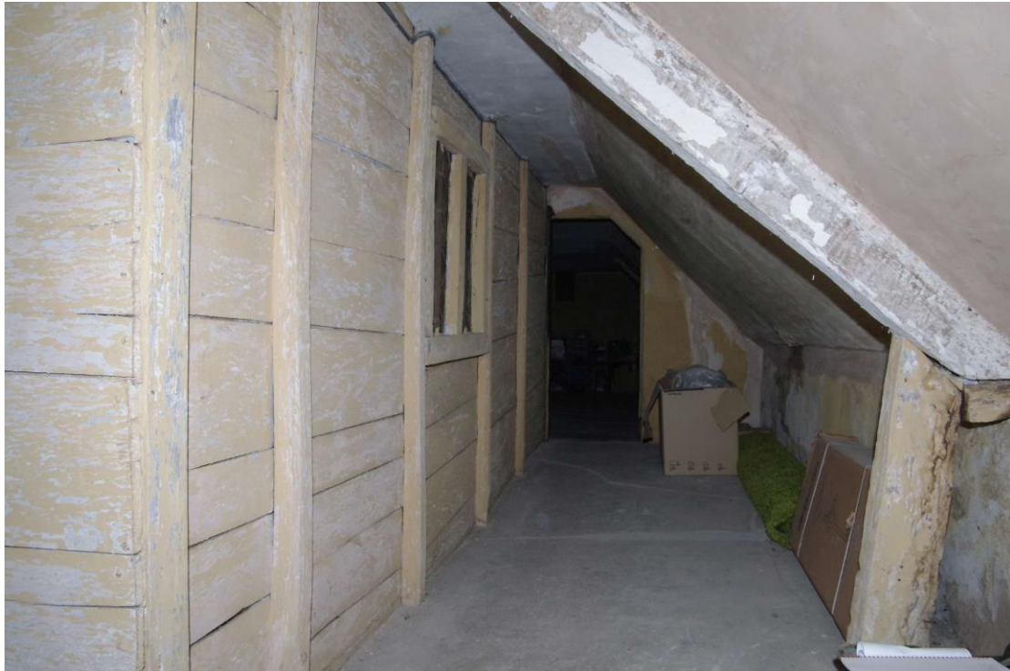
Figure 35 Second floor corridor
