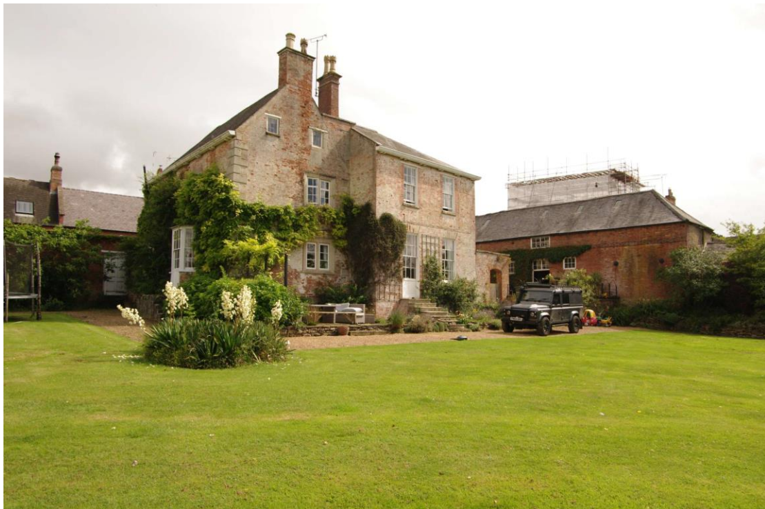
Figure 6 Rear view of Hallaton Grange Looking north-east. 1691 phase on left, the infilled 18th century addition is in the centre of the picture
