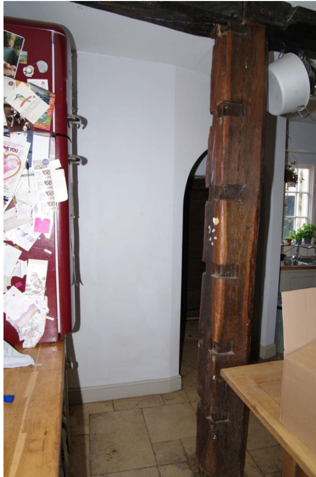
Figure 25 Ground floor, kitchen. Timber post Looking south towards inserted toilet wall
