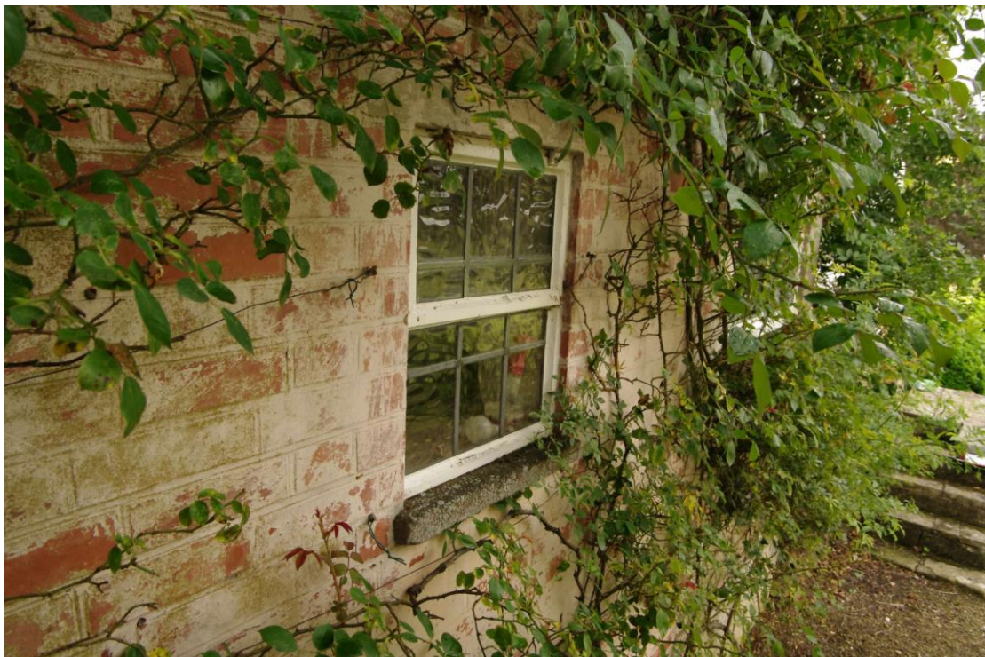
Figure 18 Single storey extension window detail Looking south-east. Note hard-fired bricks
