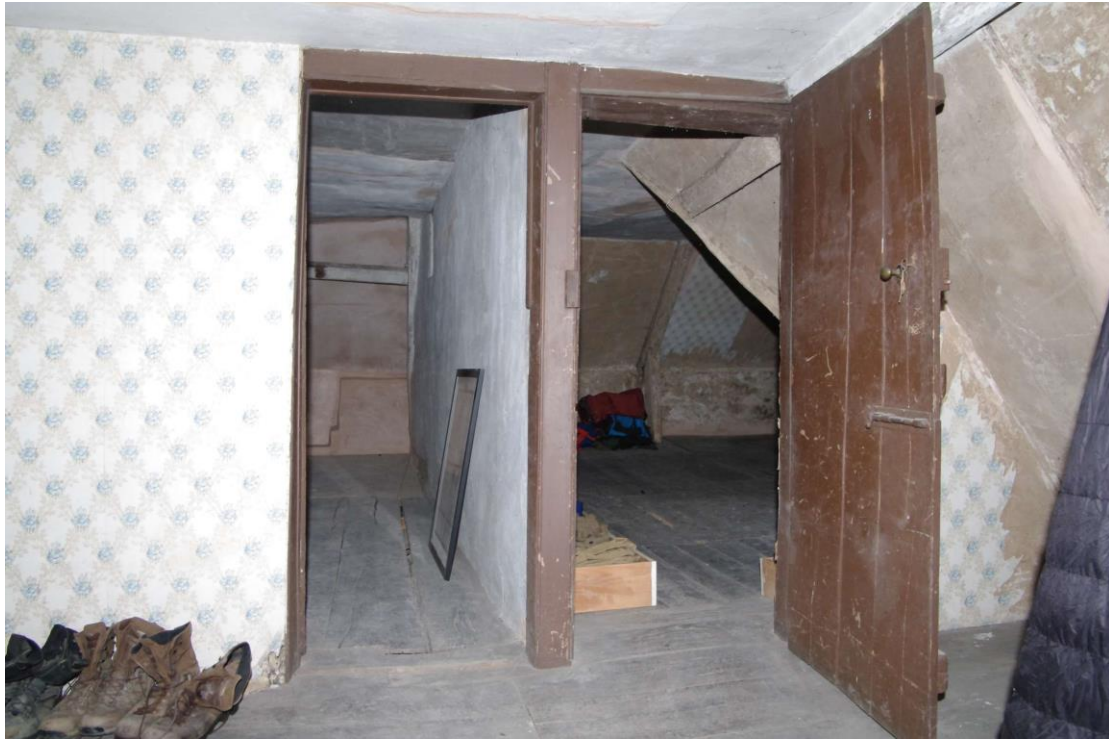
Figure 43 Second floor. Landing to former stairs Looking north from rear bedroom. Former landing on left. Middle room on right. The door on the right is that shown in Figure 42
