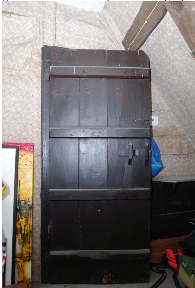
Figure 38 Second floor. Door detail in south-eastern boarded room Looking east. Note wooden sliding lock
