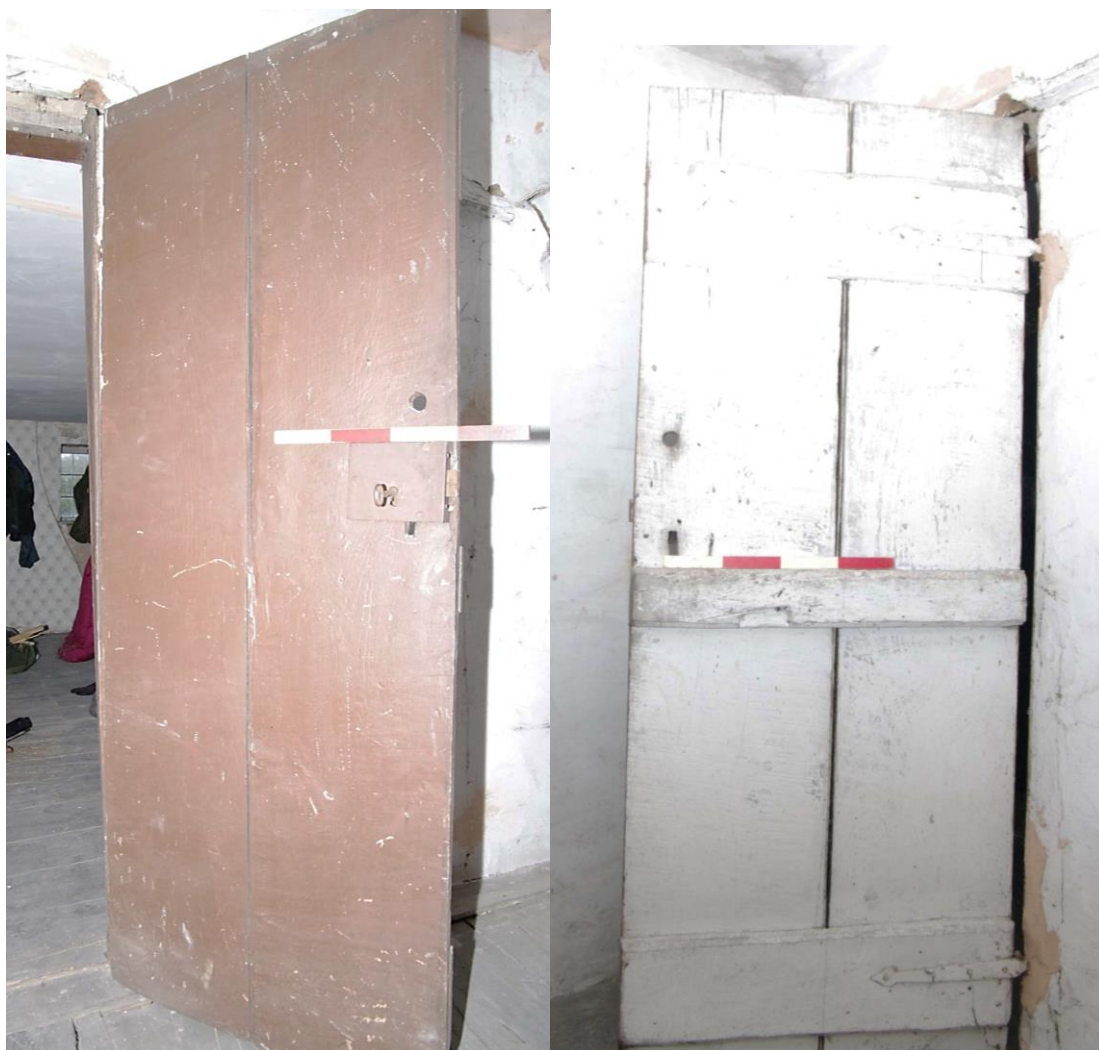
Figure 45 Door from former landing to rear room detail 0.4m scale. Note wooden lock plate still with key
