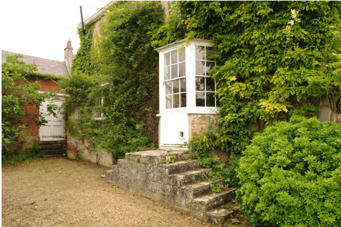
Figure 17 Single storey extension and adjacent steps Looking north-east.
