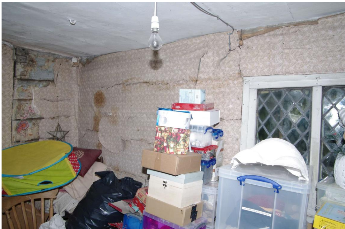
Figure 36 Second floor, inside the partitioned room
