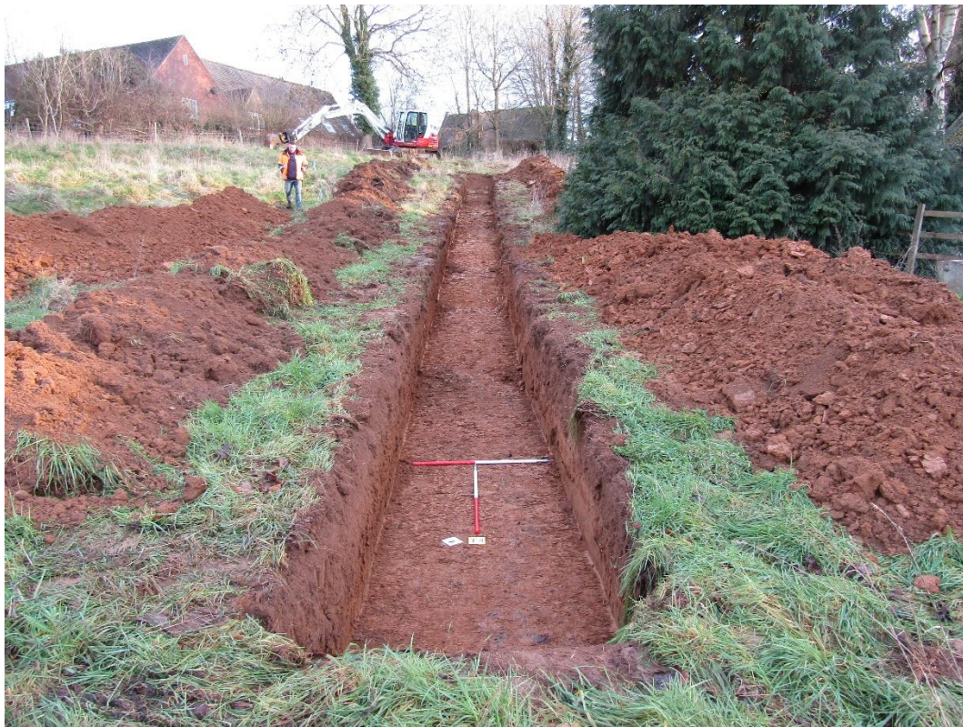
Figure 8: Trench 4. Looking south.
