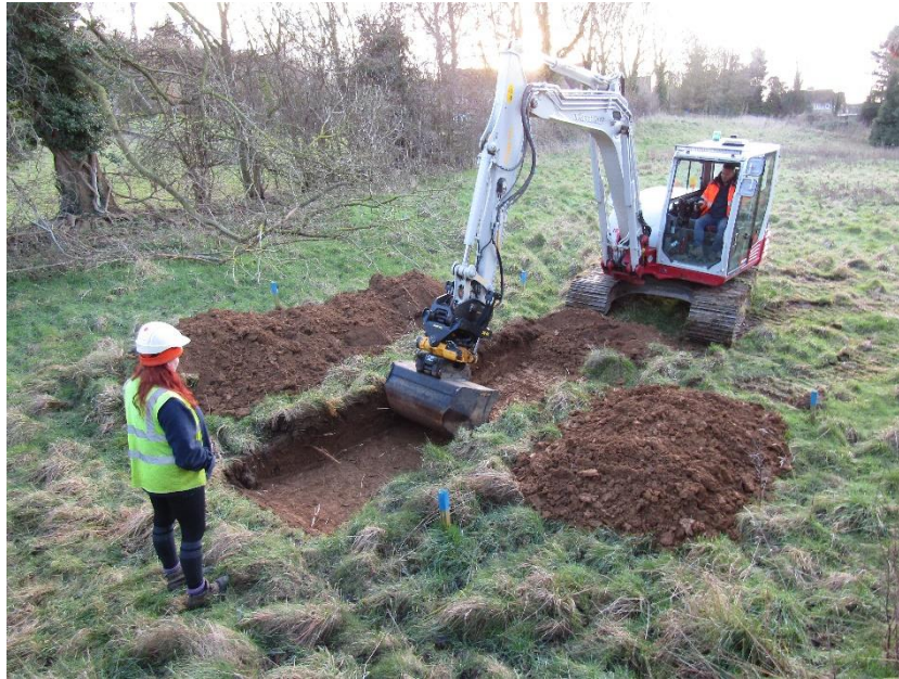
Figure 4: Work in progress.
