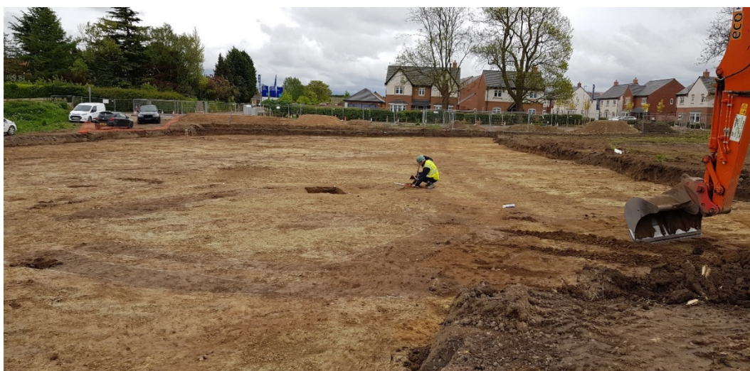
Figure 17: Machining of Enclosure 1: view south
