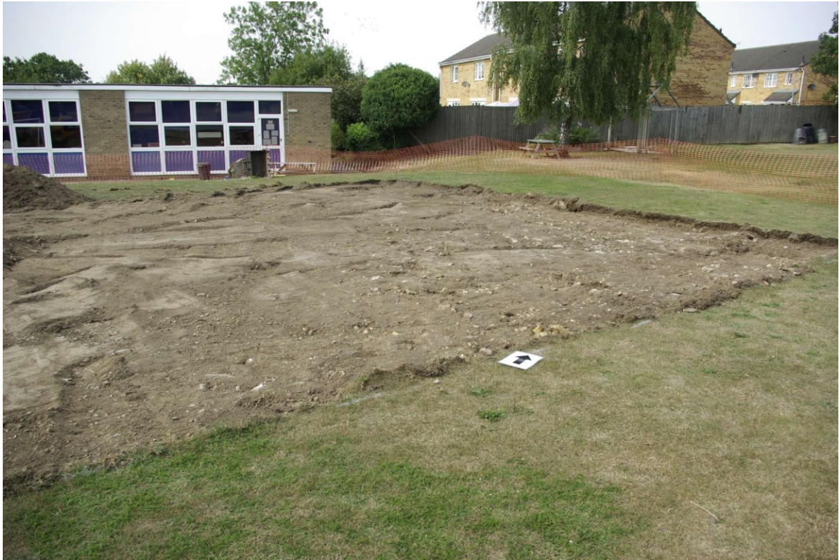
Figure 9 North end of games area at maximum depth of excavation
