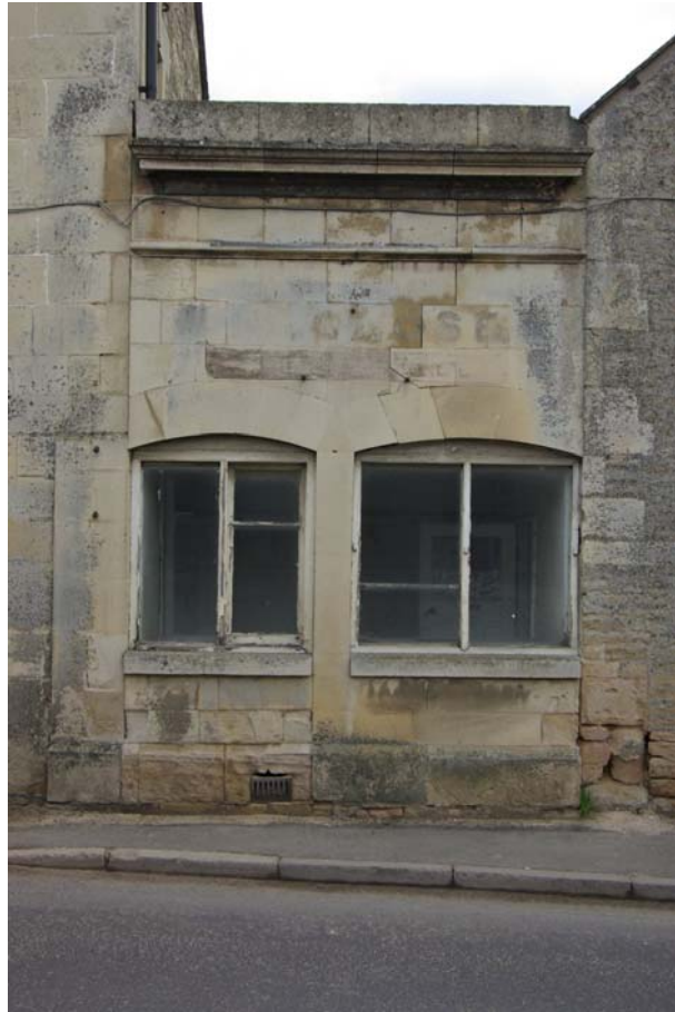
Figure 4 Principal Elevation of Passage Room Between 47 & 49 (Looking South).
