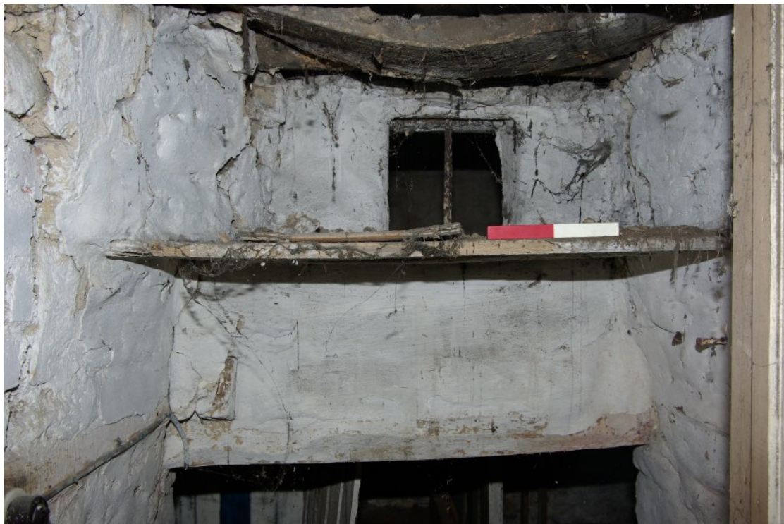
Figure 15 Arrow Slit Opening Above Cellar Access, No 49.
