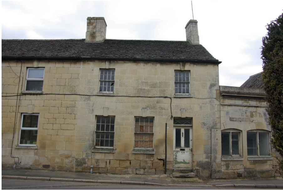
Figure 2 Number 47, Principal Elevation (Looking South).
