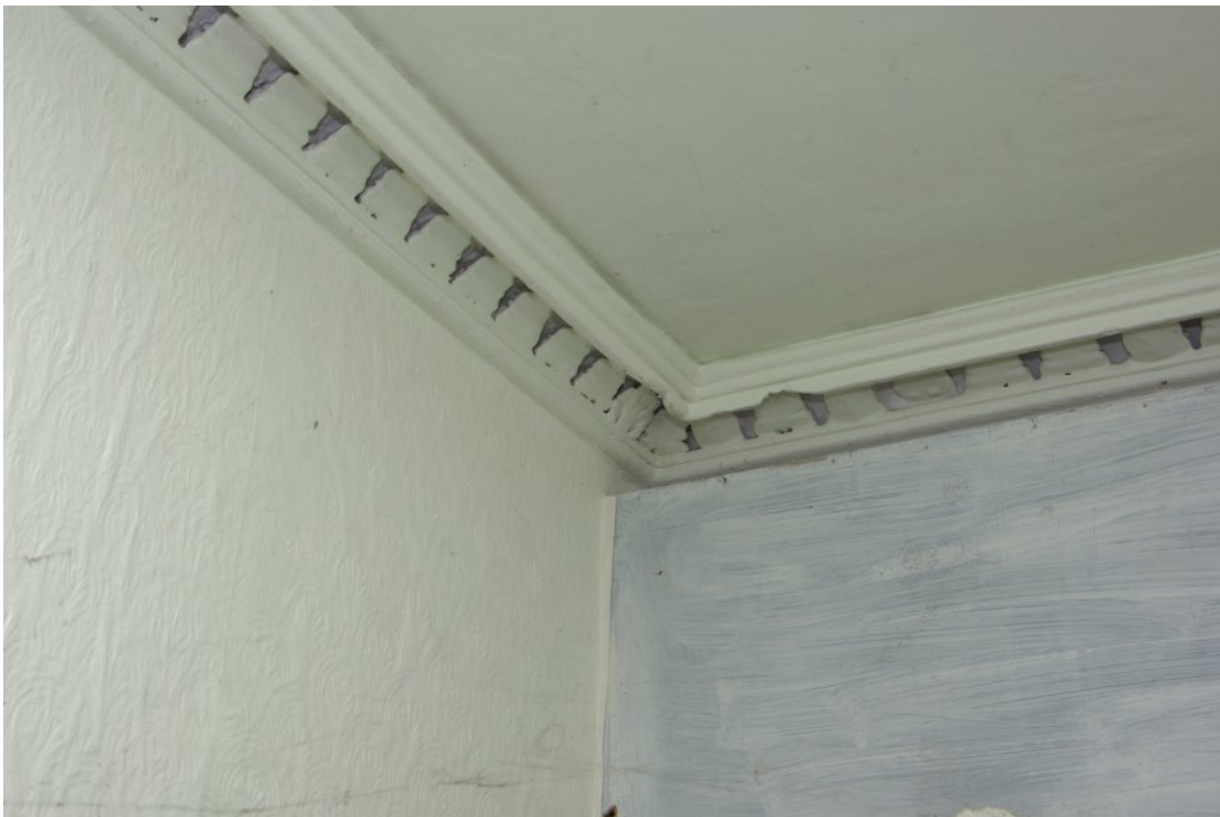
Figure 11 Outer Hallway Cornice, No 47.
