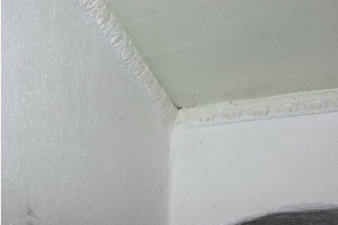
Figure 10 Hallway Cornice, No 47.
