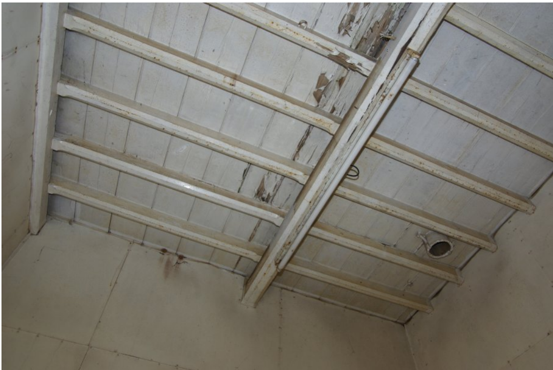
Figure 13 Roof Structure of Passage Room, No 47 & 49.
