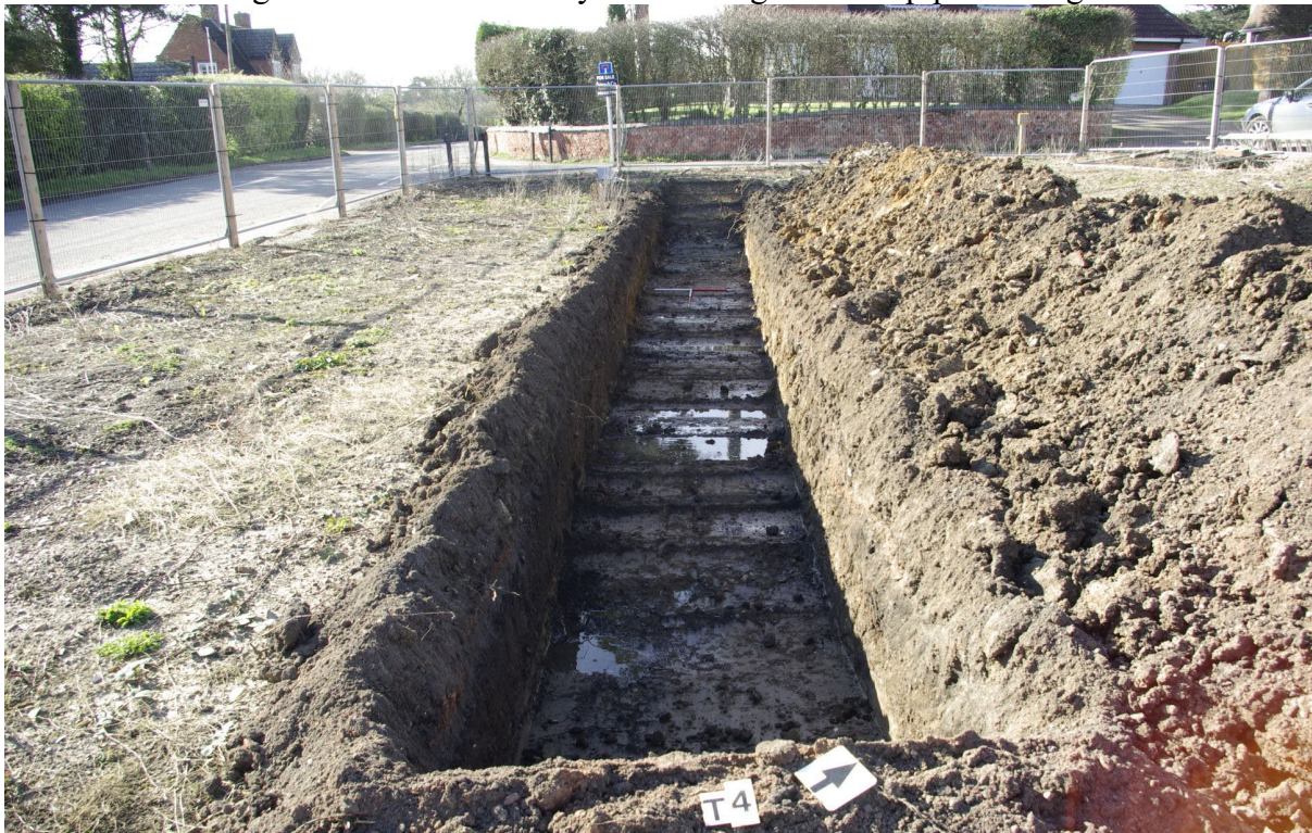
Figure 16 Trench 04 Looking west. 1m scales. Ashby Road on left, Church Lane at far end of trench
