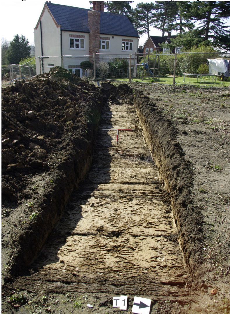
Figure 9 Trench 01 Looking south-west. 1m scales. Land drain running across the trench this side of scales
