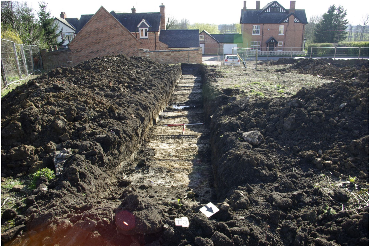
Figure 13 Trench 03 Looking south. 1m scales. Heavily disturbed area just beyond the scales
