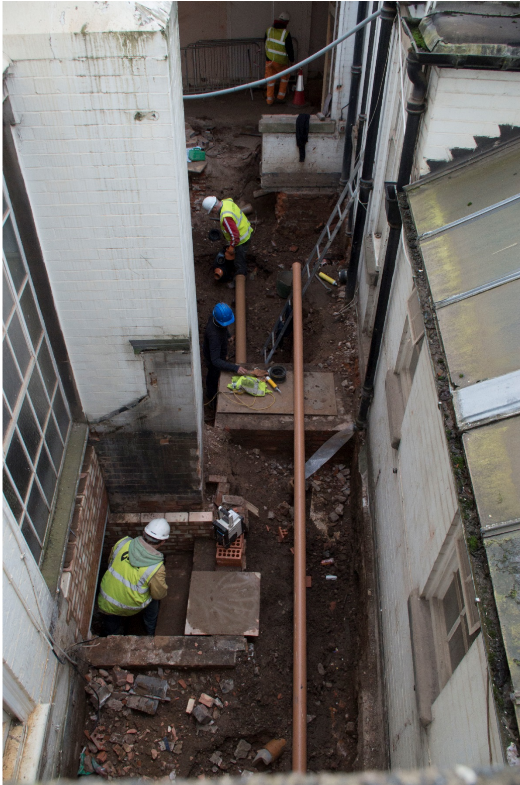
Figure 7: Hand excavation of courtyard
