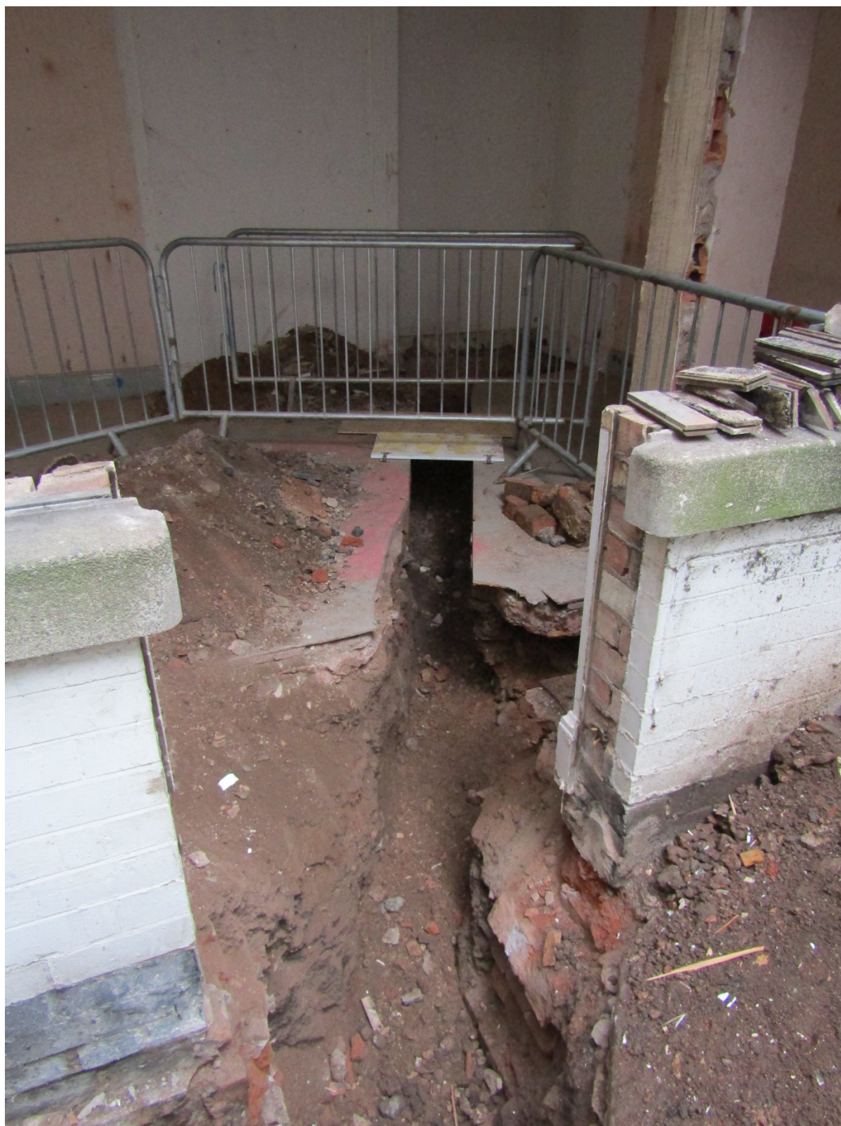
Figure 10: Trench for proposed additional services
