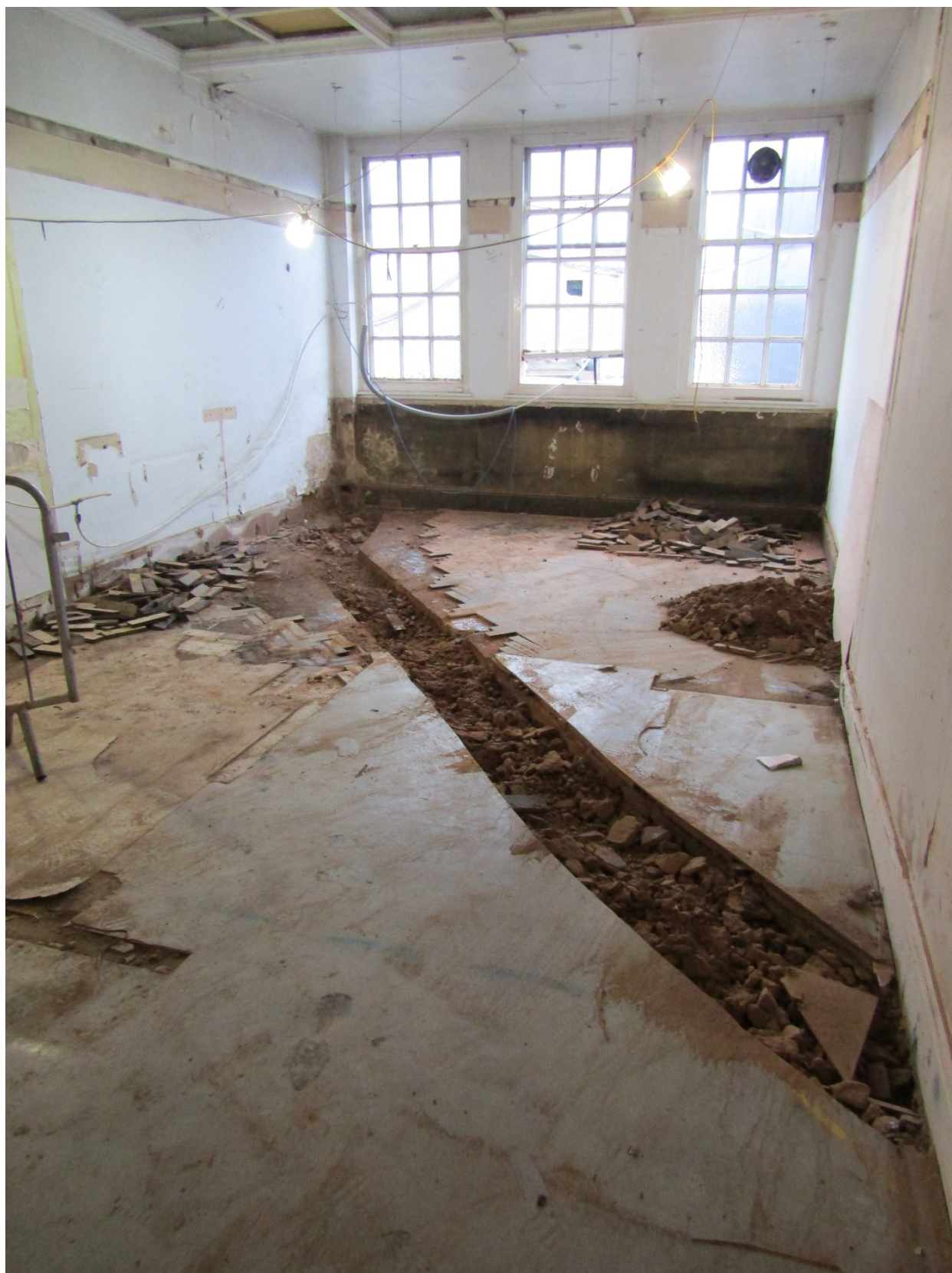
Figure 9: Trench for proposed additional services
