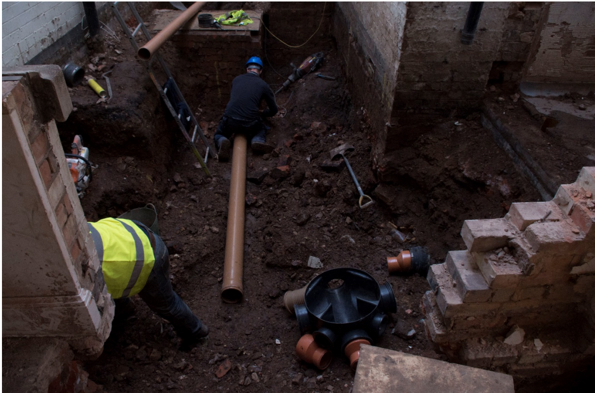
Figure 8: Hand excavation within courtyard
