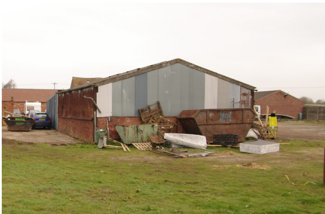
Figure 49 South and west facing elevations of Barn 4 Looking north-east
