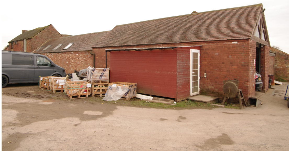
Figure 14 Western end of north facing Barn 2 range Looking south-east. The roof is new as is some of the brickwork
