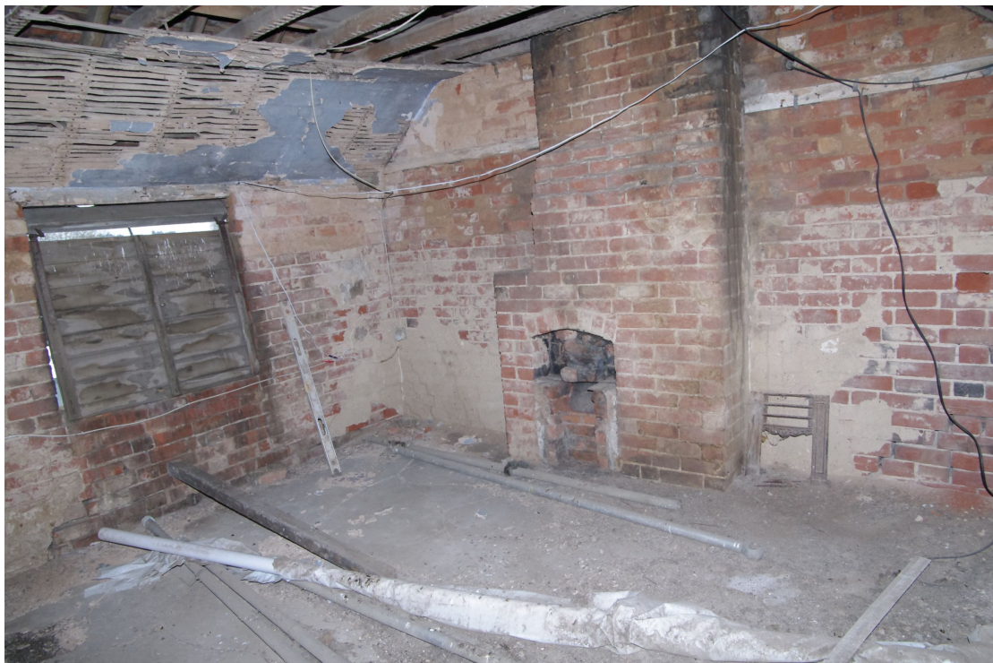
Figure 28 First floor room of former house Looking north-east. Note presence of ceiling and plaster floor
