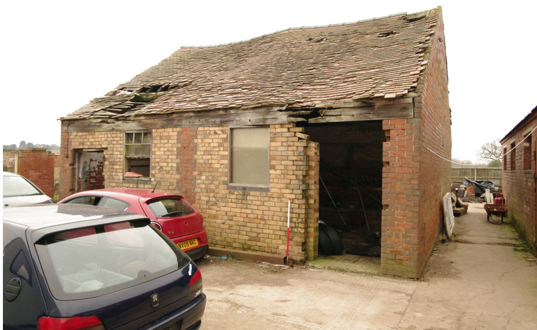
Figure 40 Barn 3 range, former double-sided cart shed Looking south-west
