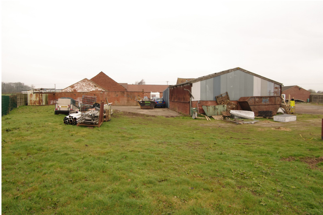
Figure 9 Saltersford Farm seen from the south Looking north
