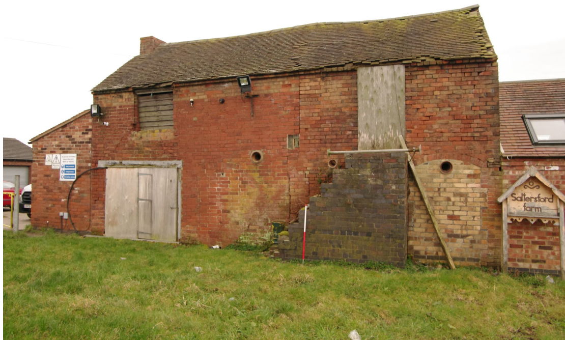
Figure 12 North facing elevation of two storey former house and hayloft Looking south-east. The buff-coloured bricks blocking the door to the right can be seen elsewhere on the farm
