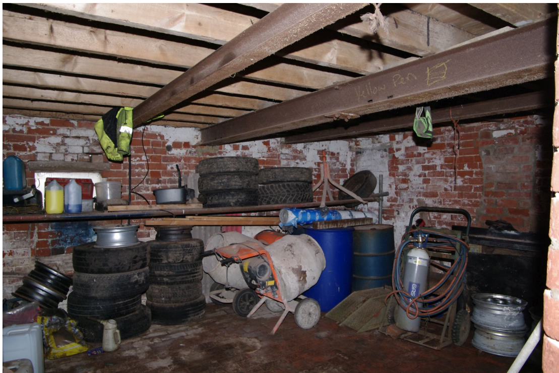
Figure 32 Ground floor room at southern end of Barn 1 range Looking south-east
