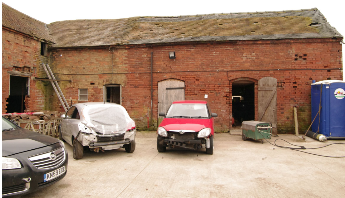
Figure 21 West facing elevation of Barn 1 range Looking east. 1m scale
