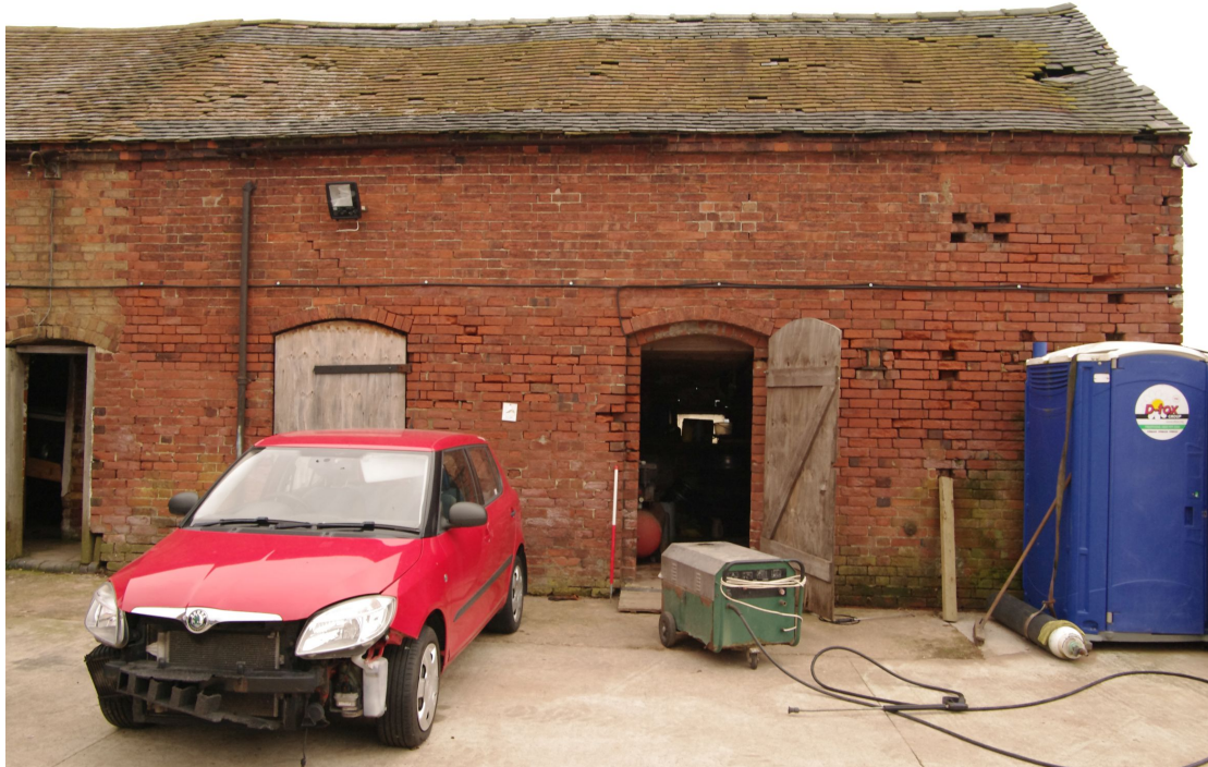
Figure 23 Southern end of west facing elevation of Barn 1 range Looking east. 1m scale
