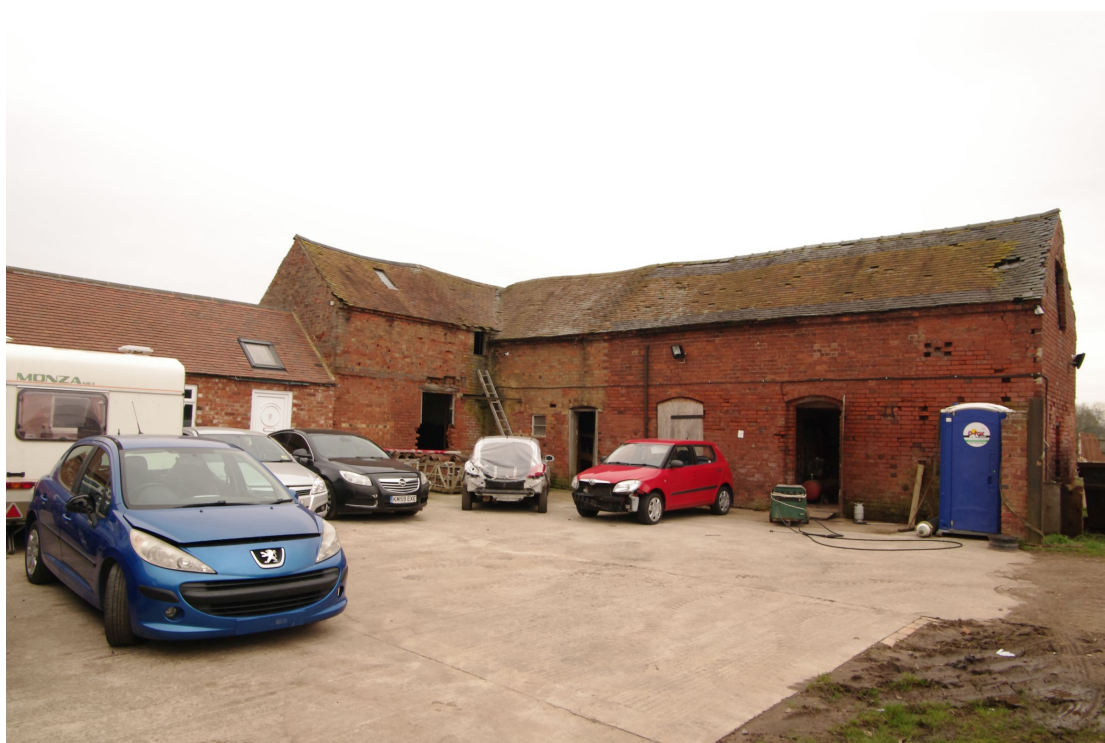
Figure 18 South and west facing elevations of Barn 1 Looking north-east. Barn 2 range on left
