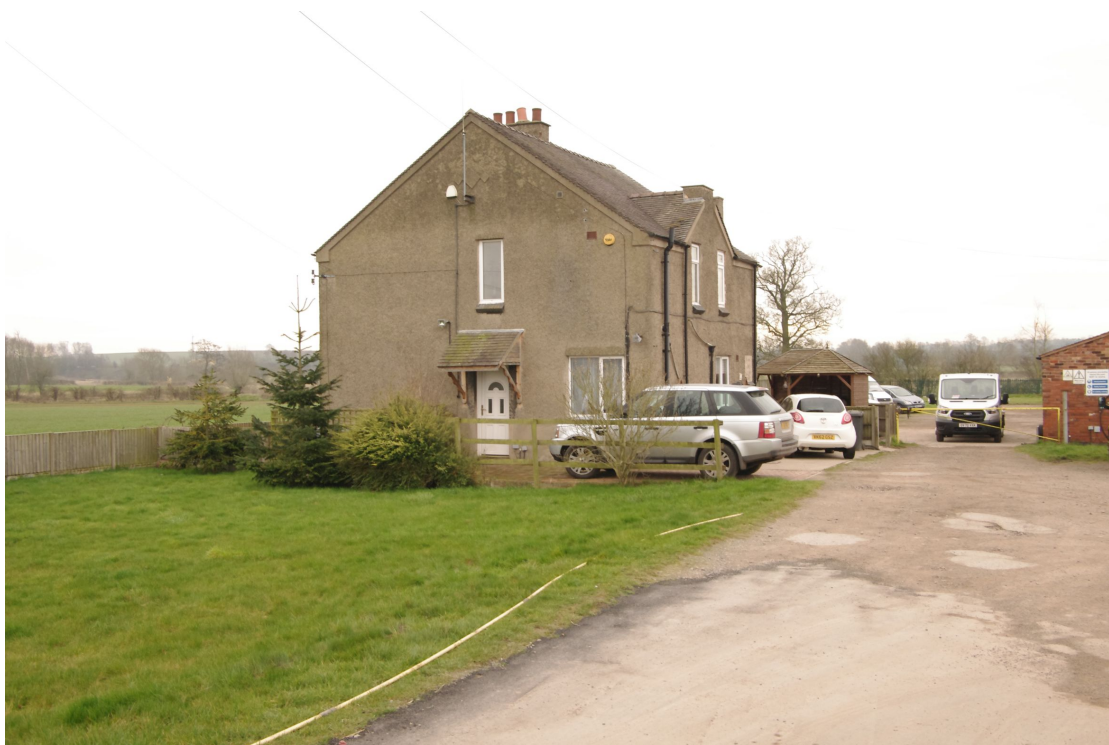
Figure 10 Saltersford farmhouse Looking south-east. This 1920s building is not part of the proposed redevelopment scheme
