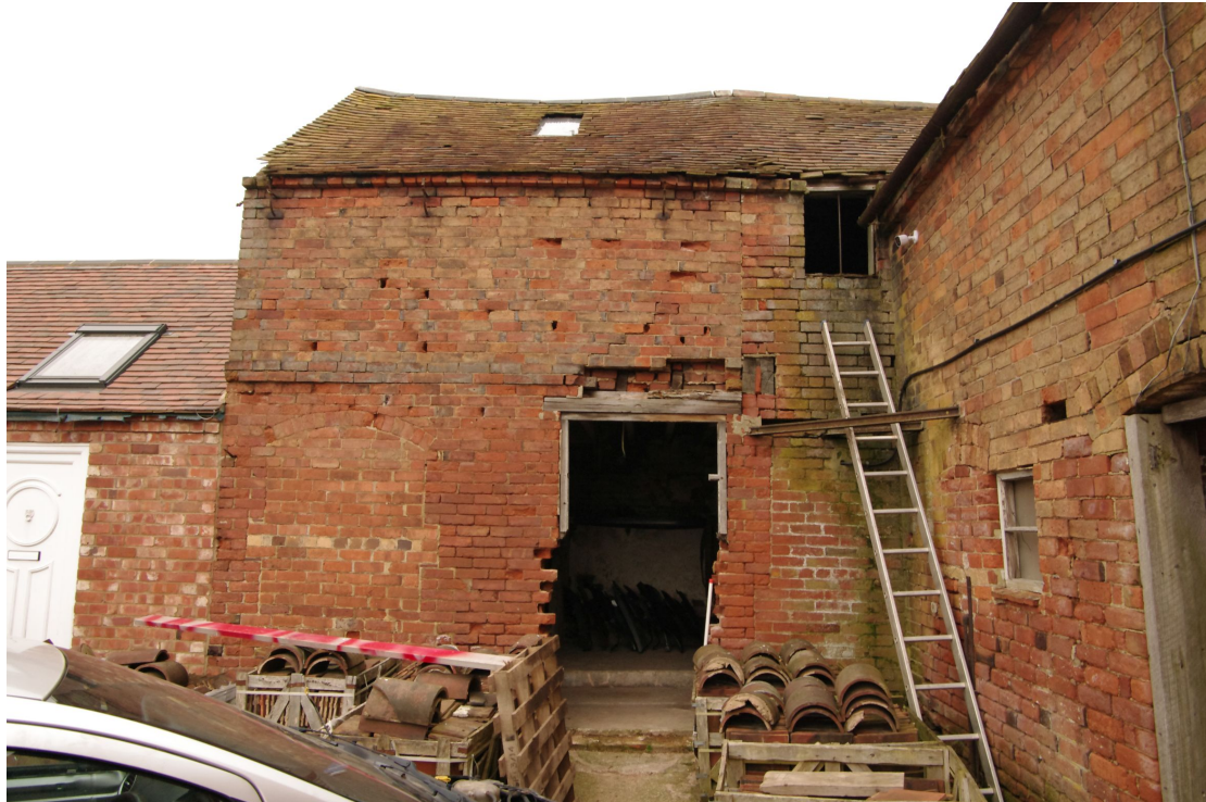
Figure 19 South facing elevation of hayloft Looking north. Note the brick joint to the right of the doorway
