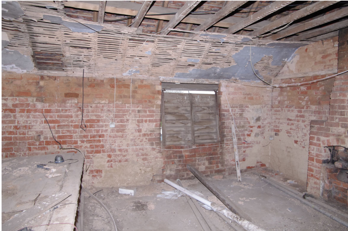
Figure 29 First floor room of former house Looking north. Note change in bricks indication raised wall height
