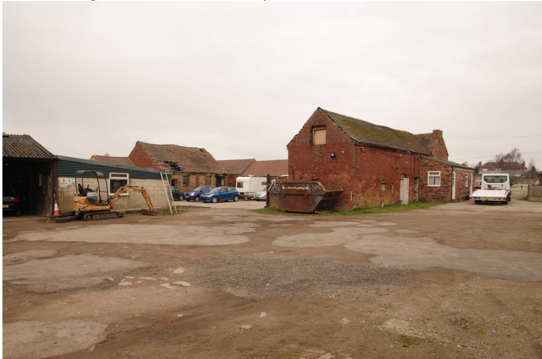
Figure 8 Saltersford Farm seen from the south-east Looking north-west towards the yard. Barn 4 on far left
