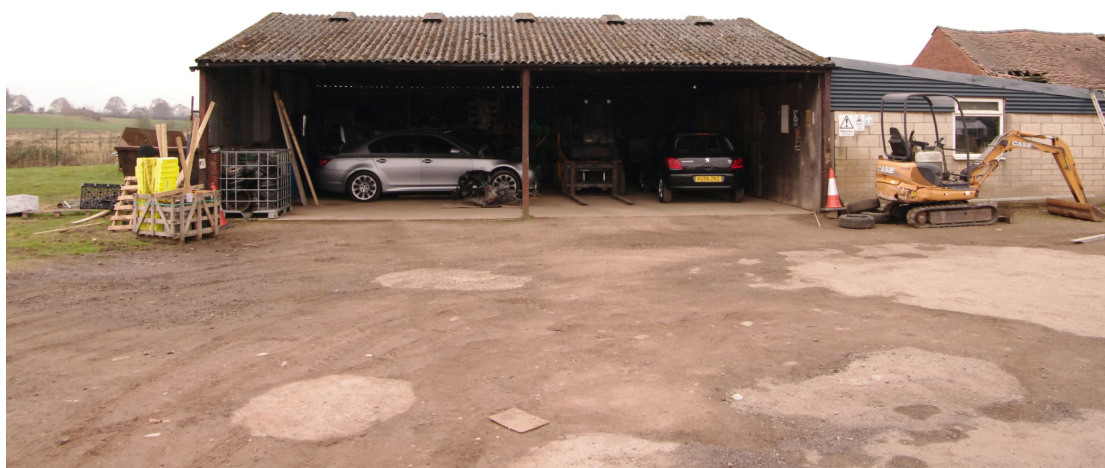
Figure 48 Metal-clad and framed Barn 4 Looking west
