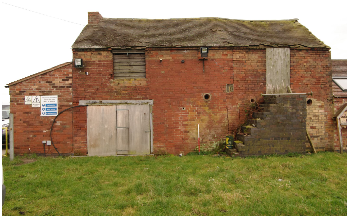
Figure 11 North facing elevation of two storey former house Looking south. 1m scale. Note the extension to the right and raised eaves. There is a blocked ground floor window to the left of the scale. Lean-to extension on left is relatively modern
