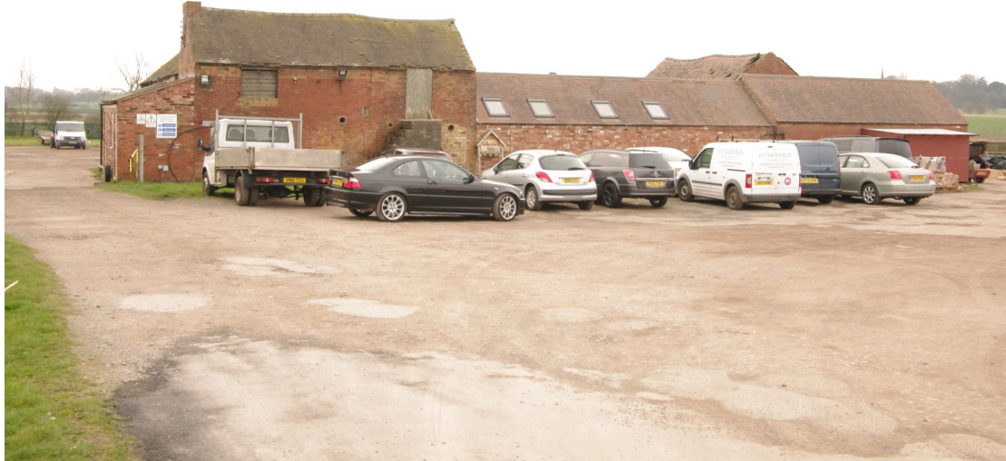
Figure 7 Saltersford Farm seen from the north Looking south-west. The two storey barn on the left is the oldest element
