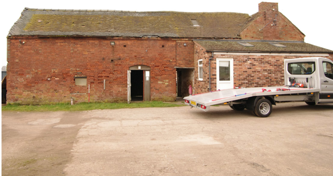
Figure 25 East facing elevation of Barn 1 range Looking west. 1m scale. The lean-to structure on the right is relatively modern
