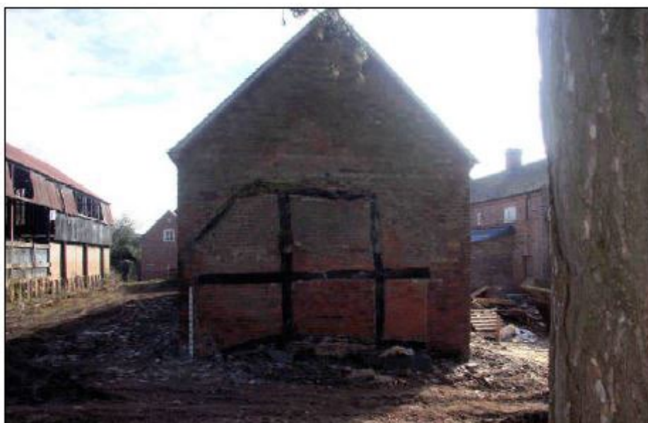
Figure 4: Home Farm renovations in 2010, looking east, Dutch barn to north (Bradwell 2010).
