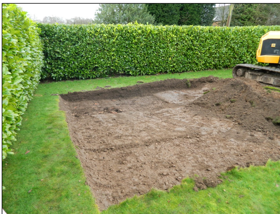
Figure 8: Southern end of pool house excavation, looking east.
