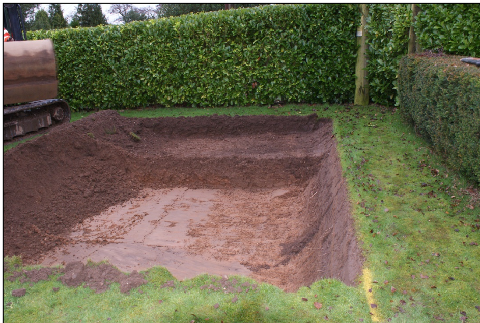
Figure 7: Northern end of pool house excavation, looking east.
