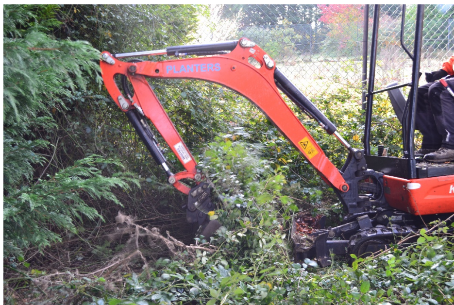
Figure 4: Trench 1, cleaning plant growth prior to digging. Looking south.
