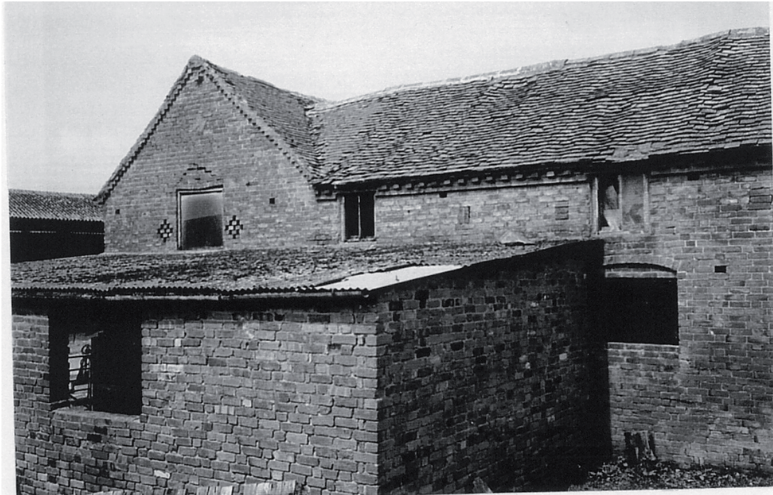
Plate 5 Lean-to II, adjacent to southwest corner of south range and south gable of west range. Also shows diamond ventilator panels and stepped brickwork of the south gable.
