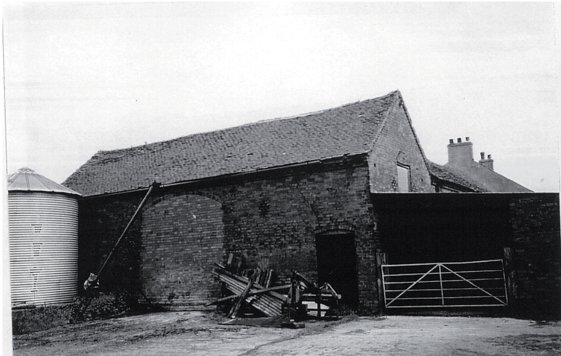
Plate 5 Lean-to II, adjacent to southwest corner of south range and south gable of west range. Also shows diamond ventilator panels and stepped brickwork of the south gable.
