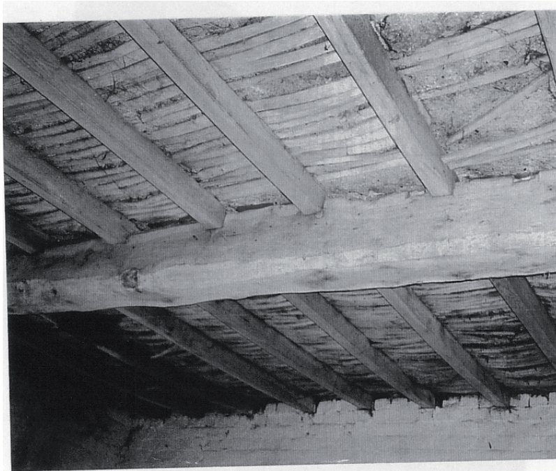
Plate 2 Underside of lath and lime-ash plaster floor to upper storey. South range.
