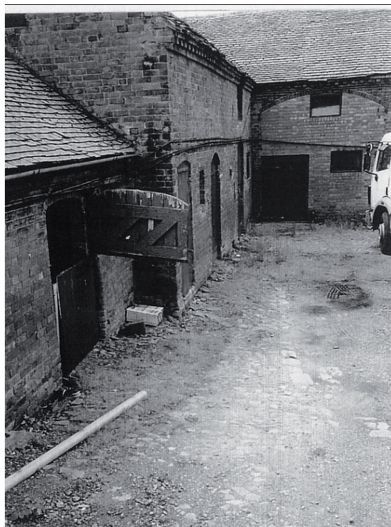
Plate 1 South range (left) showing trap pony stable door, other doors and window in range and decorative eaves work. Also shows West range (ahead) with original wagon entrance door, now blocked and later doors and windows.
