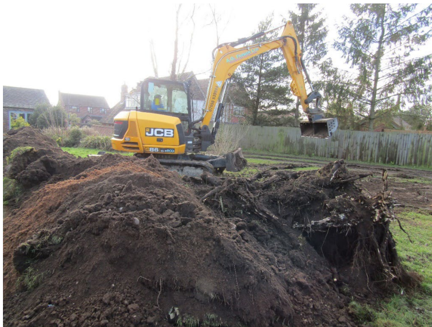
Figure 6: Work in progress.
