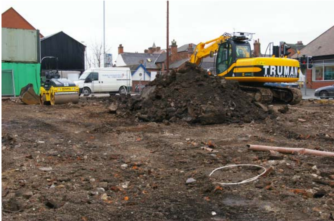
Plate 1: Work in progress, looking south-west
