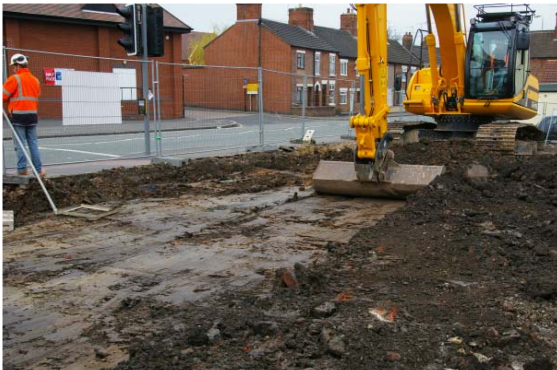
Plate 2: Stripping on south west corner, looking north-west
