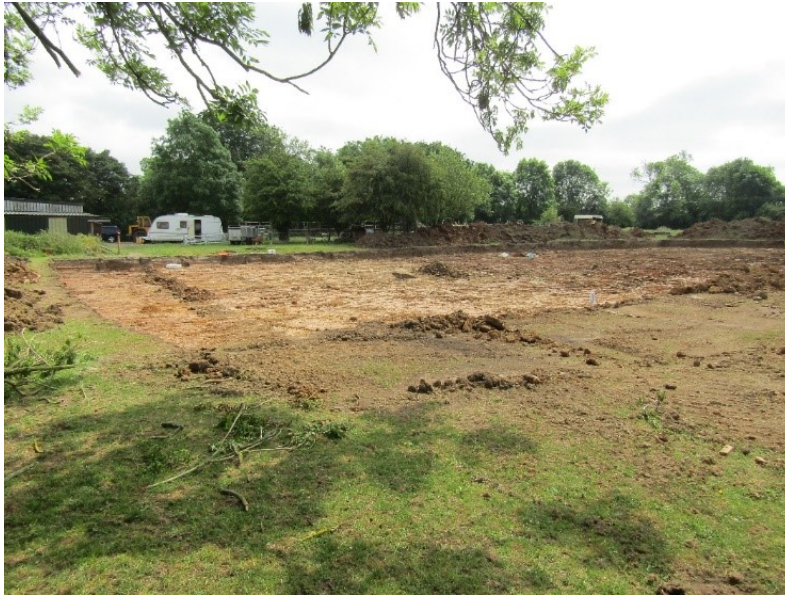
Figure 6: Work in progress, looking south-east.
