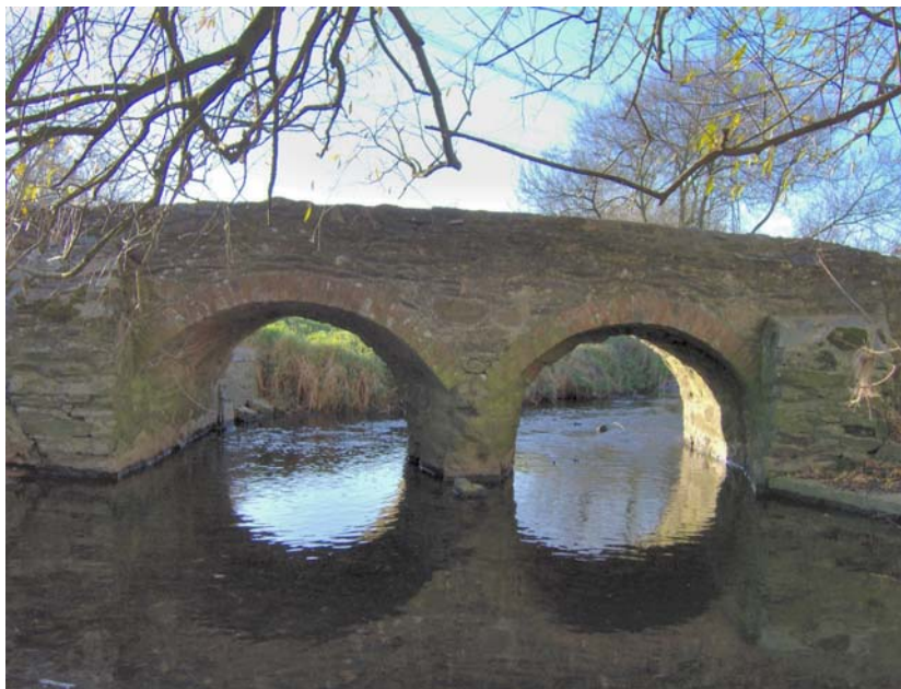
Figure 6 North Facing Parapet.
