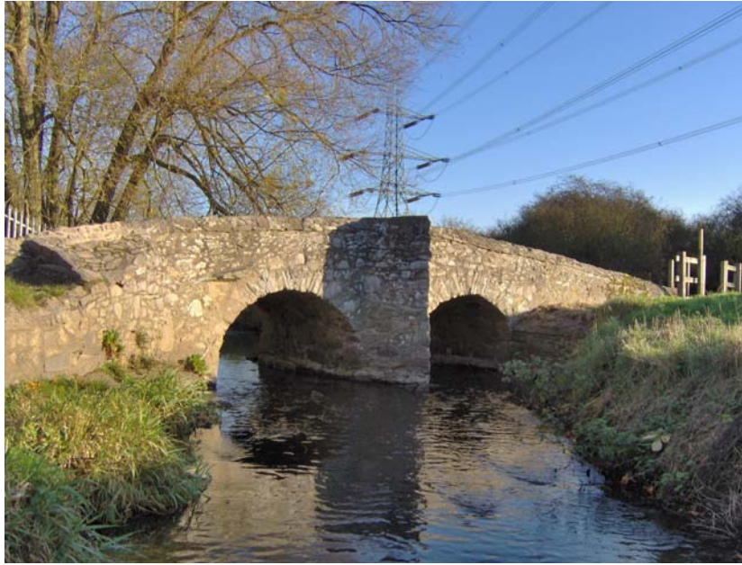
Figure 5 South- Facing Parapet.
