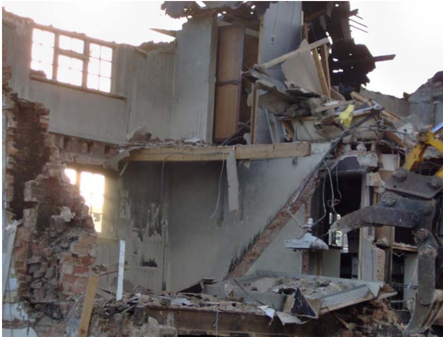
Colour Plate 4 Demolition in Progress.
