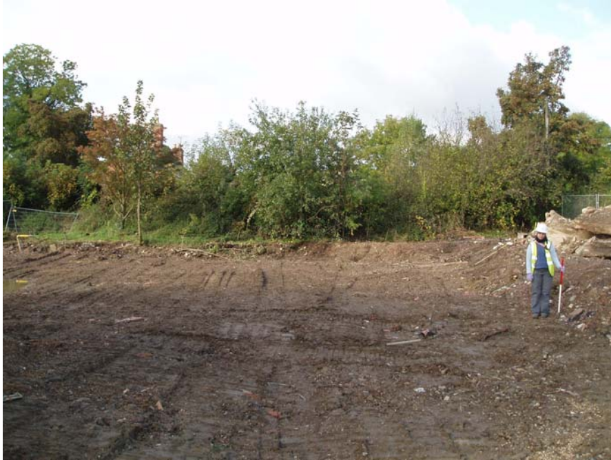
Colour Plate 3 Extent of Ground Reduction.
