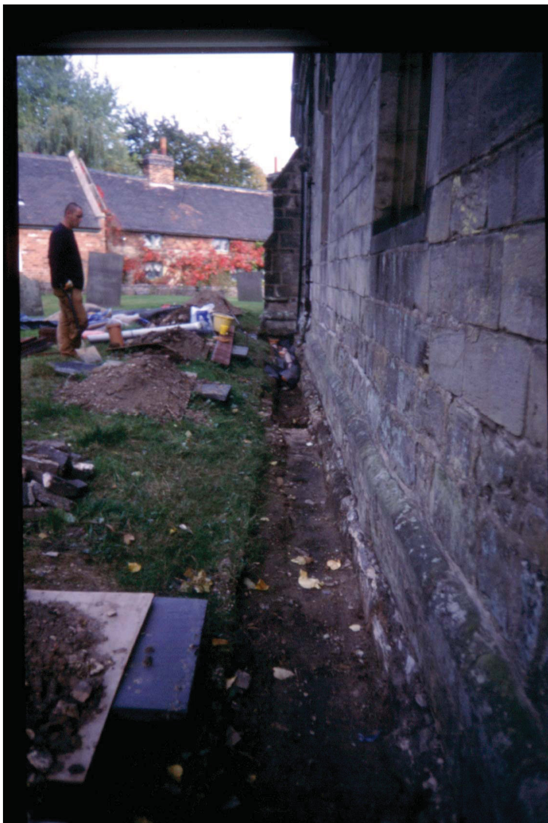
Illus. 5 Drainage works along the north wall of St James Church, Sutton Cheney viewed from the west
