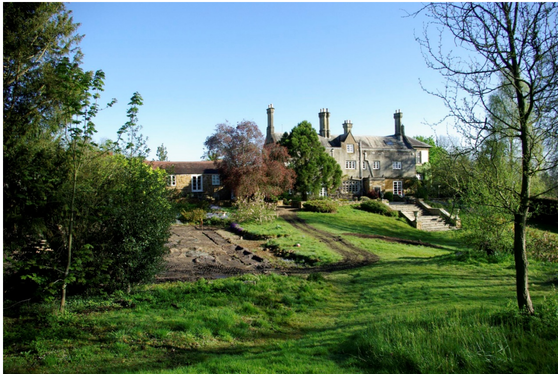
Figure 5: The Old Hall and pool site Looking north. The pool is to be located in the stripped area lower left
