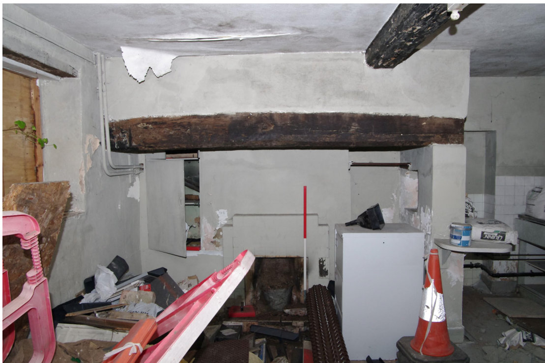
Figure 33 Room G1 fireplace Looking north-west. Note the blocked possible former doorway to right of fireplace. 1m scale
