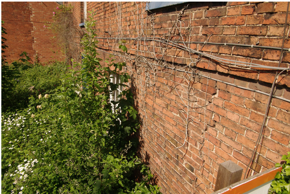
Figure 17 Decorative brick string course along south-east facing elevation Looking south-west
