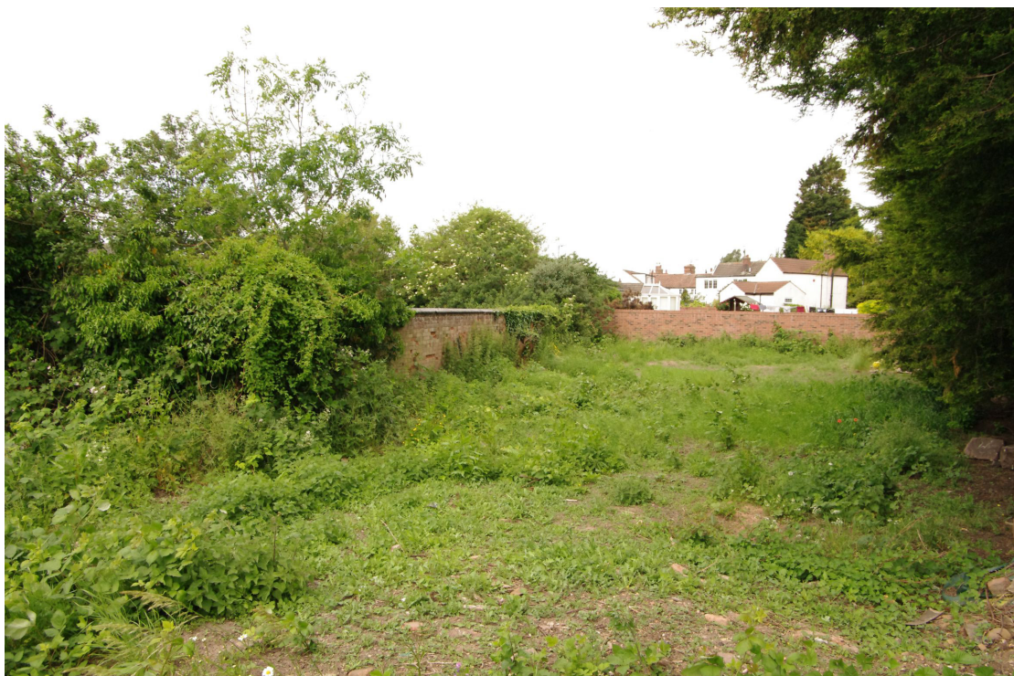
Figure 107 Boundary wall in north-eastern corner of site The wall is completely brick-built at this point. The eastern boundary alongside the railway is a modern steel fence
