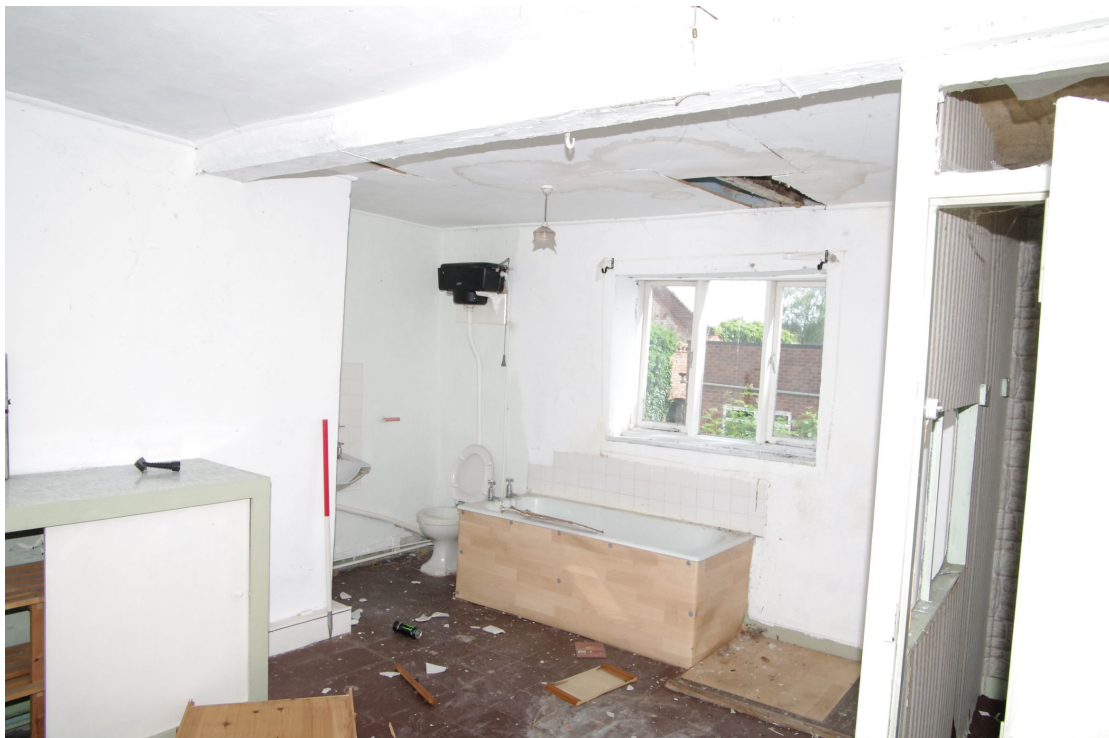
Figure 63 General view of Room F6 Looking north. The raised woodwork to the right of the bath show where the stairs came up from the ground floor. The stairs to the second floor were enclosed by the partition on the right. 1m scale
