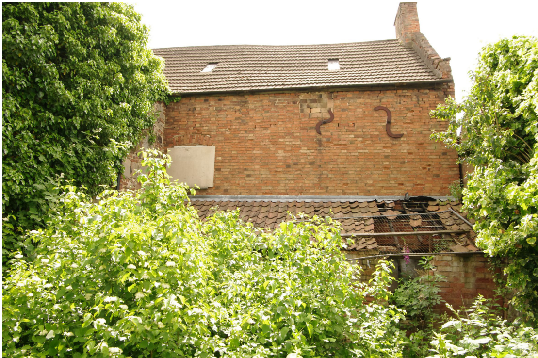
Figure 27 North-west facing elevation of 18th century range
