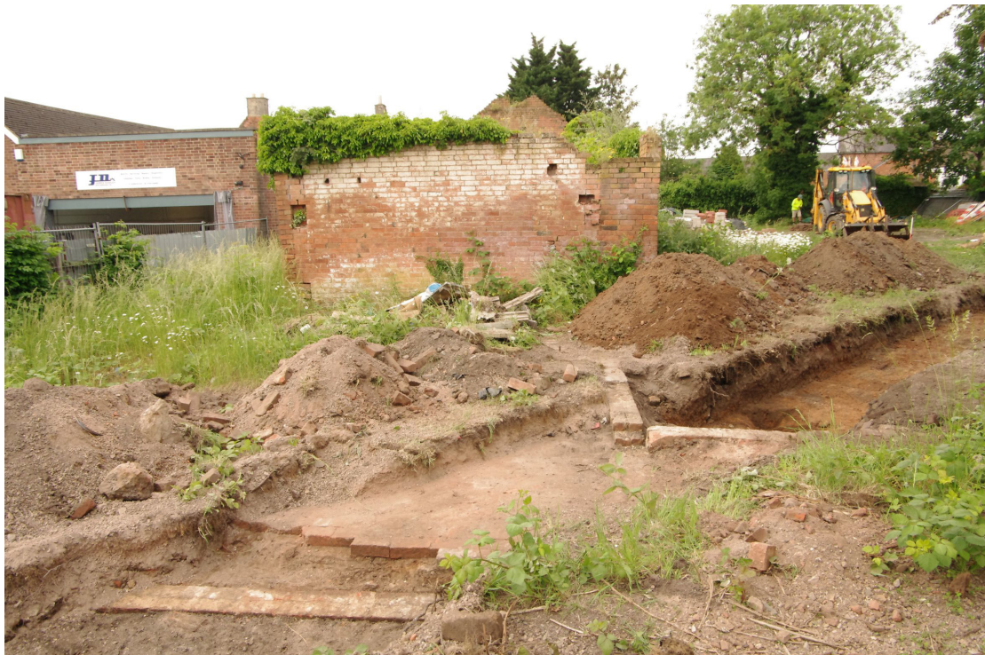
Figure 97 Barn 2, north-east facing elevation Looking south-west. The evaluation trench shows the foundations of the corner of the former courtyard ranges which can be seen in the foreground, as can the link to Barn 1 on the right
