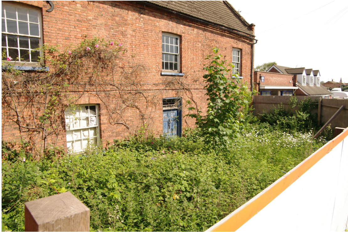
Figure 16 South-east facing elevation Looking north-east over hoardings
