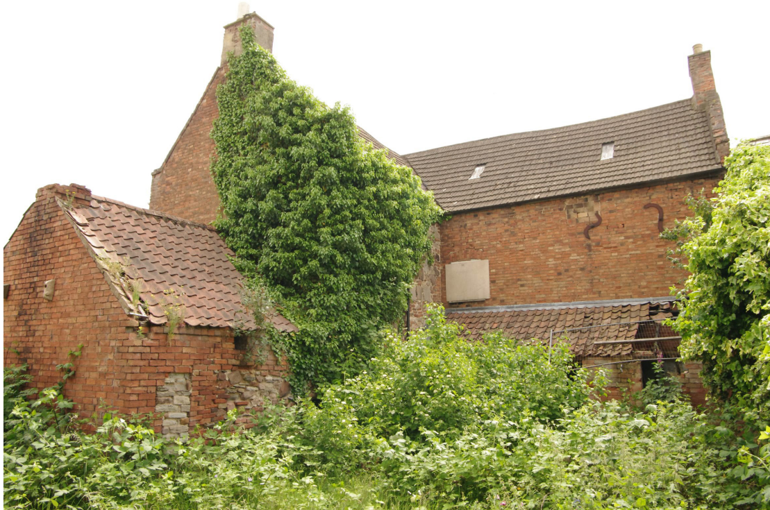
Figure 24 Rear of farmhouse looking south-east Note remnants of stone walling in the single storey building and the rear two-storey range (see Figs 25 and 26 below)
