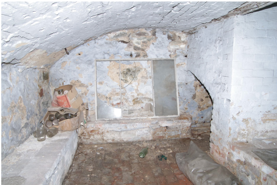
Figure 29 Cellar Looking north-east. Stone walls, brick vaulting, floors and thralls
