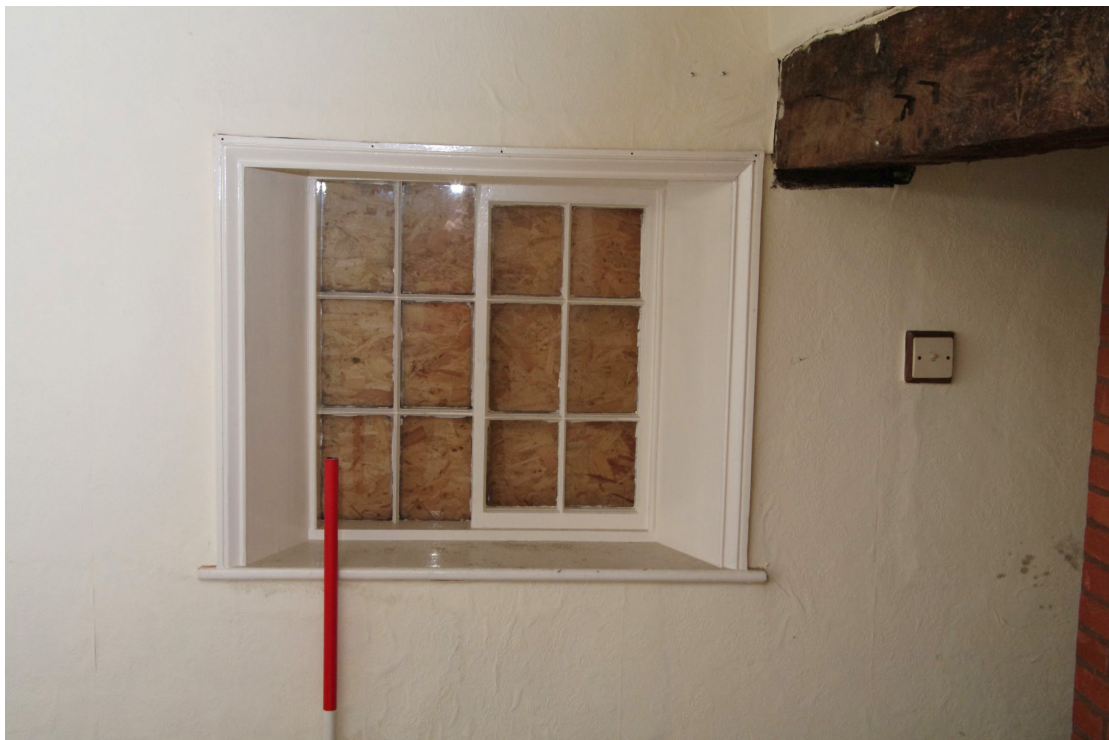
Figure 45 Window detail on north-west wall of Room G5 Horizontal sliding sash
