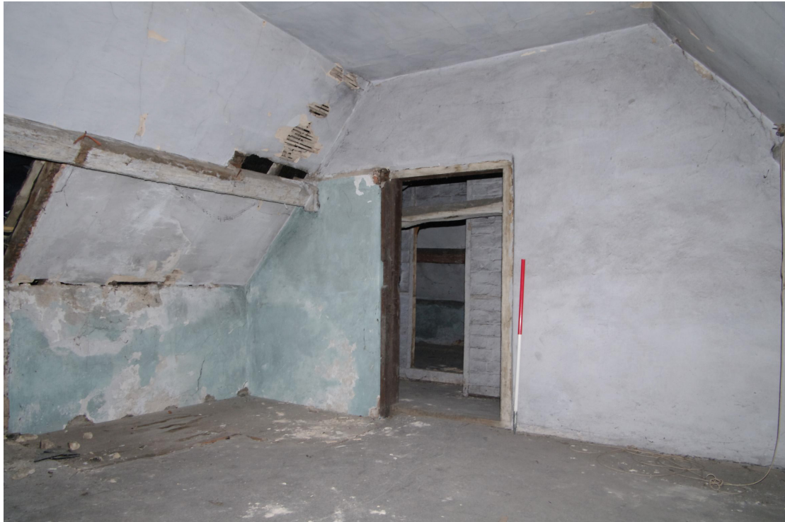
Figure 84 General view of Room S6
