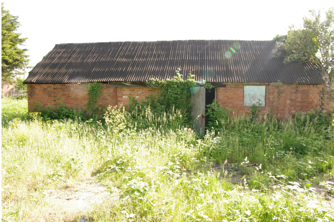
Figure 85 Barn 1, south-west facing elevation
