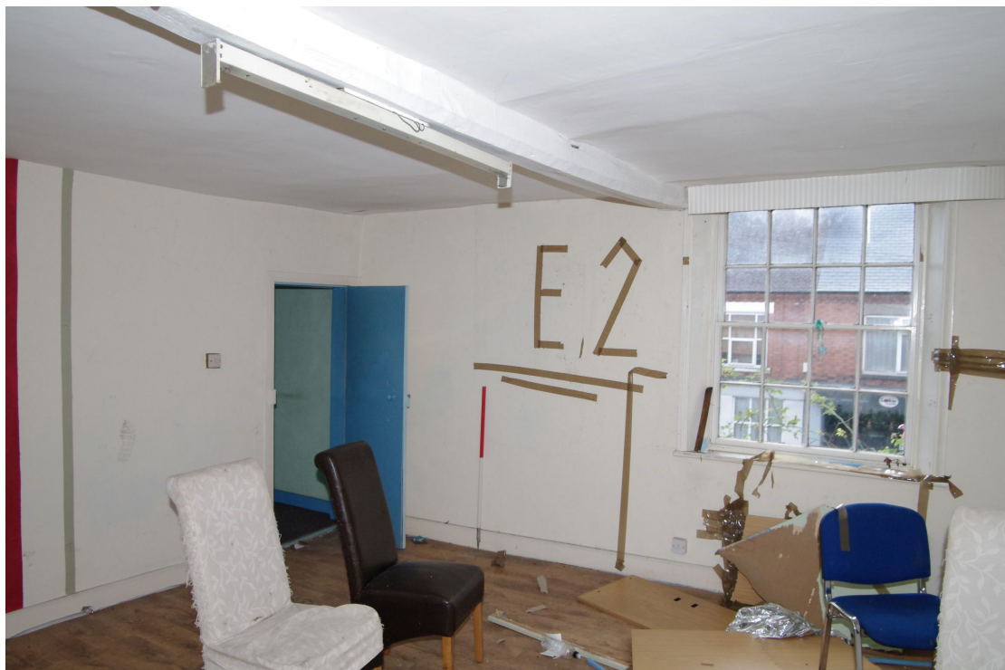
Figure 55 General view of Room F2 Looking south-east. A blocked window can be seen on the outside wall to the left of the 1m scale
