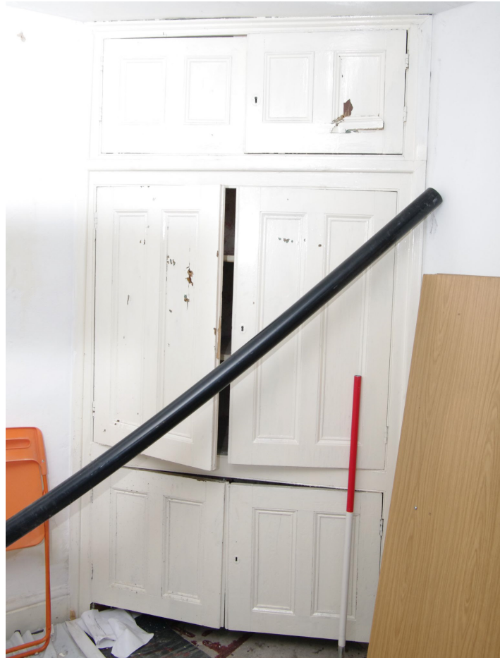
Figure 50 Corner cupboard detail Room G6 Looking north. 1m scale
