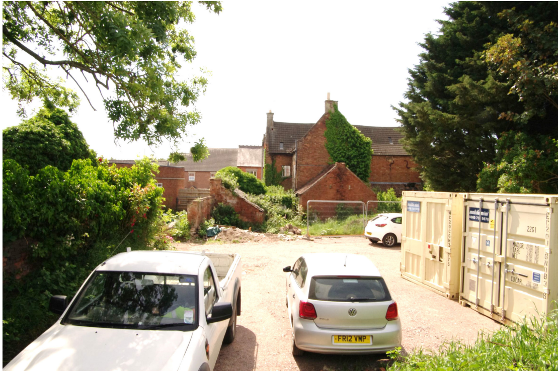
Figure 14 General view looking south-east Farmhouse on right, Outbuilding 1 centre left, ivy covered gable of Barn 2 on left
