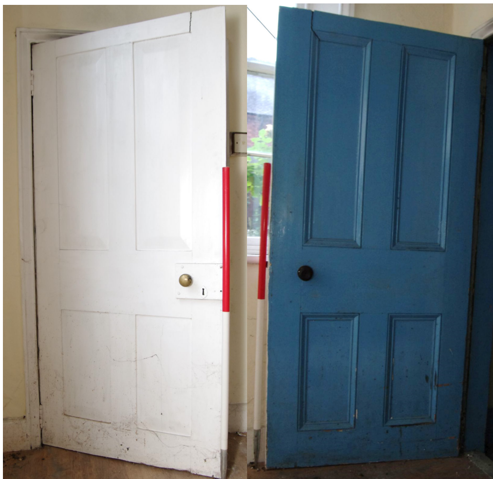
Figure 46 Room G5 door detail 1 metre scale
