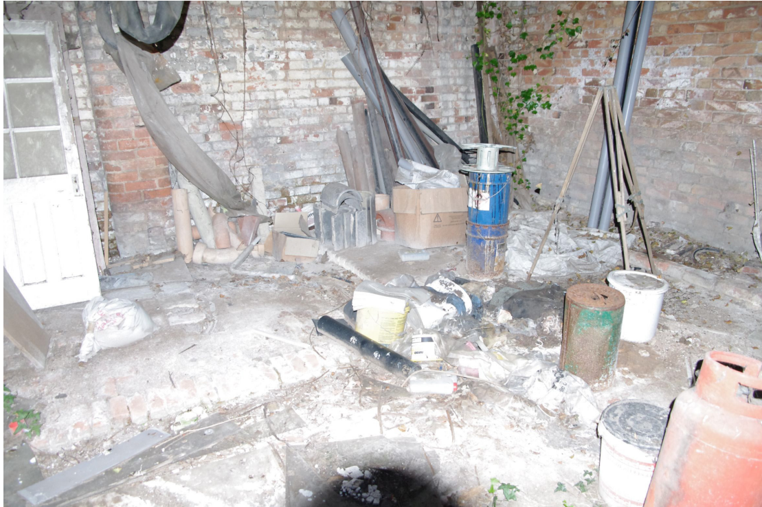
Figure 90 Barn 1, southern room Looking east at raised brick stands for cattle and byers
