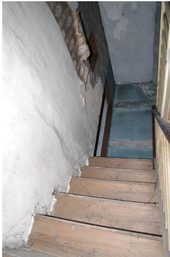
Figure 66 View up the servant's stairs to second floor Looking north-west
