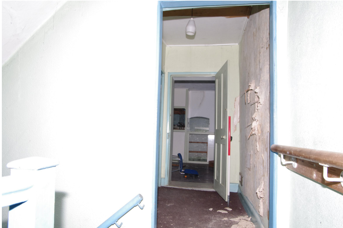
Figure 60 Room F4 seen from F1 Looking north-west towards F6. 1m scale
