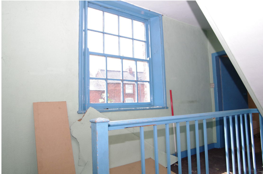
Figure 54 Window detail Room F1 Looking south. 1m scale
