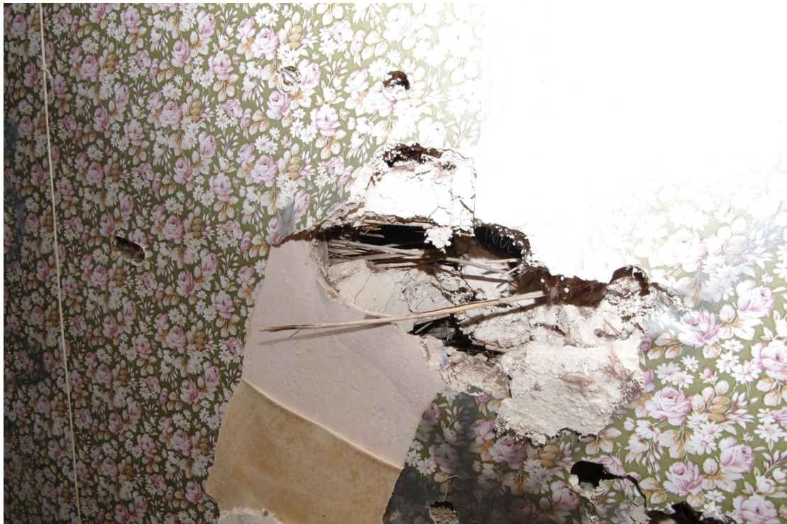
Figure 59 Wall detail of Room F3
