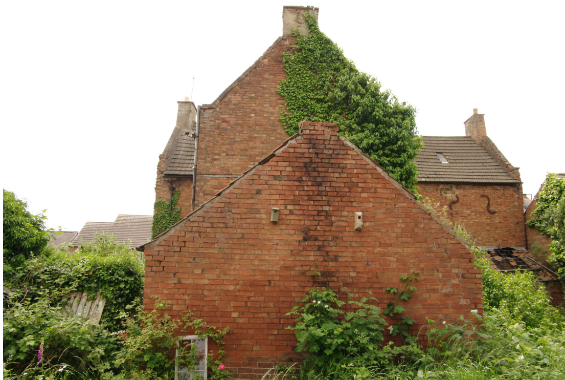
Figure 23 North-west facing elevations of farmhouse Looking south-east
