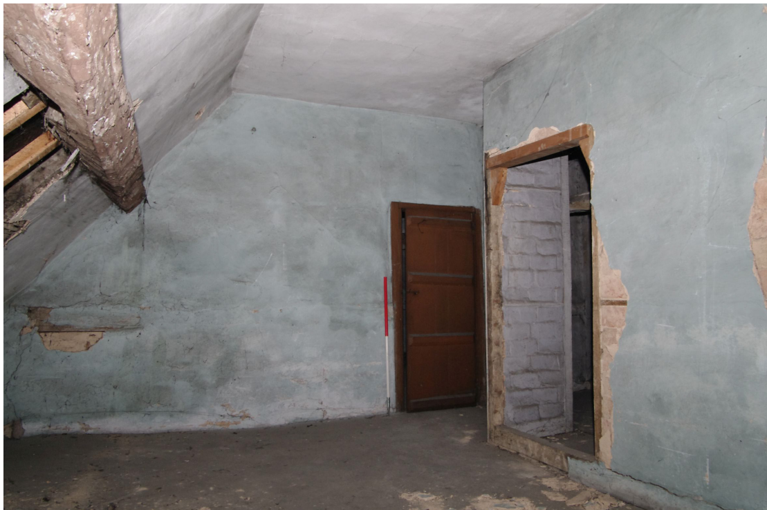
Figure 77 General view of Room S4 Looking west. The door on the right leads to Room S5. Note the use of large oversized bricks similar to “Measham or Wilkes Gobs” on partition wall on right. These date to the mid-18th century. 1m scale
