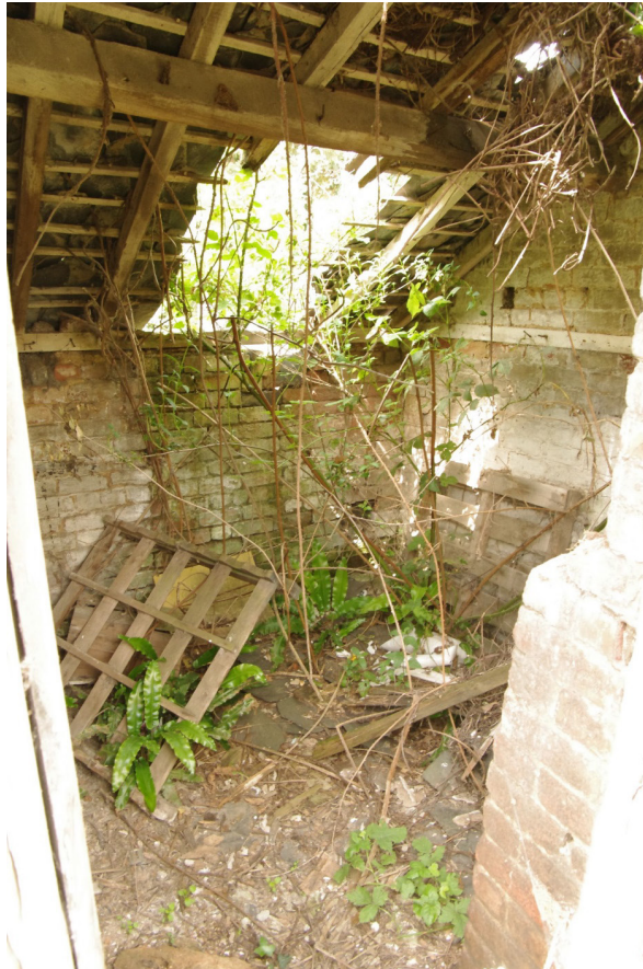
Figure 102 Inside Outbuilding 1 Looking west
