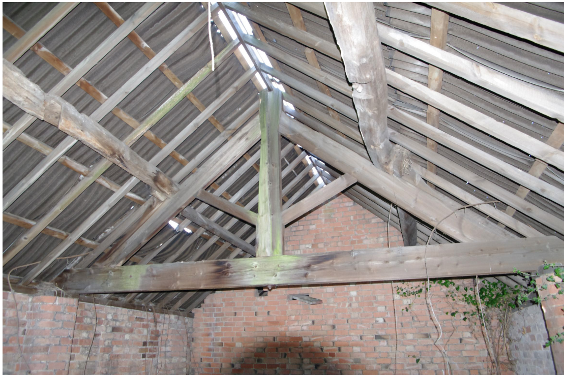
Figure 89 Barn 1, northern room Looking south-east. Note redundant sockets for braces on the purlins
