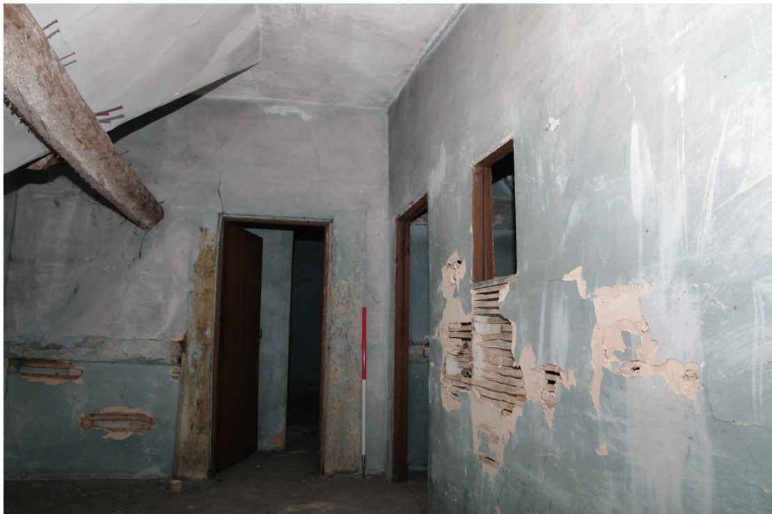
Figure 71 General view of Room S2 Looking north-west. The door on right leads to stairs and Room S1. The door on left leads to Room S4. 1m scale
