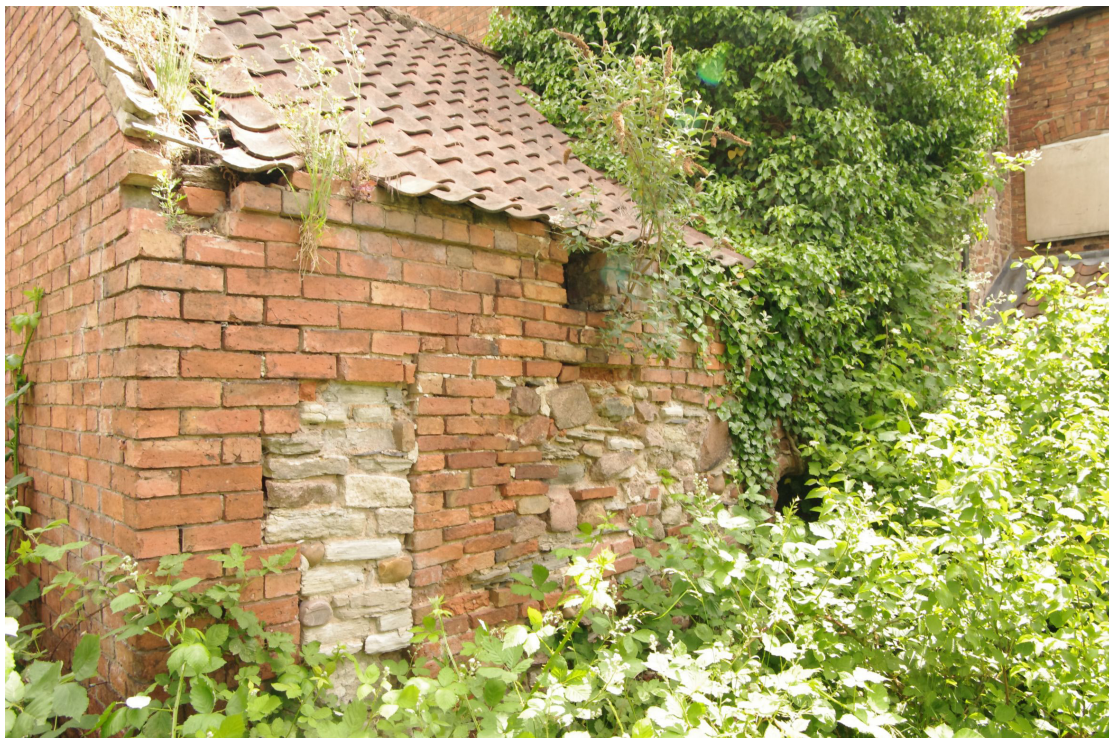
Figure 25 Remnant of stone wall in single storey rear range Looking south-east
