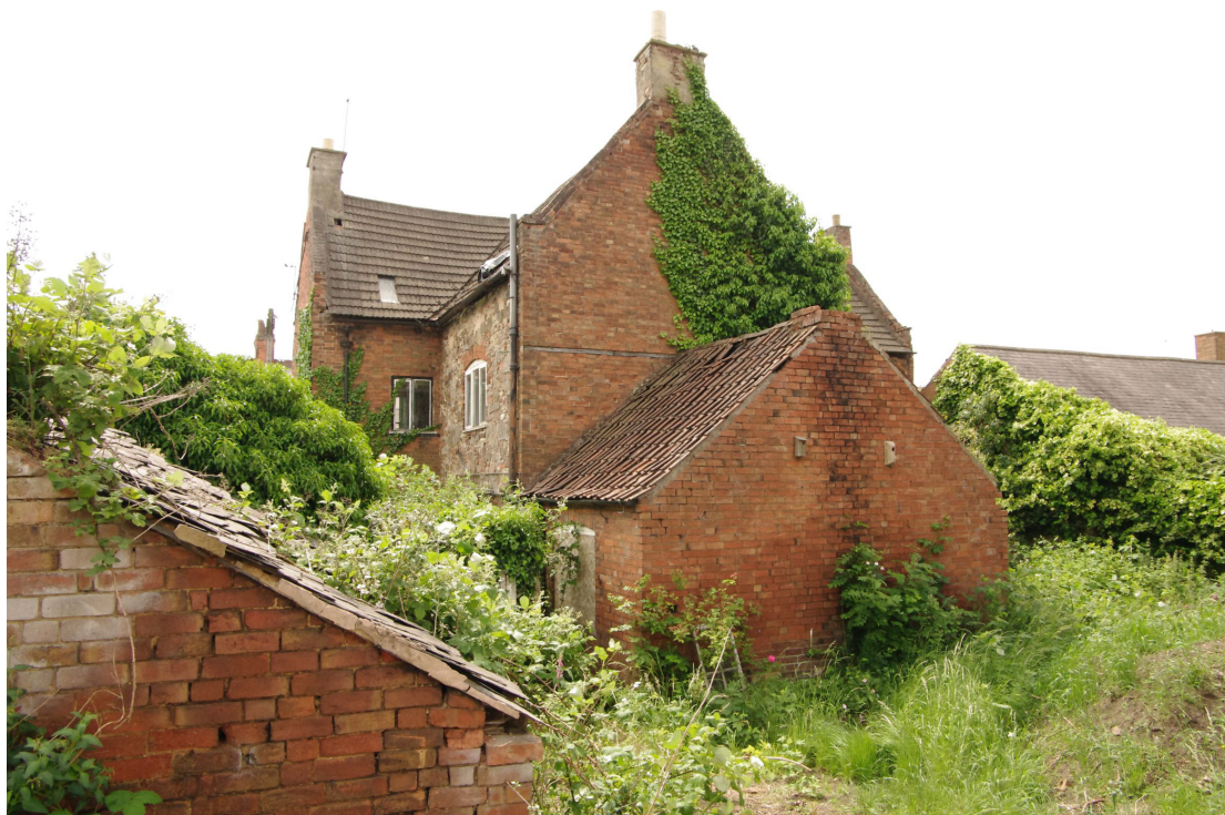
Figure 22 Rear of farmhouse looking south Note gable end of rear range is of brick suggesting stone range may have extended further. Outbuilding 1 on left
