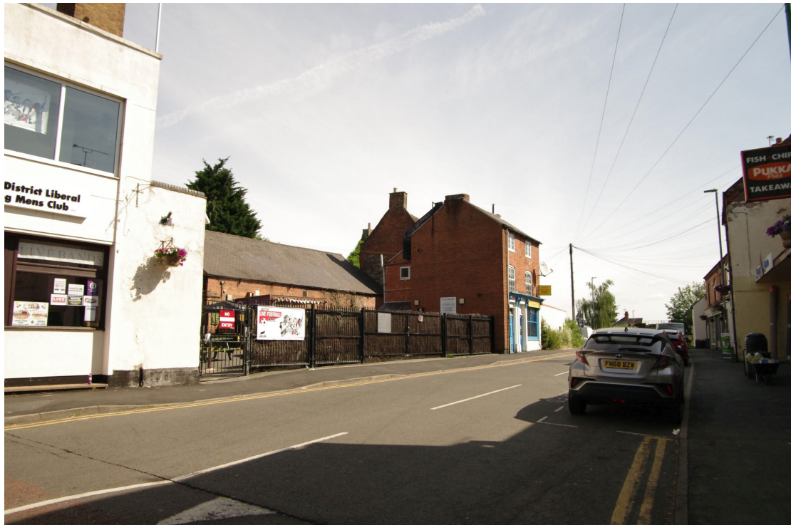
Figure 12 View along King Street looking east No. 7 is the central gable and chimney stack in this picture
