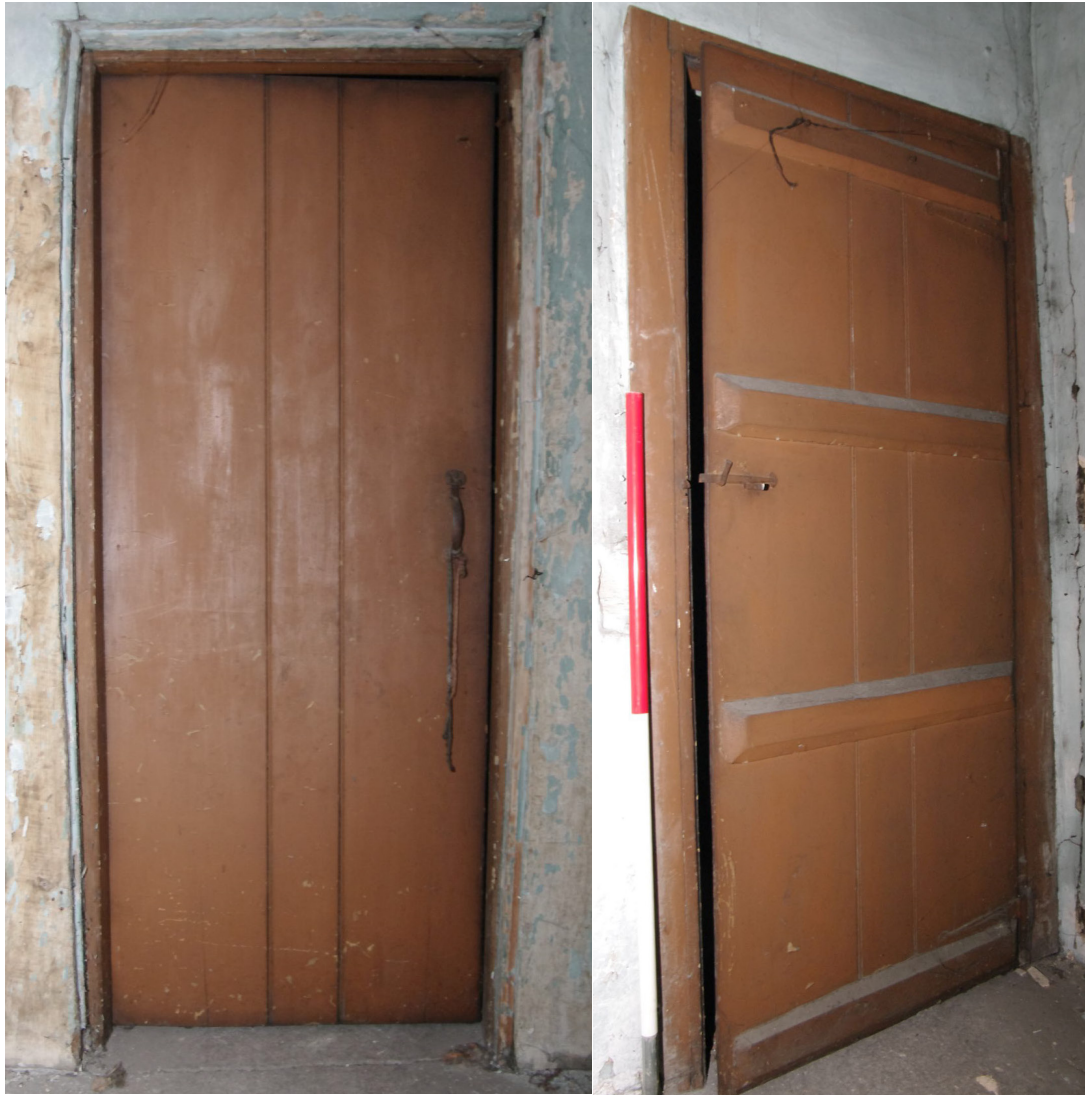
Figure 72 Detail of the door from S2 to S4
