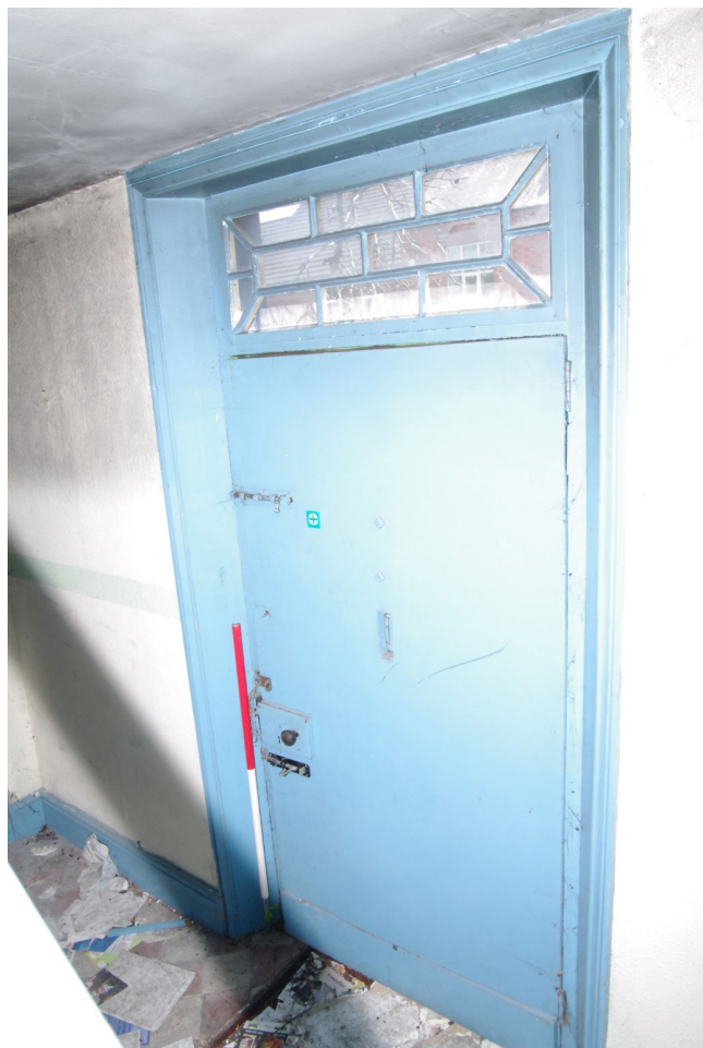
Figure 42 Hallway G4 door detail Looking east. 1m scale
