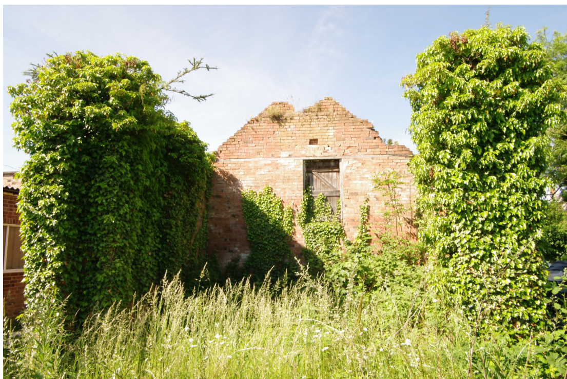
Figure 98 Barn 2, eastern room Looking south-west towards two-storey hayloft
