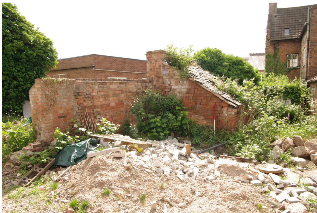
Figure 100 Outbuilding 1, north-west facing elevation Looking south-east. 1m scale
