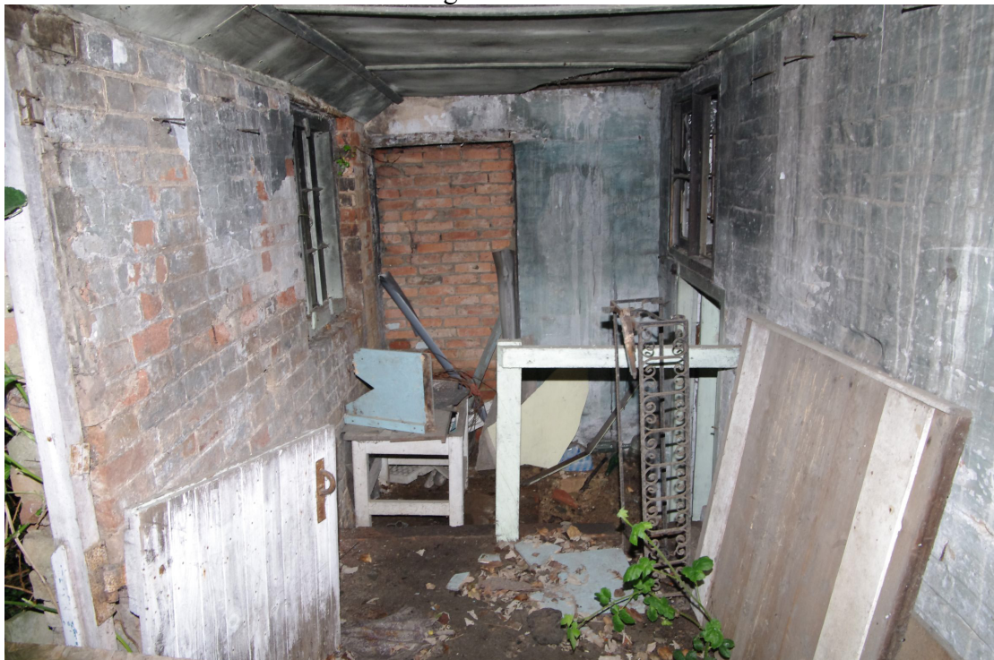
Figure 51 Room G8 lean-to Looking north-west. The white rail marks the top of the cellar stairs. Evidence of a blocked doorway on far wall leading into G1 (see Fig. 31)
