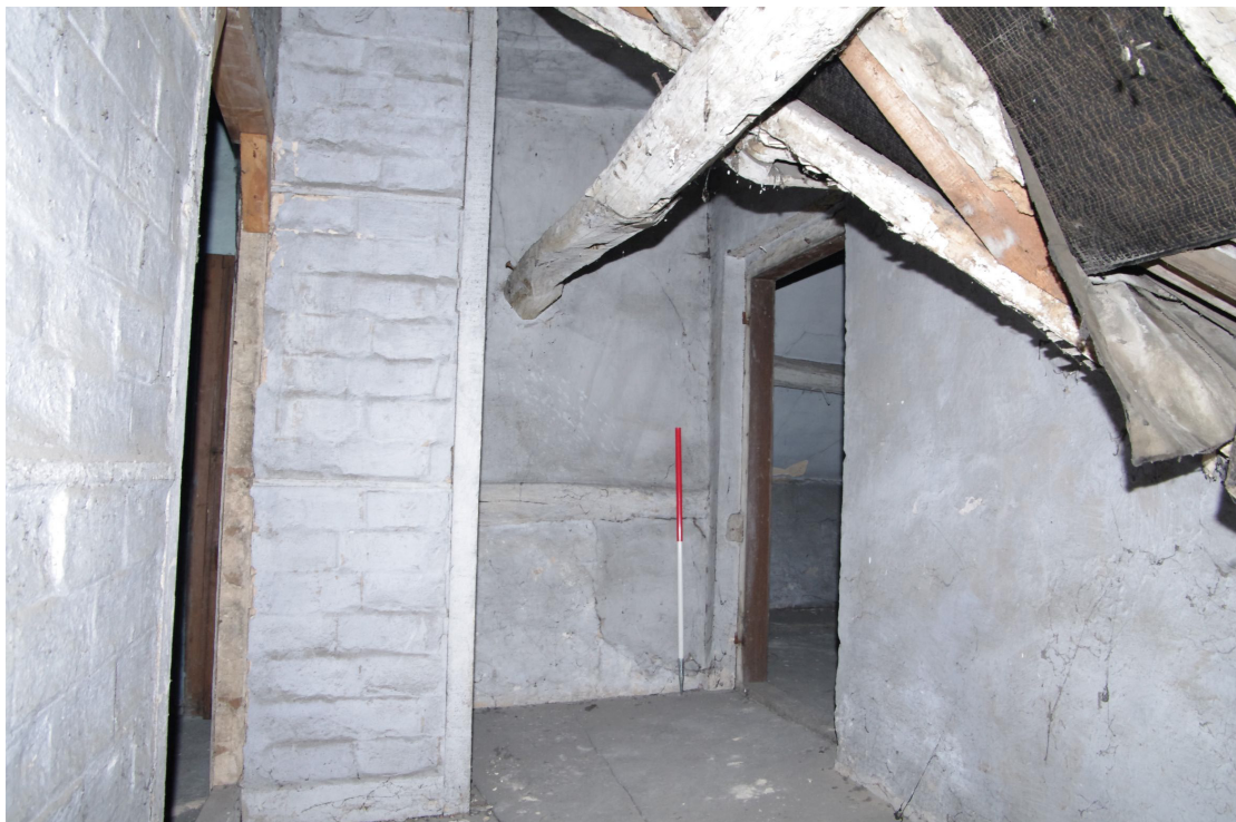
Figure 81 General view of Room S5 Doorway to Room S4 on left, S6 on right. The purlin has many redundant sockets and peg holes (see next image). 1m scale
