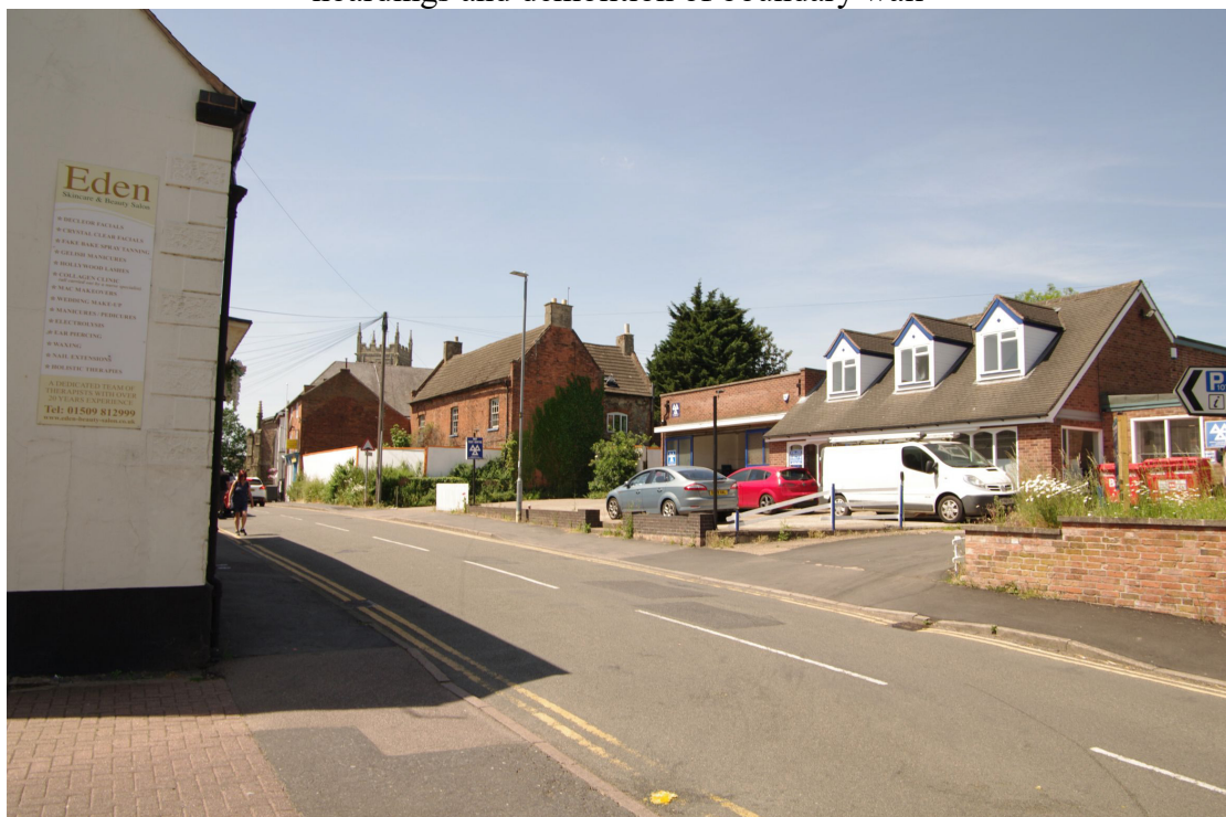
Figure 11 View along King Street looking north-west Hoardings around building now present. Garage on right is located where the courtyard range of agricultural building were
