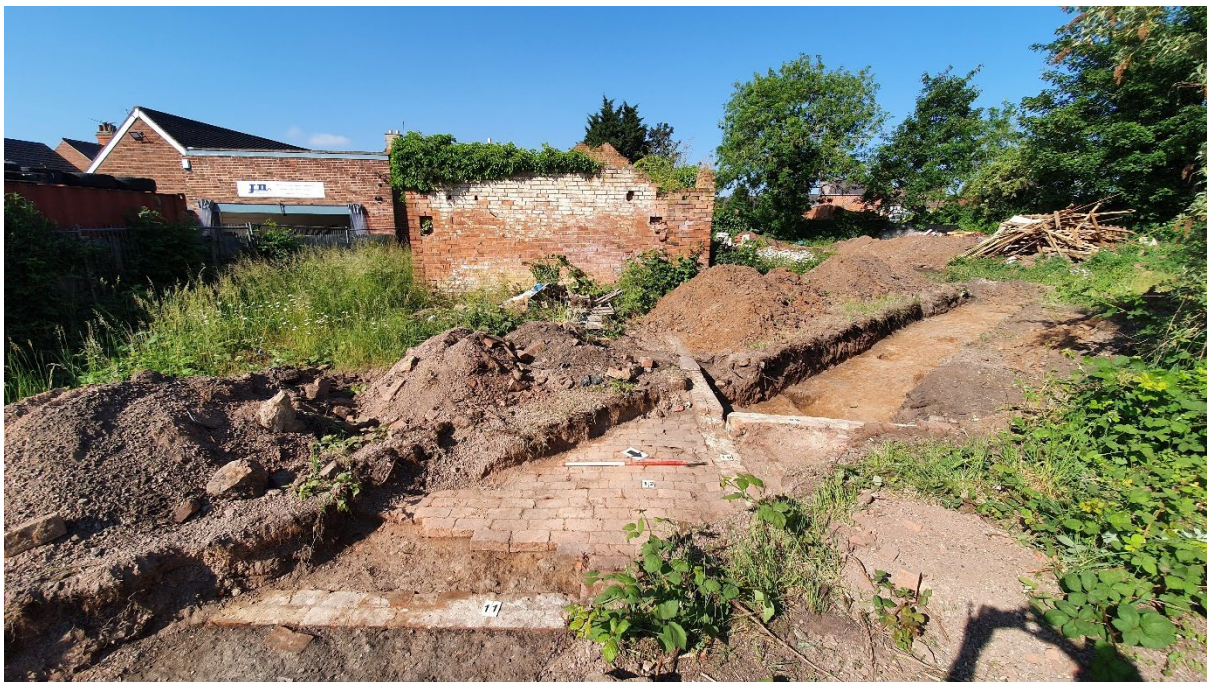
Figure 13: Trench 2: east end of trench; view west (1m scale)
