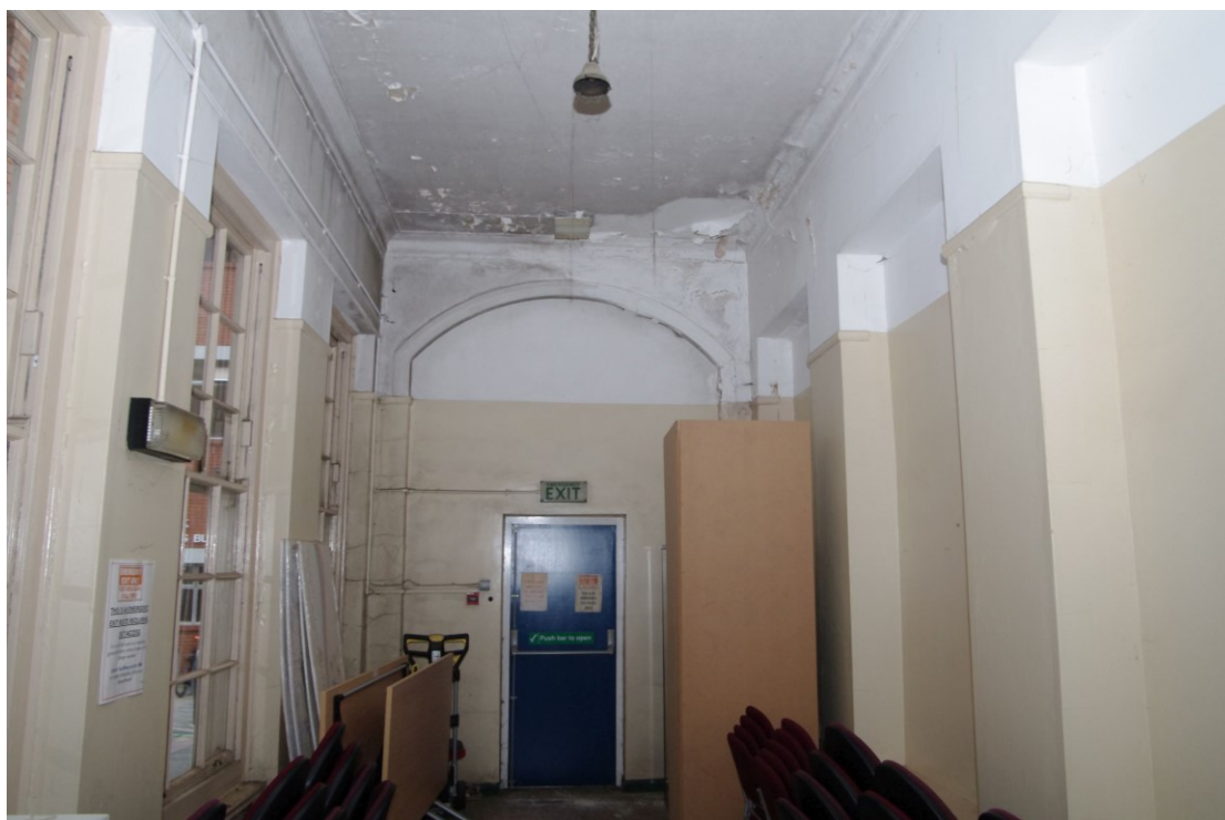
Figure 59 Ground floor: east to west corridor Looking west towards the blocked arch which continued across the entire 1910 range. The blind arcades on the right may have held windows which were blocked following the construction of the theatre
