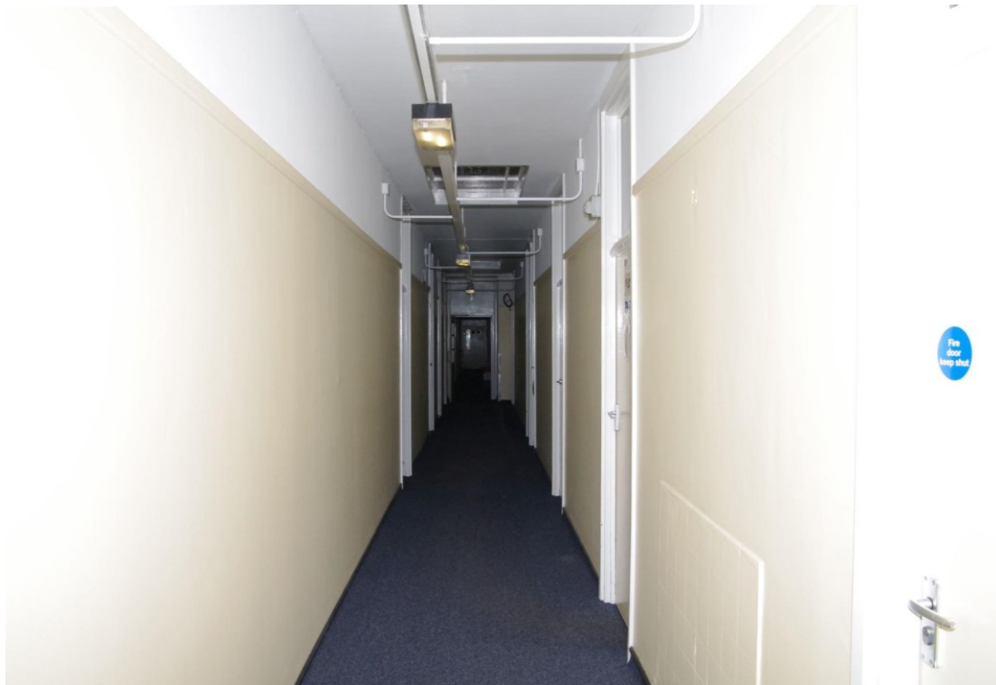
Figure 137 Third floor, later 1930s north to south corridor Looking north. Noted painted over glazed brick panel in foreground on right
