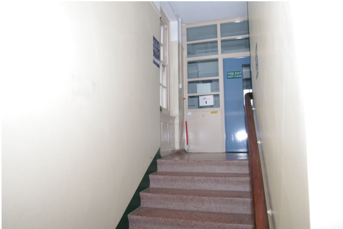
Figure 96 1910 stairs to first floor Looking south-east. 1m scale
