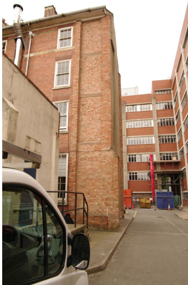
Figure 22 Scarring left on north side of 1910 range Note the new bricks on the right mark where one of the rear ranges extended towards the white van in the foreground. Looking south. 1m scale
