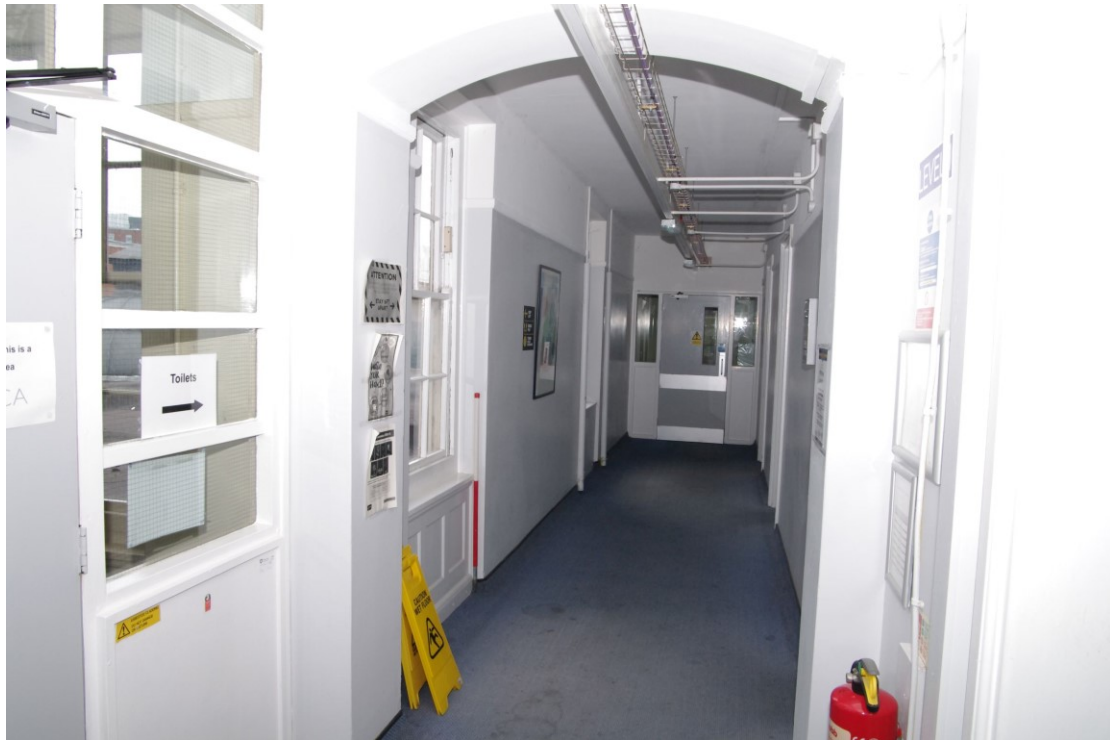
Figure 97 1910 rear north to south corridor Looking north. Stairs on left. Toilet block and lift beyond modern door. 1m scale
