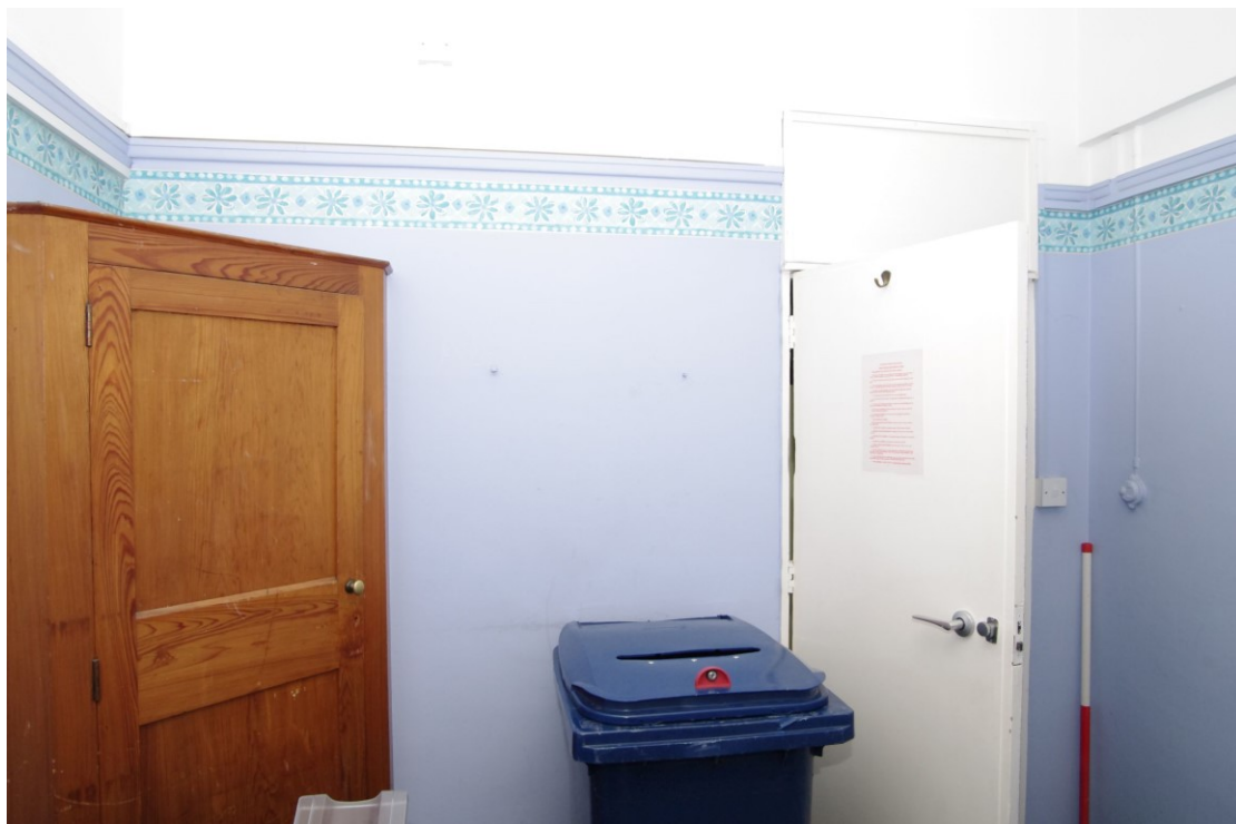
Figure 108 First floor: first phase 1930s north to south corridor. West side Looking east. Note light switch and original coat hook on door. 1m scale
