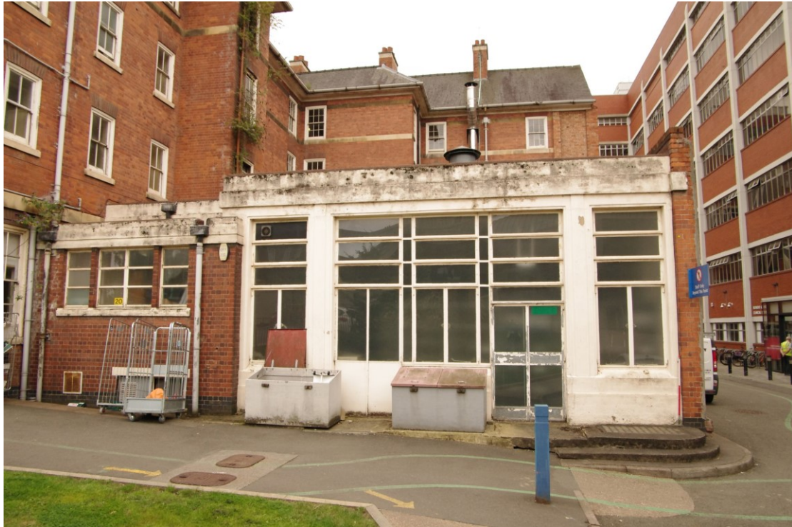
Figure 25 Close-up of the north facing elevation of the theatre Looking south
