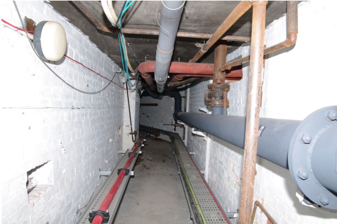
Figure 49 Basement: service tunnel Looking east. Corridor leads towards the Outpatients Building
