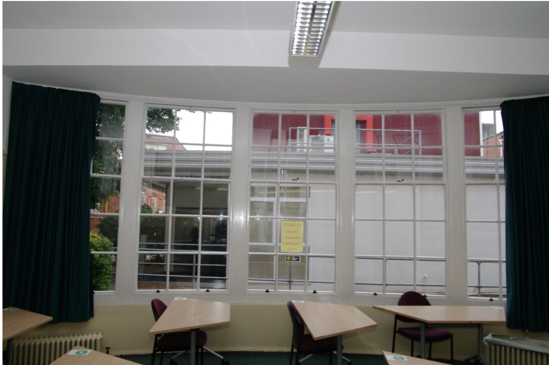
Figure 92 Ground floor: bow window detail Looking east. Note the low radiators. See also Figure 91
