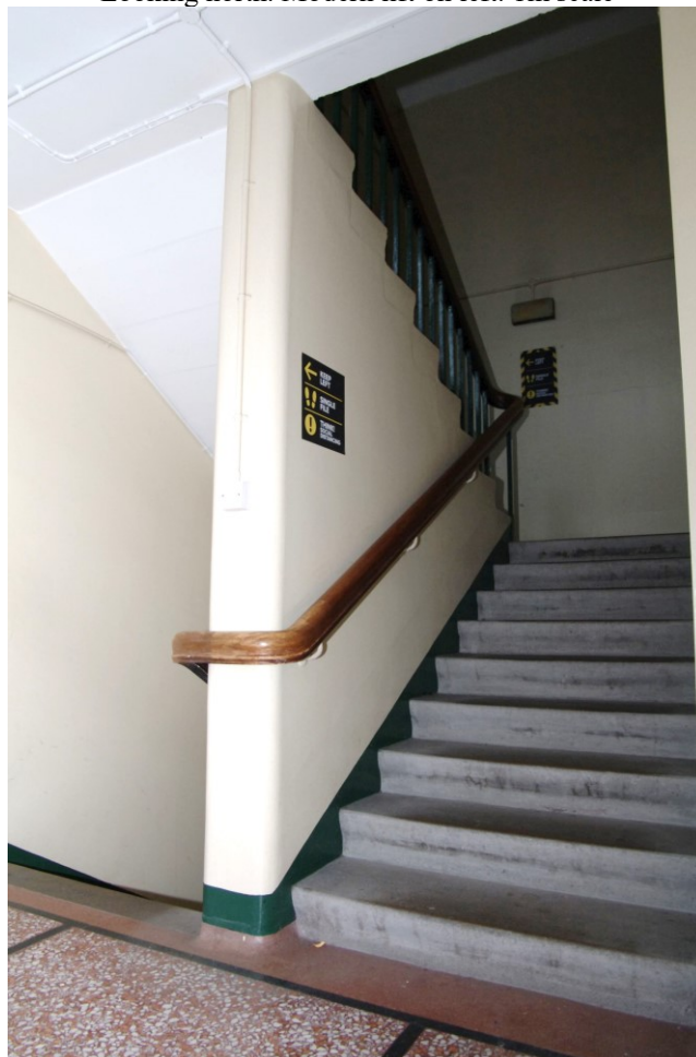
Figure 122 Second floor: 1930s stairs Looking south-east
