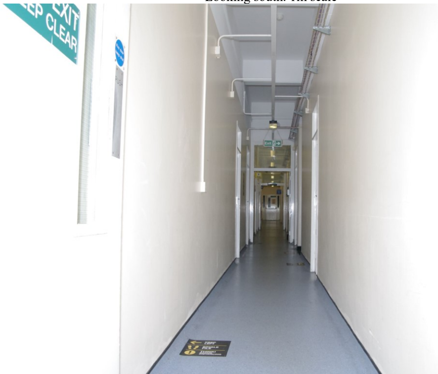
Figure 83 Ground floor: 1930s extension north to south corridor Looking south. The far double doors mark the joint between the two 1930s phases
