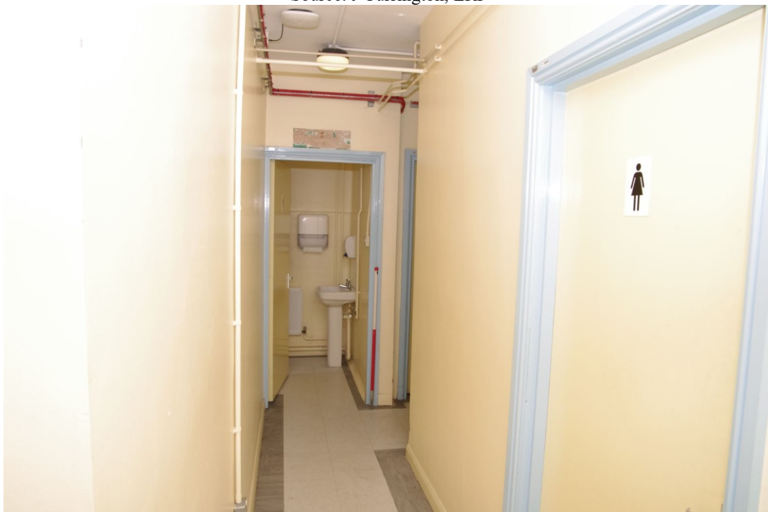
Figure 100 First floor: 1910 rear corridor, toilet block Looking north. 1m scale
