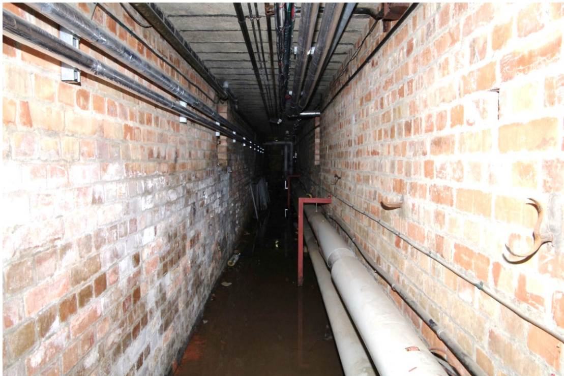
Figure 52 Basement: corridor beneath 1930s extension Looking south
