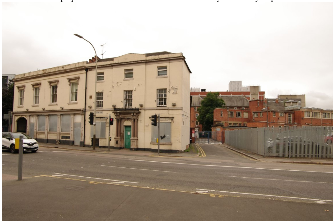
Figure 15 Remnant of Knighton Street seen from Aylestone Road Looking west. Only one of the two pubs on Knighton Street survive. The slate roof of the nurses’ home can be seen just below the skyline
