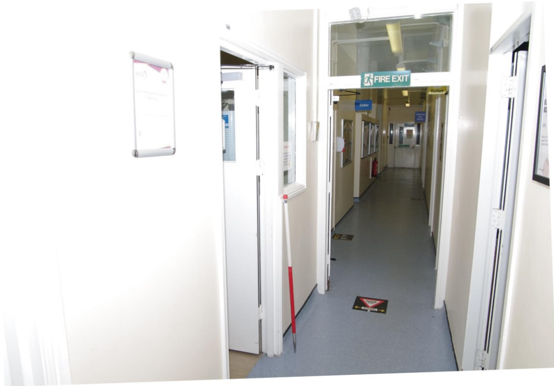
Figure 84 Ground floor: junction between the two 1930s phases Looking south. Toilets either side in foreground. Note how the corridor widens beyond the doorway
