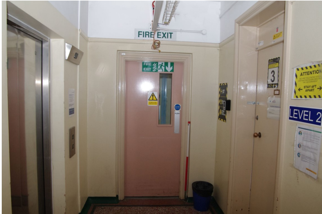
Figure 121 Second floor, 1910 north to south corridor: toilet block Looking north. Modern lift on left. 1m scale
