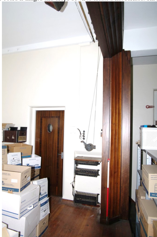
Figure 69 Recreation room/theatre: stage curtain winding gear Looking south. Note the door to the left which leads into the wings and changing rooms. 1m scale
