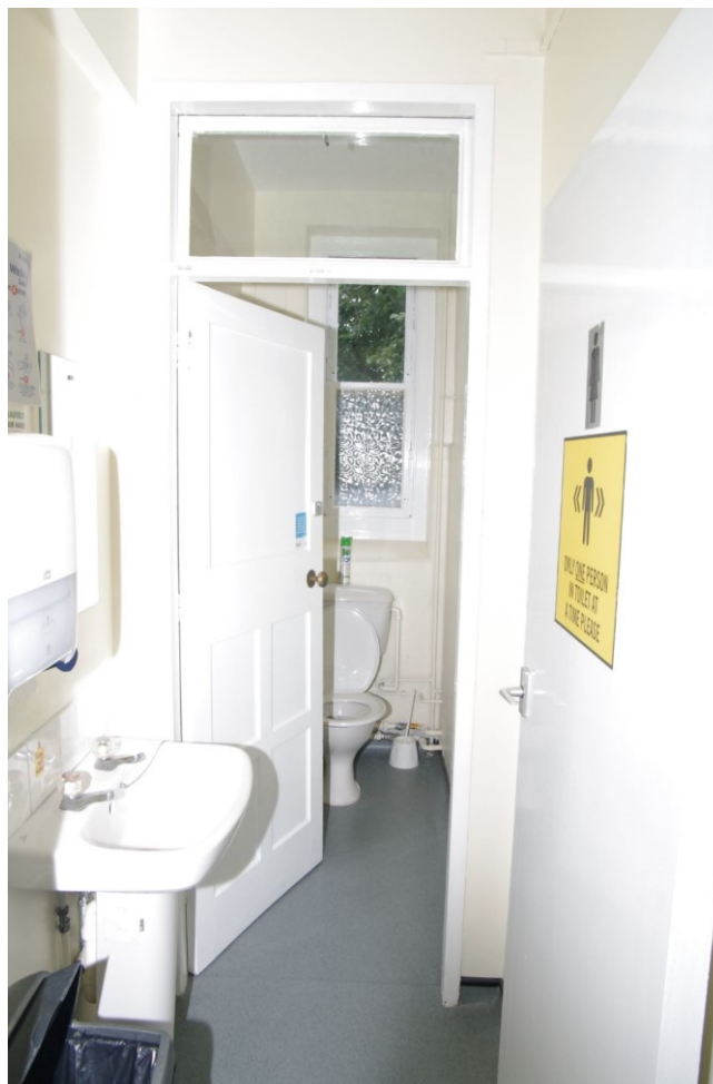
Figure 125 Second floor, first 1930s extension: toilet block Looking east. Note fanlight above panelled door
