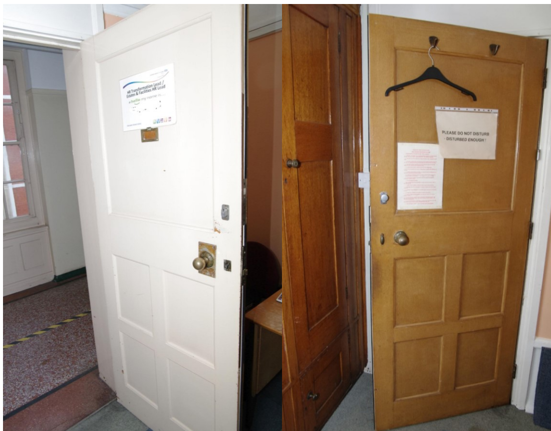
Figure 116 Second floor, 1910 north to south corridor: door detail Note brass door fittings and fitted cupboard. Room 217
