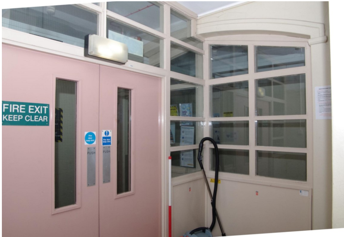
Figure 115 Second floor: top of 1910 stairs Looking south-east. 1m scale
