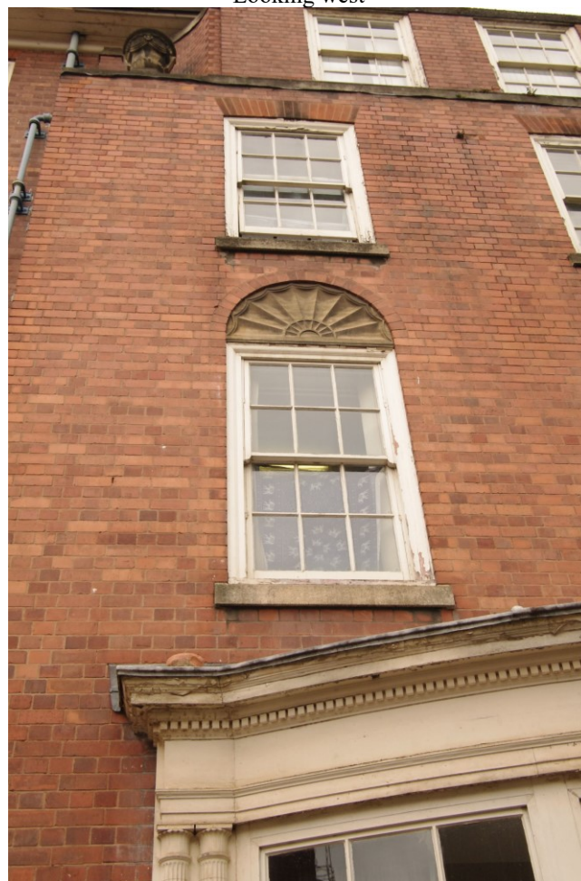
Figure 42 Decorative detail of east facing bay Looking west
