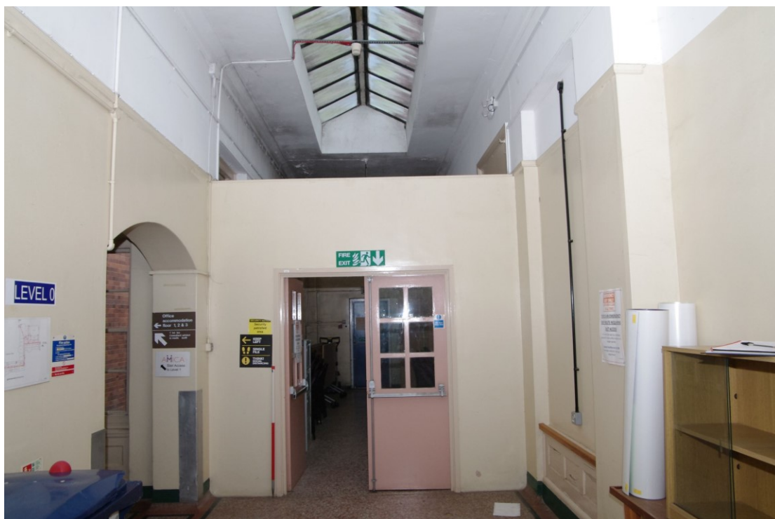
Figure 58 Ground floor: rear east to west corridor Looking west. The archway on the left leads to the stairs to the basement and upper floors. See also Figure 59
