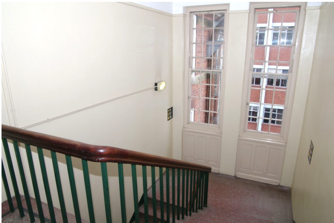
Figure 131 Third floor: top of 1910 stairs Looking south-west
