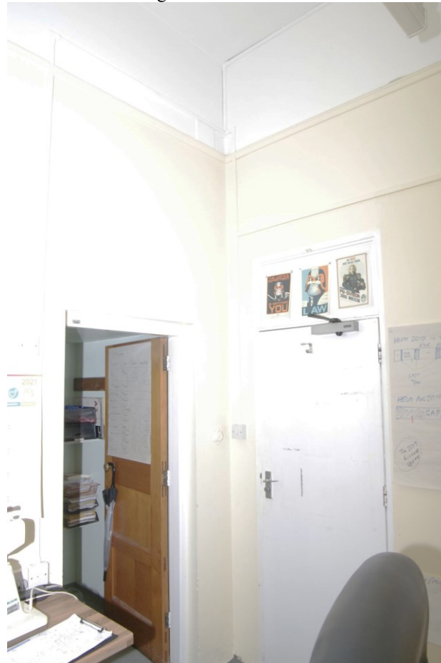
Figure 85 Ground floor: earliest 1930s phase room Looking north-east in Room 044. Note panelled door to cupboard beneath the stairs
