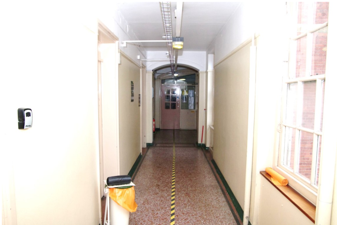
Figure 118 Second floor: terrazzo floor
