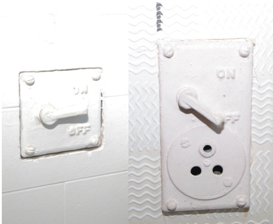
Figure 128 Second floor, later 1930s extension: swith and socket detail
