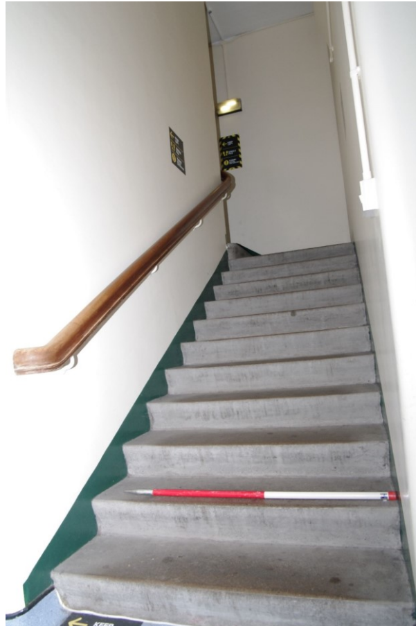
Figure 82 Ground floor: 1930s extension stairs Looking south. 1m scale
