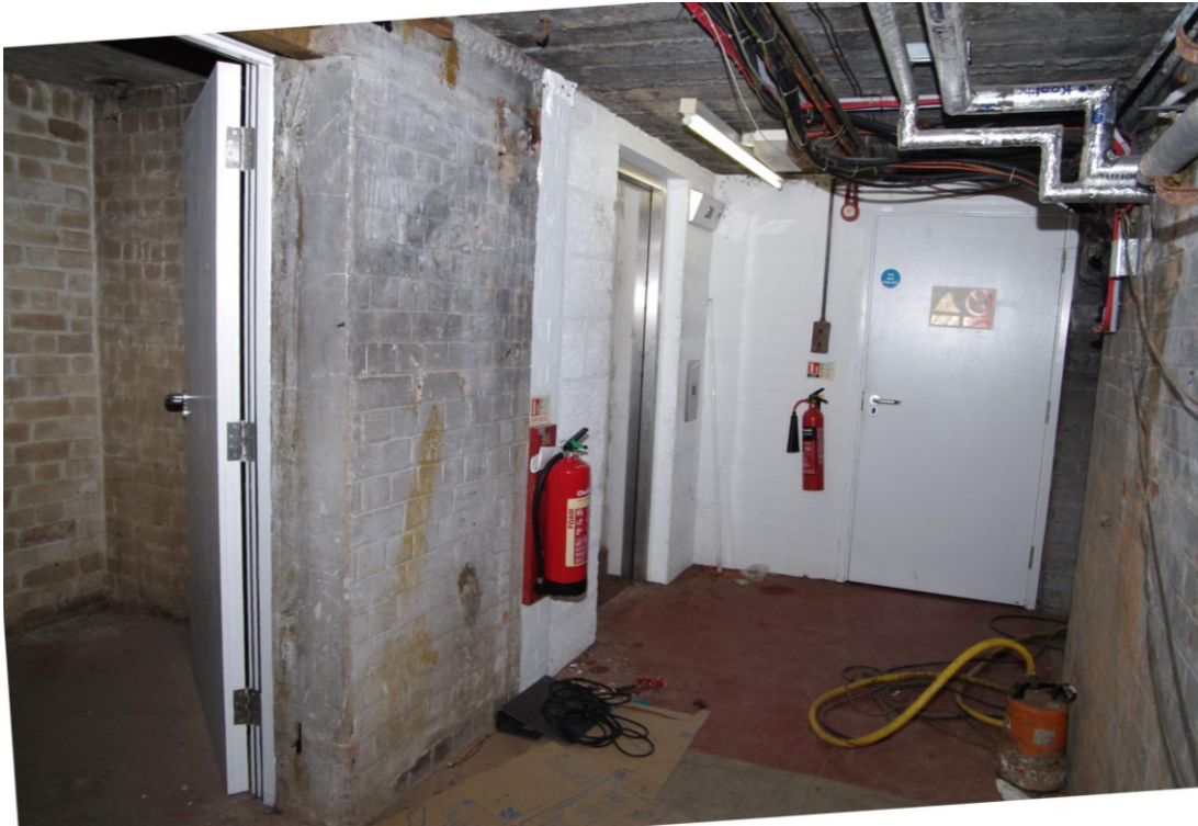
Figure 47 Basement corridor with lift shaft on left Looking north-west
