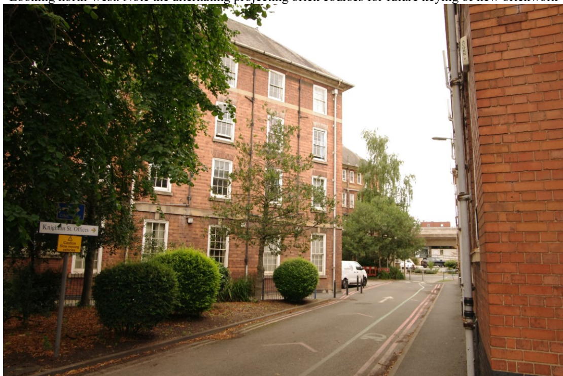
Figure 38 East facing elevation of earliest 1930s extension phase Looking north-west. Rear of 1910 range visible above the white van. Outpatients Building on right
