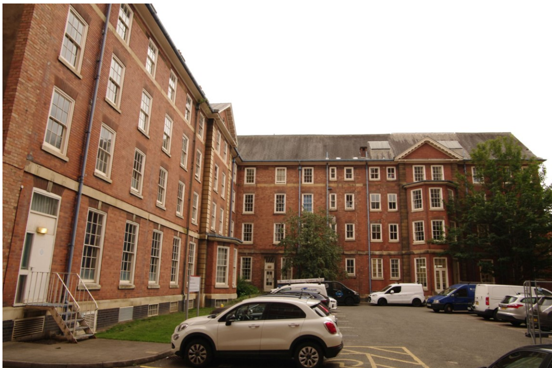
Figure 32 West facing elevation of 1930s extensions Looking east. 1910 range on left. Compare with Figure 33
