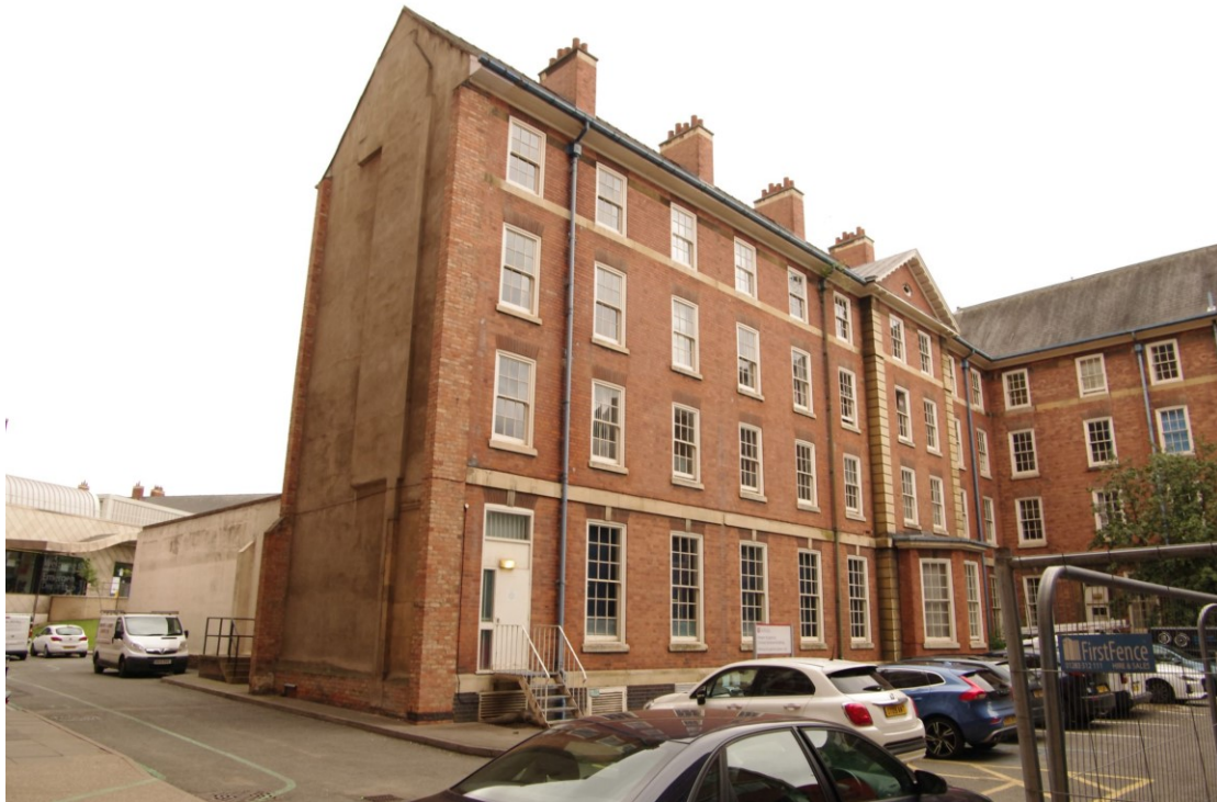
Figure 21 South facing elevation of the 1910 range Looking north-east. Later east wing extension on right
