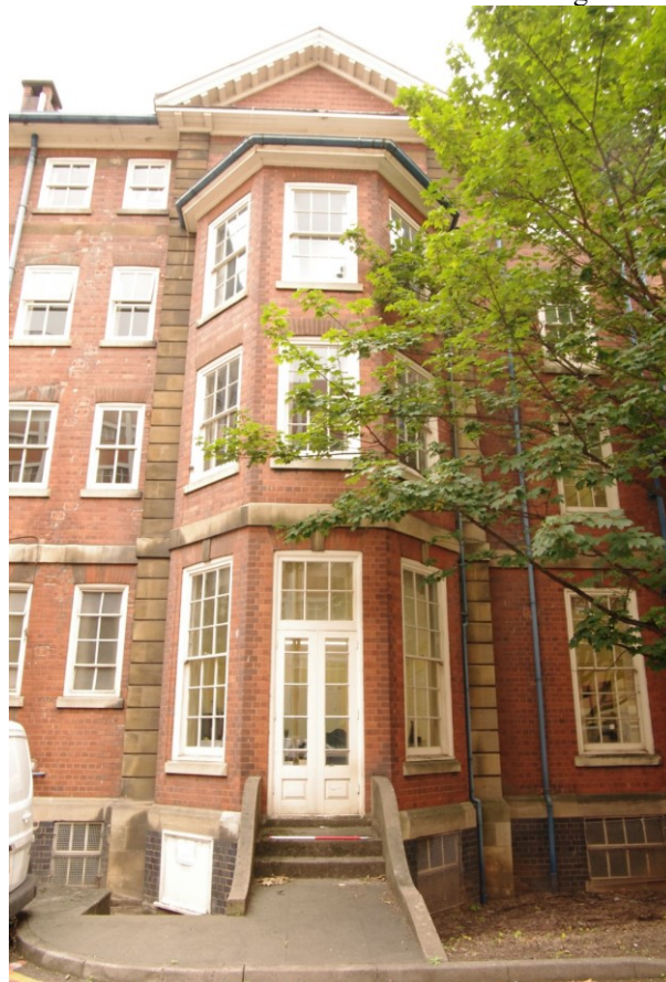
Figure 34 Detail of the 1930s extension west facing bay Looking east. Note the small bridge from the French windows. 1m scale
