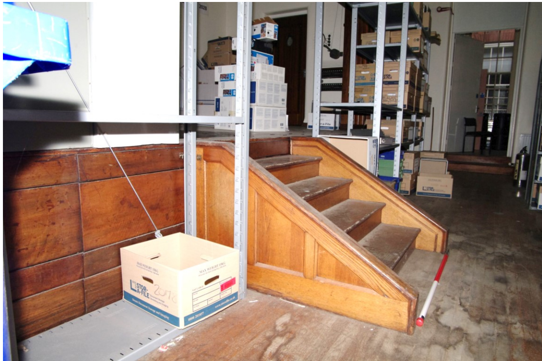
Figure 66 Recreation room/theatre: stage steps Looking south-east. Note the step up to the outside corridor to the right. 1m scale
