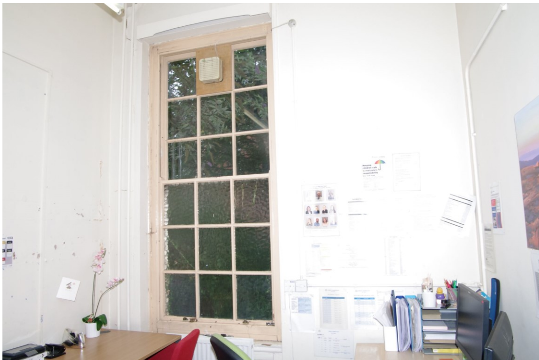
Figure 55 Ground floor window detail
