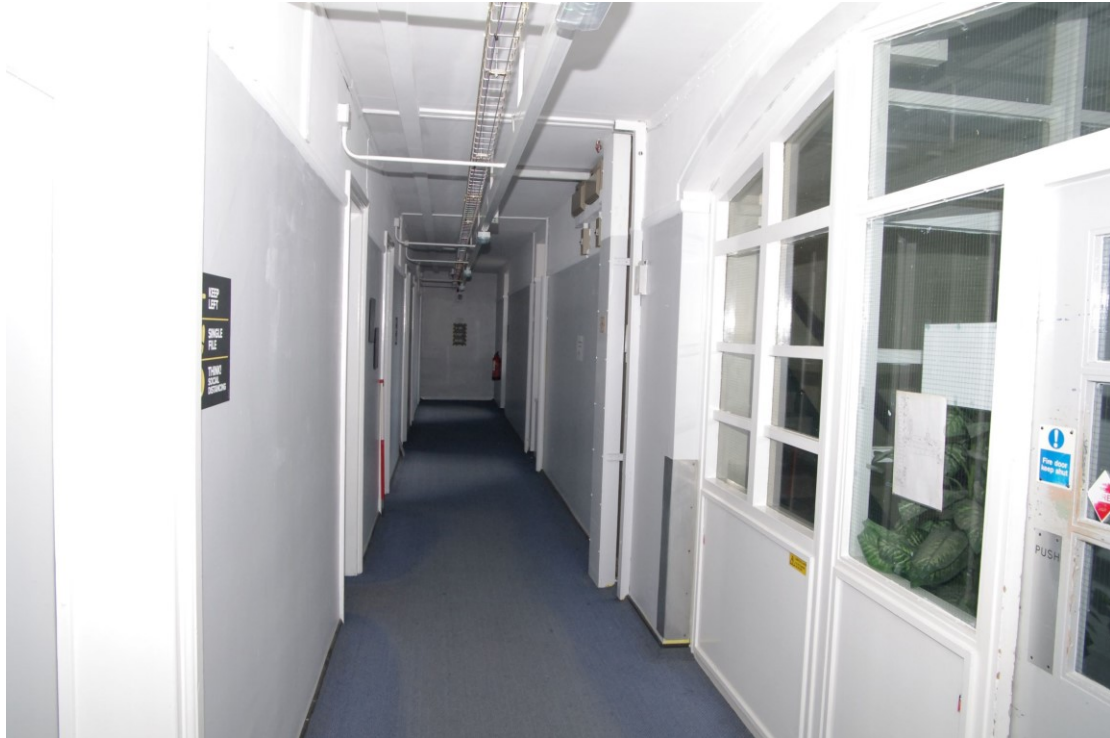
Figure 101 First floor: 1910 east to west corridor Looking west. Stairs on right. 1m scale
