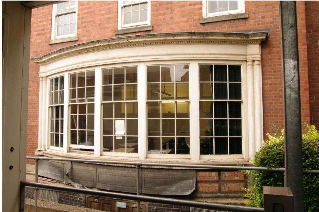
Figure 41 Detail of bay window Looking west
