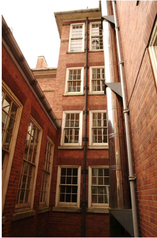
Figure 23 North side of the 1910 range. Former light well Looking east
