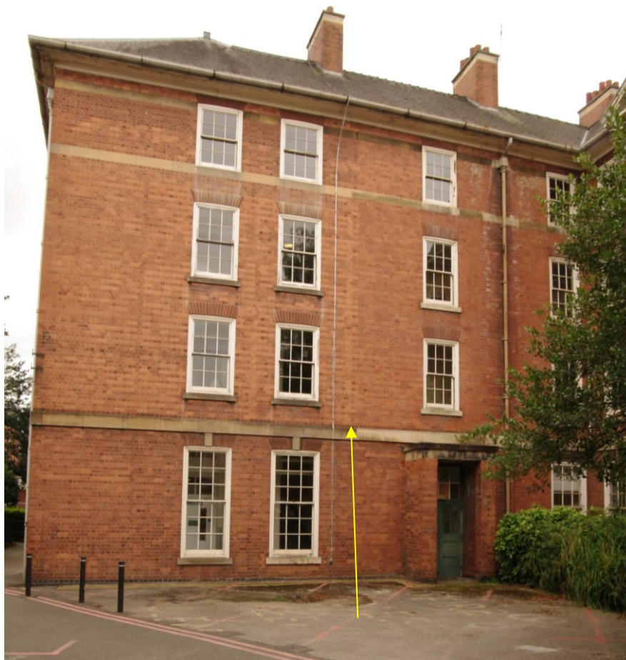
Figure 30 North facing elevation of 1910 range and later extension Looking south. The joint between the 1910 range (on right) and the 1930s extension (on left) is shown by the arrow
