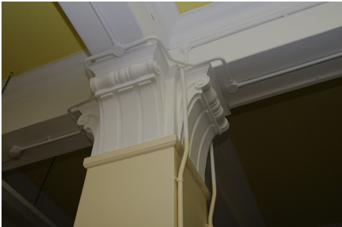
Figure 75 Ground floor: Room 049 decorative capital
