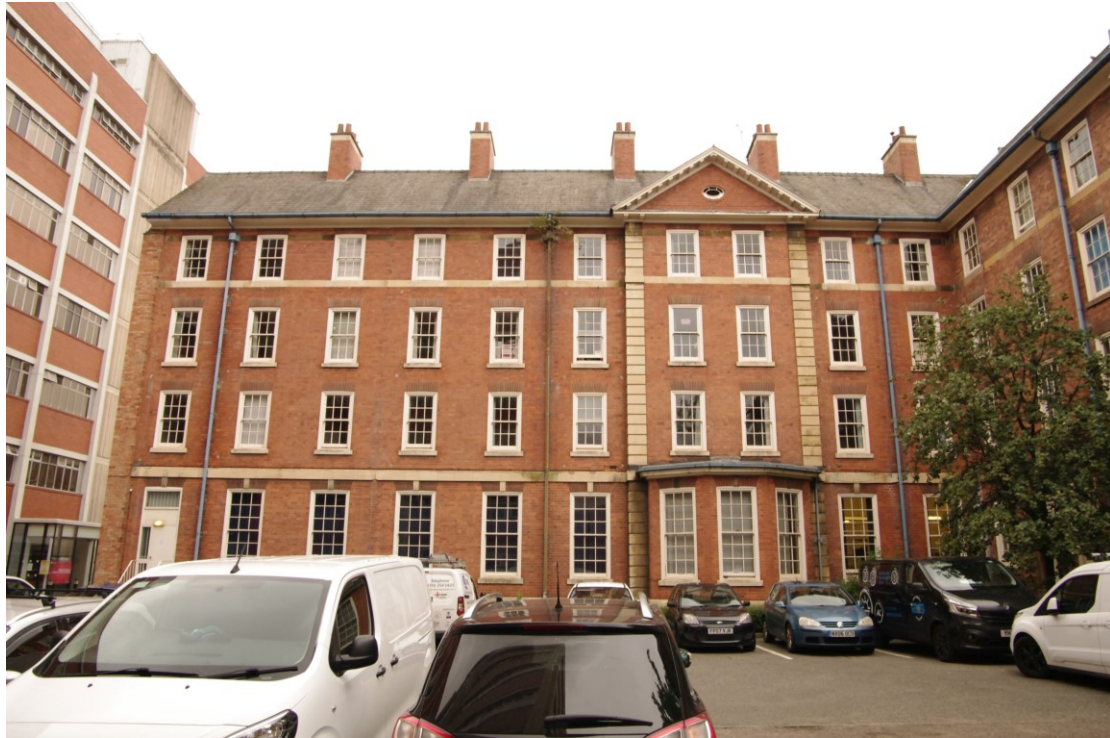
Figure 19 South facing elevation of the 1910 range Looking north. The original main entrance was to the left of the current edge of building. Compare with Fig. 5. See also Appendix 1
