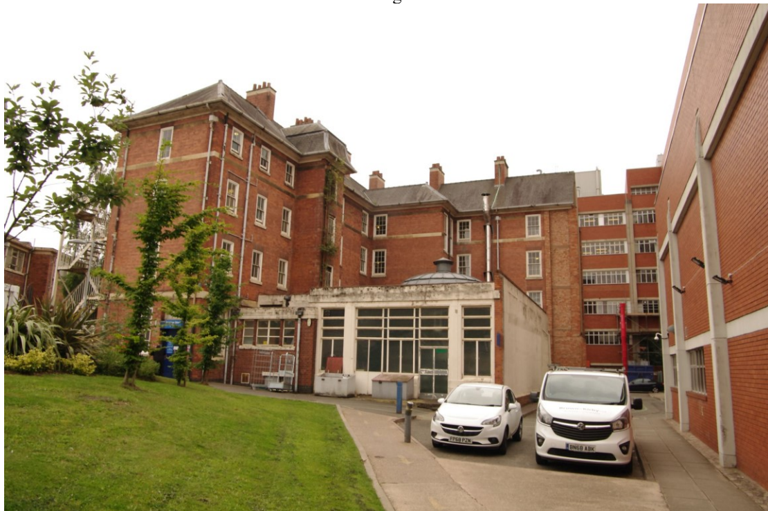
Figure 24 Rear of the 1910 range and 1930s theatre Looking south-east. Clinical Sciences building on right.
