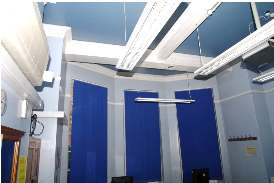
Figure 57 Ground floor: window and ceiling detail Looking east
