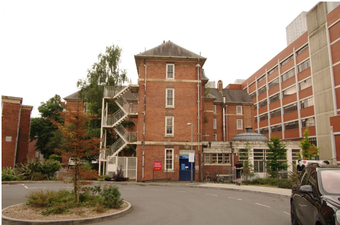
Figure 17 Knighton Street Offices seen from the north
