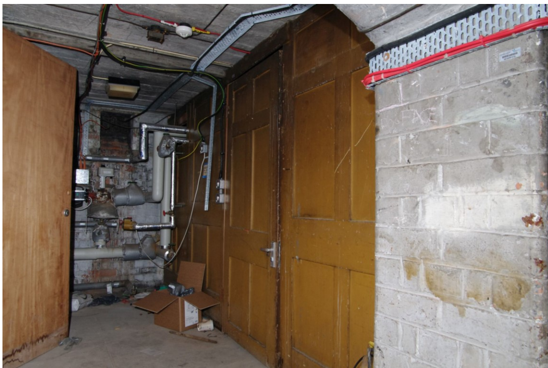
Figure 48 Basement: panelled cupboard in Room 1012 Looking north-east
