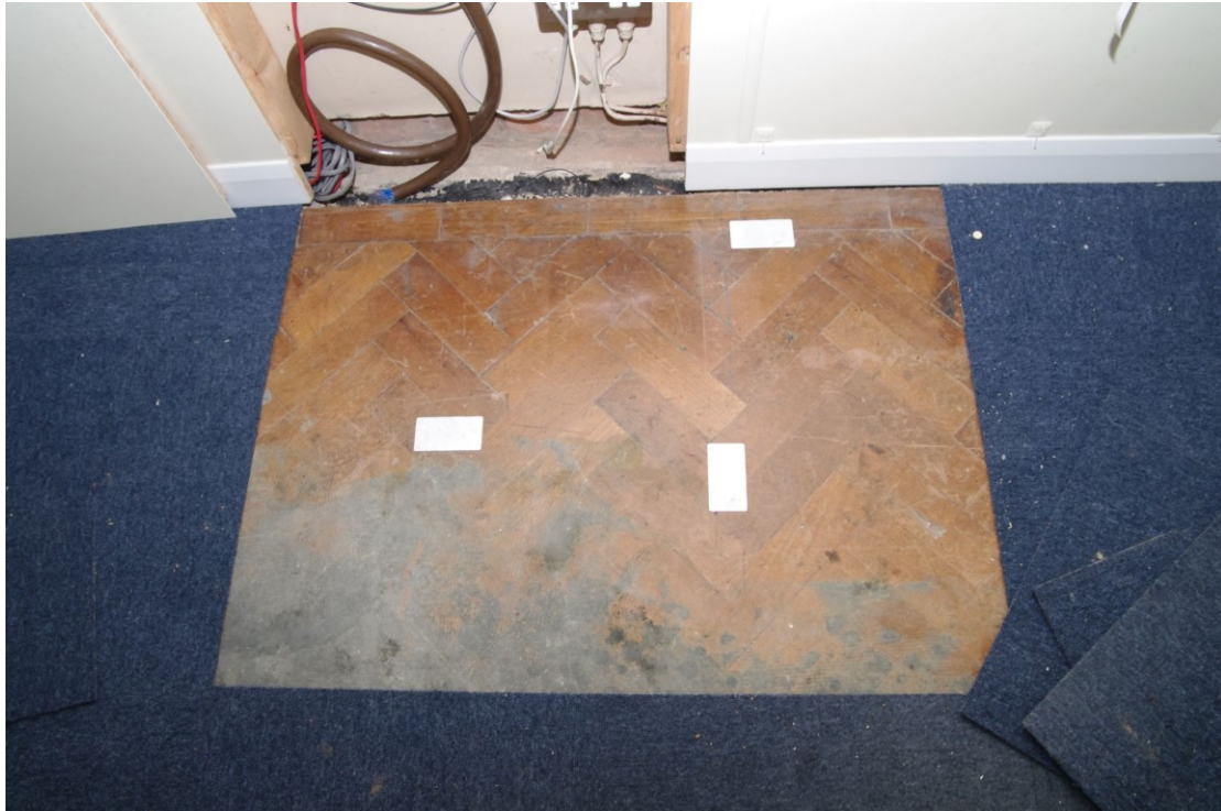
Figure 127 Second floor, later 1930s extension: wooden flooring beneath carpet
