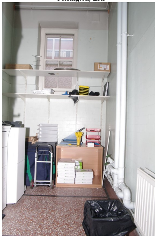
Figure 89 Ground floor: south end of first 1930s phase Looking east. Note terrazzo floor
