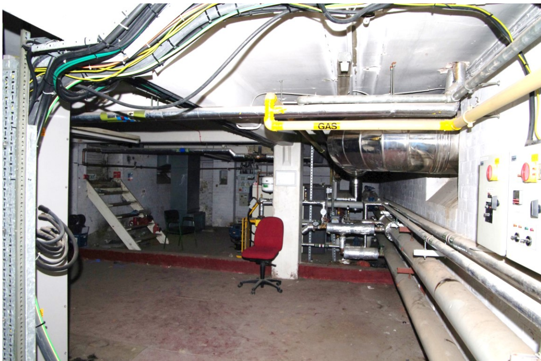
Figure 50 Basement: Room 1021 beneath 1910 range Looking south-west
