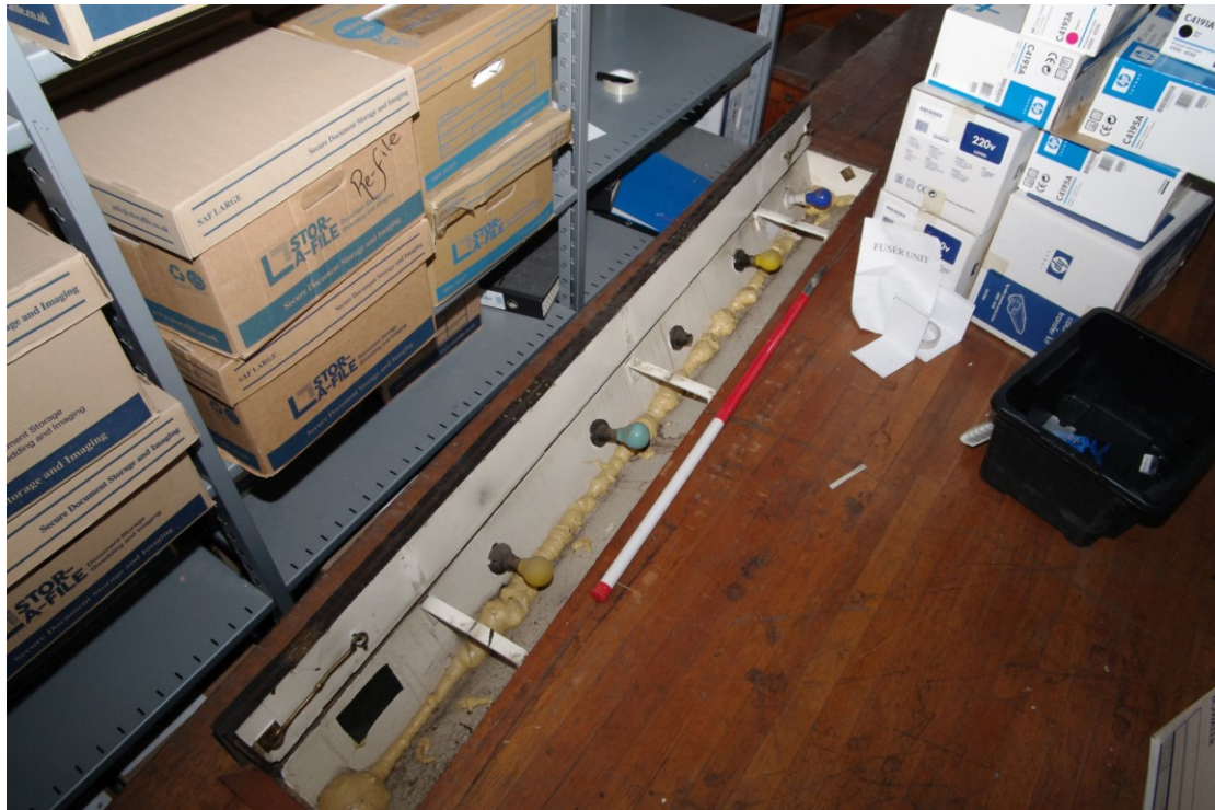
Figure 68 Recreation room/theatre: footlights set into the stage The board is hinged and drops down to create a flat surface. 1m scale
