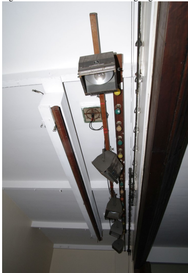
Figure 71 Recreation room/theatre: stage lights, curtain rails and drop down screen
