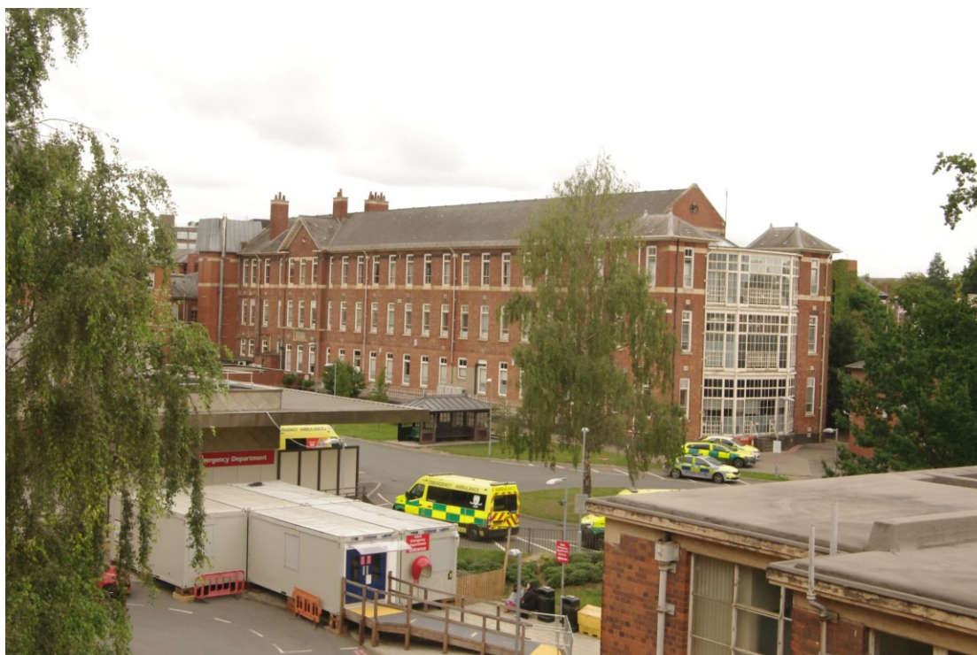
Figure 18 View of the earliest hospital buildings Looking north-east from the third floor of the Knighton Street Offices
