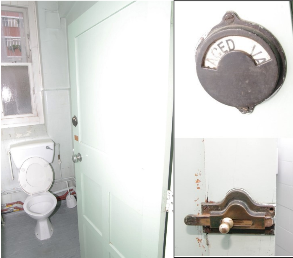
Figure 109 First floor: first phase 1930s north to south corridor toilets Note paneled door. Fittings shown on right
