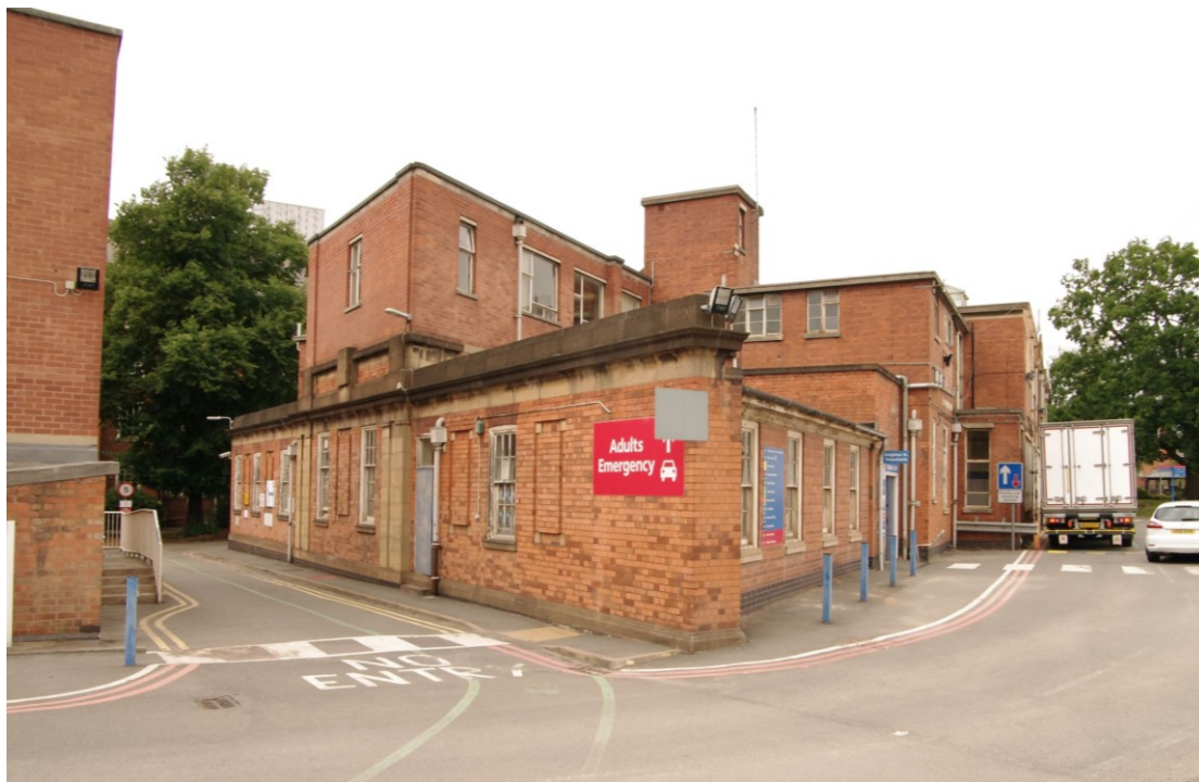
Figure 15 South facing elevation Looking north-east
