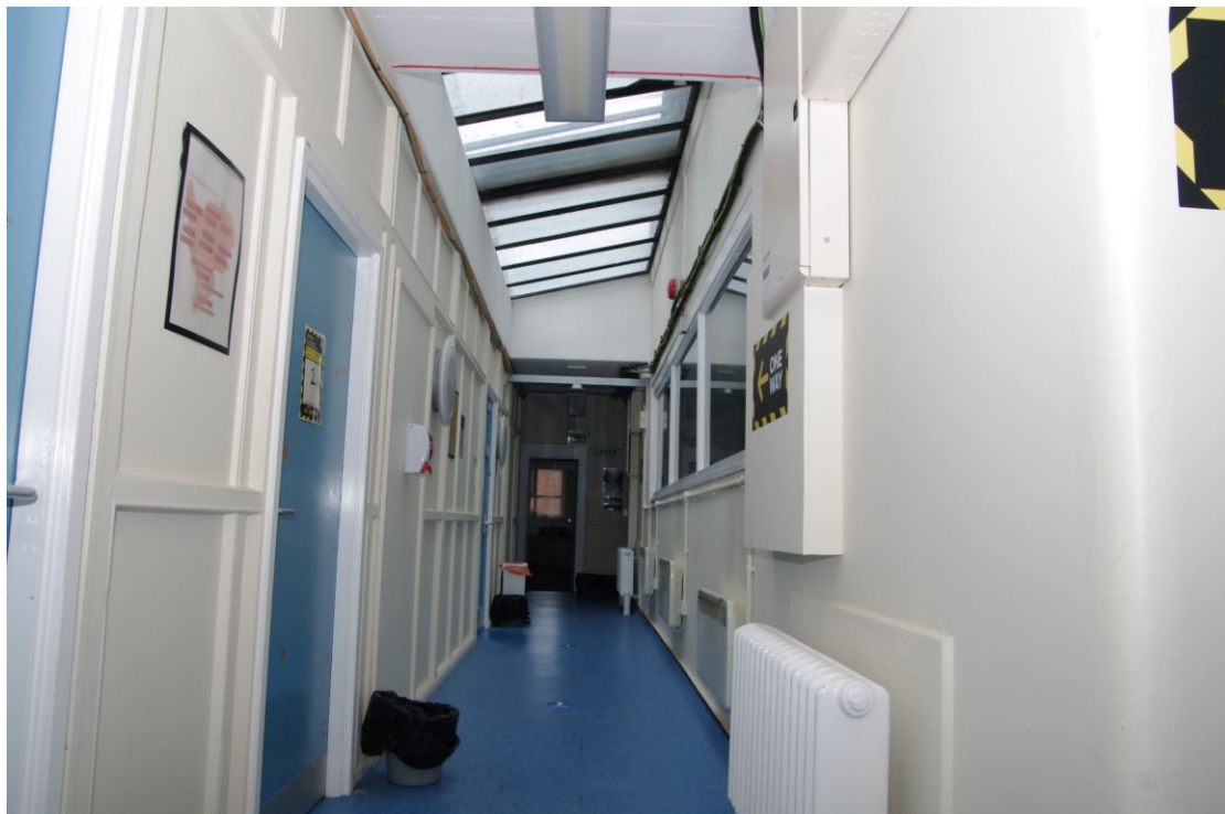
Figure 38 First floor northern corridor Note original radiator with glazed panel behind
