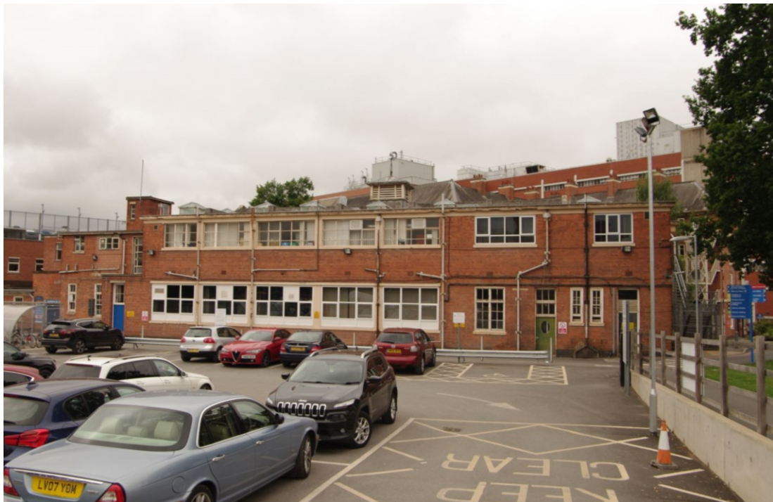
Figure 19 East facing elevation Looking south-west. Note the variety of window styles
