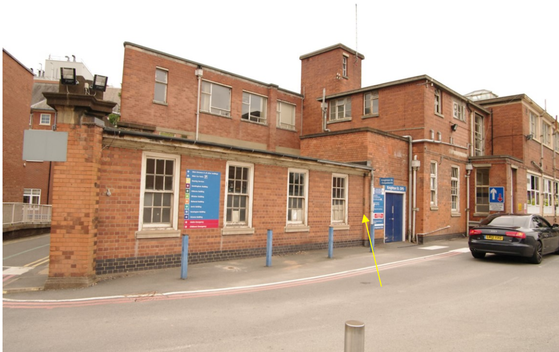
Figure 17 South-east corner of east facing elevation Looking north-east. Yellow arrow points to obscured sign – see Figure 18
