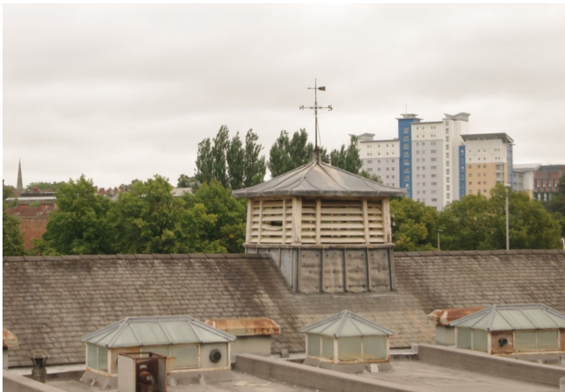
Figure 11 Close-up of vent and weather vane Looking east
