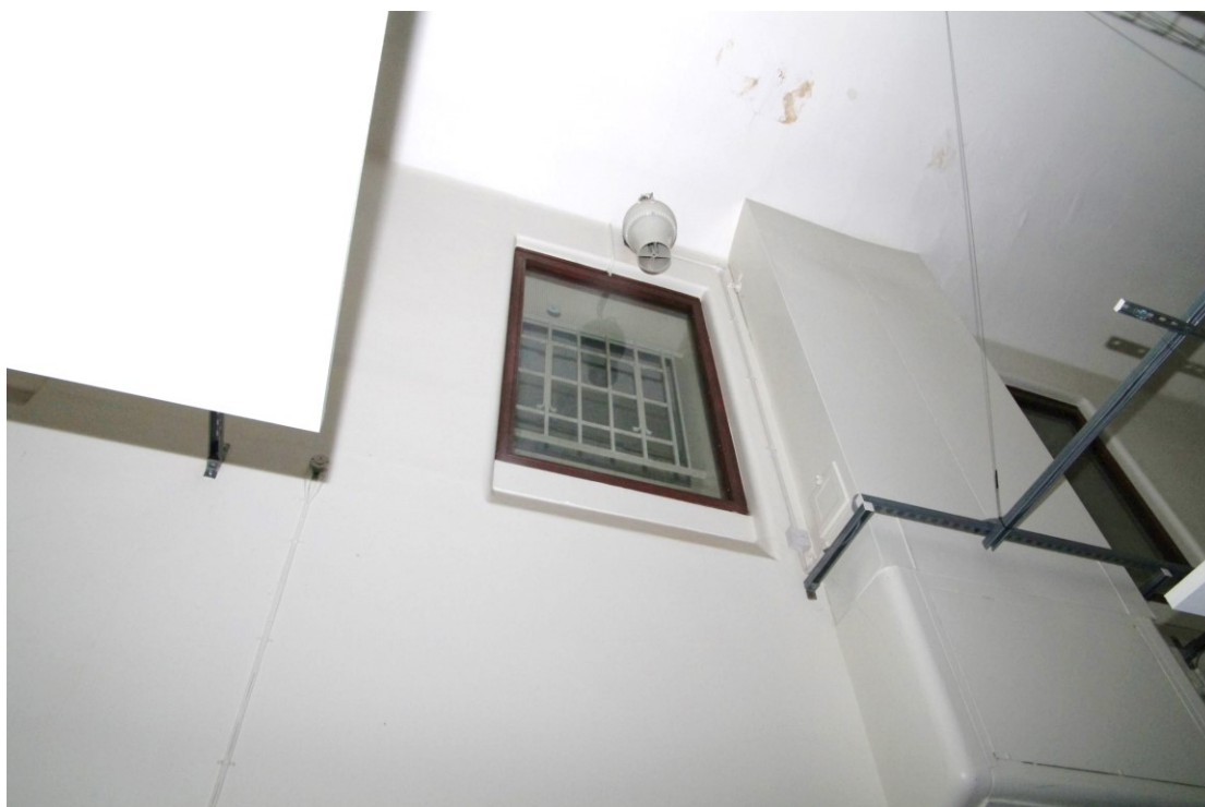
Figure 29 Former external window in central hall Modern glazing unit is in front of the earlier iron grille
