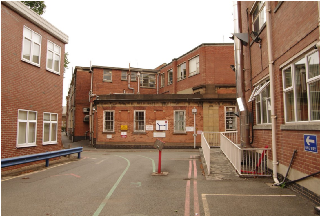
Figure 14 Western end of south facing elevation Looking north. The line of Knighton Street ran from left to right in front of the building
