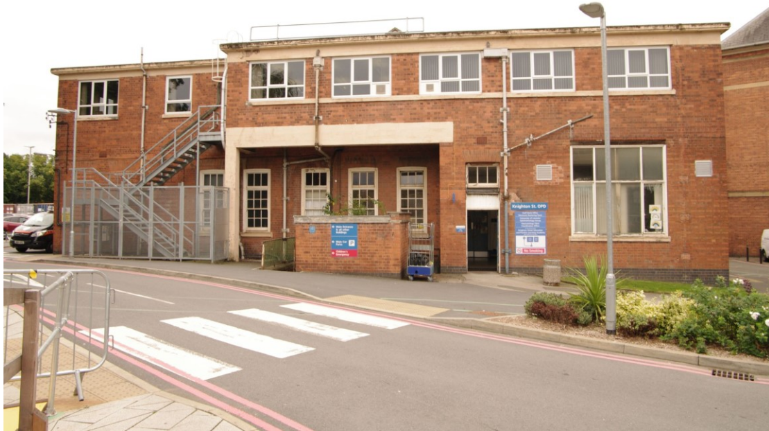
Figure 20 North facing elevation Looking south. Note how the later first floor steps out beyond the original wall line
