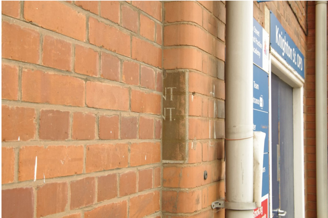
Figure 18 Partially obscured sign on east facing elevation This appears to have been to the side of an earlier south facing entrance but was later built-over
