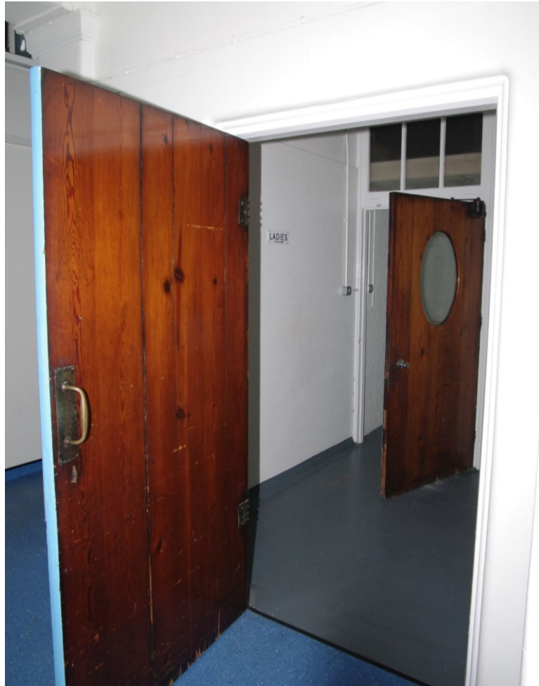
Figure 23 Entrance area: female toilet doors and fittings
