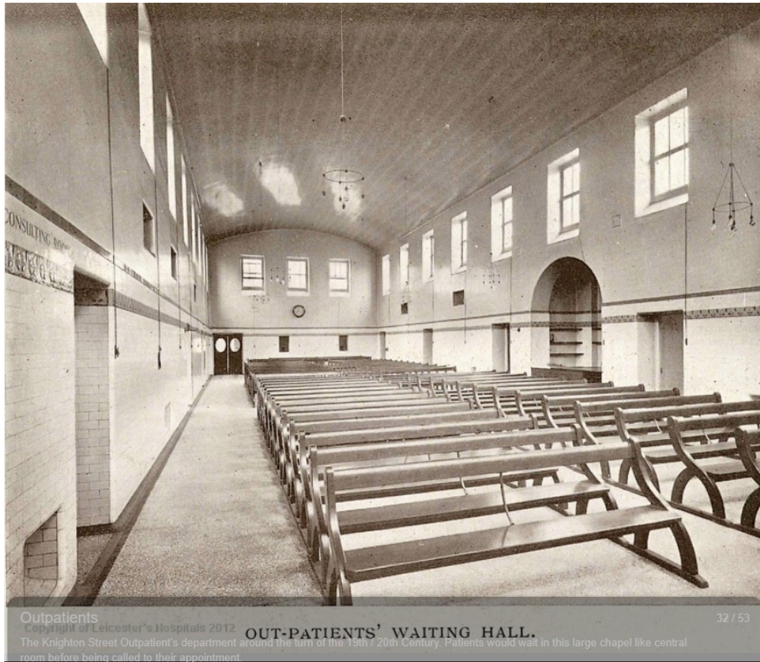
Figure 27 Central hall as first built
