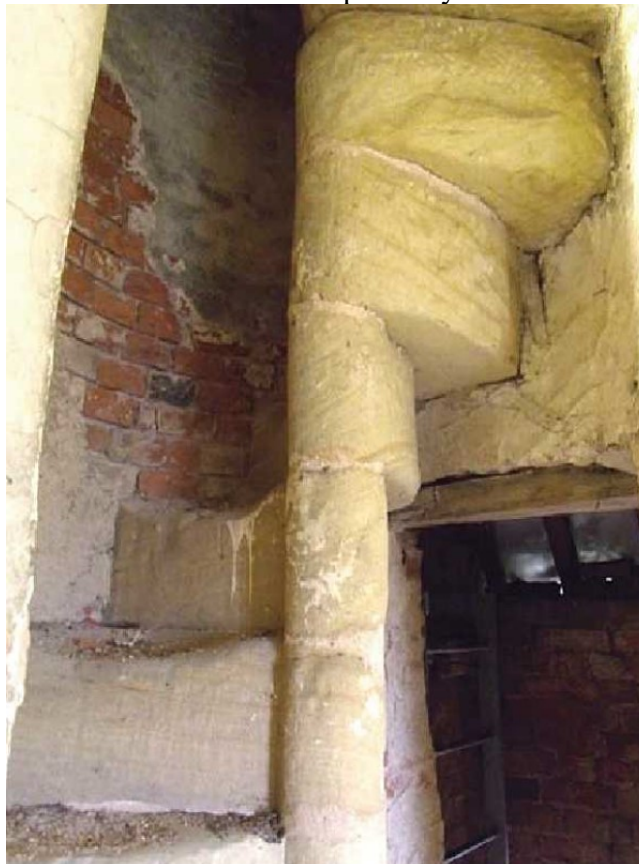
Figure 16 Remnant of spiral stairs within the main tower Note the top of the metal ladder on the right which is seen in Fig. 15 Picture credit: P R Associates, Design and Access Statement 2019
