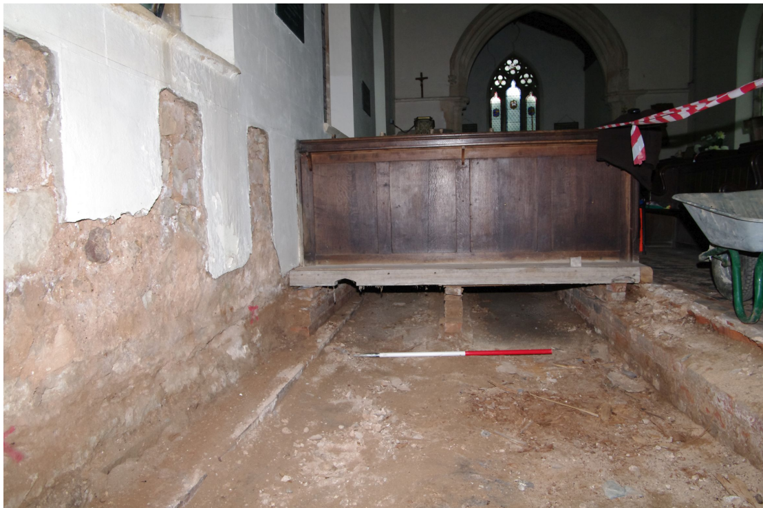
Figure 38 Supporting brickwork beneath pew platforms Looking east at pews to north of aisle. 1m scale
