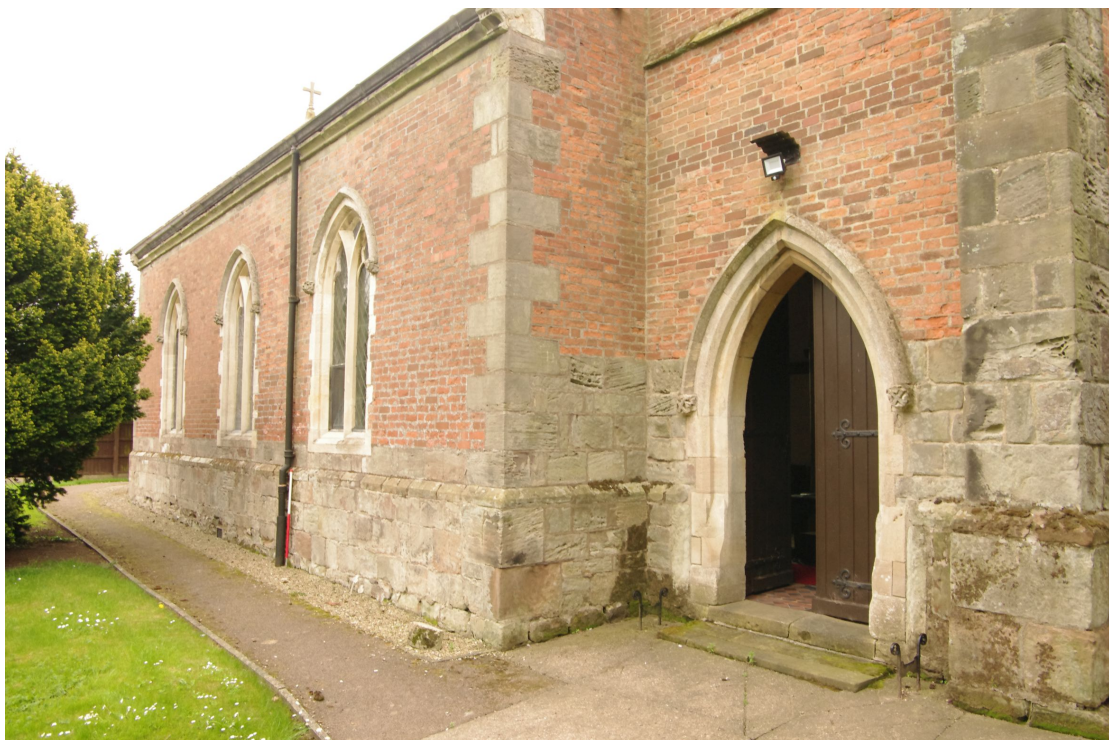
Figure 8 Detail of south facing tower door Looking south-east. 1m scale
