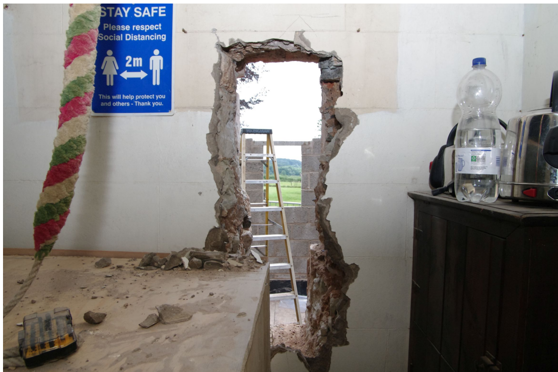
Figure 49 Slot through tower wall Looking south from the inside
