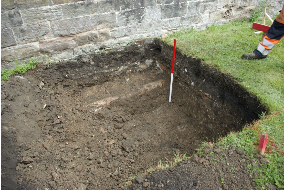
Figure 26 Drain alongside the church being exposed Looking north-east. 1m scale
