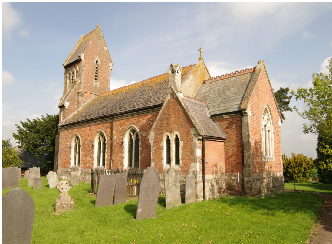
Figure 9 General view of south side of church Looking north-west. 1m scale. The new extension will be located to the far left of the building
