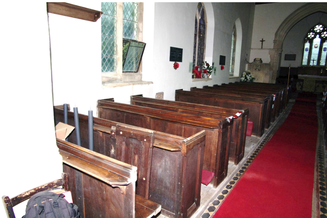
Figure 22 Pew detail on north side of nave Looking north-east. The first four pews and the platform will be removed
