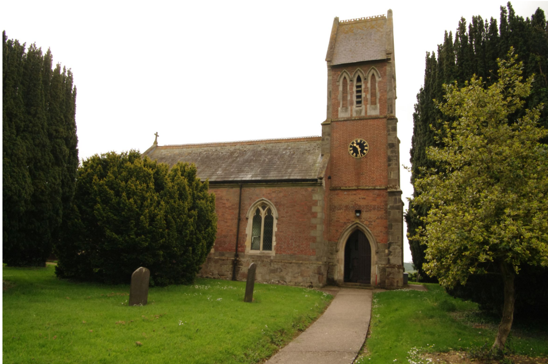
Figure 7 North facing elevation of tower A new access ramp will be added to cross the raised step into the doorway. No significant excavations will be involved for this work
