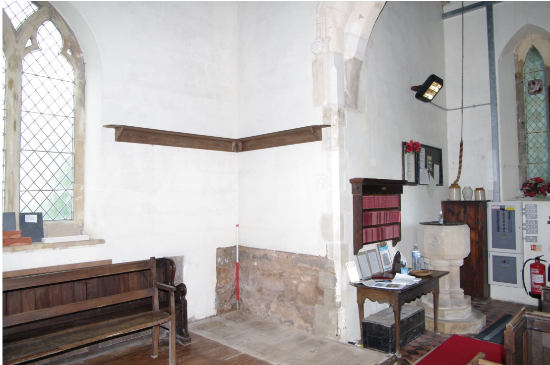
Figure 19 South-west corner of nave
