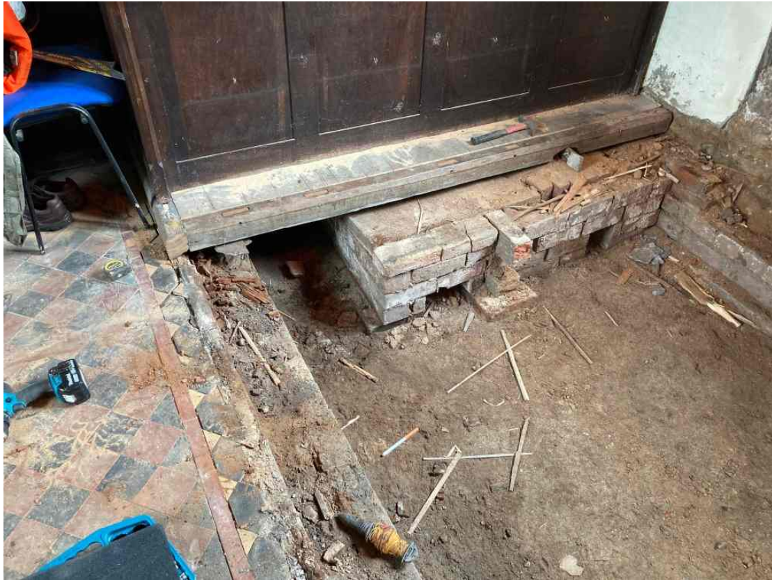
Figure 37 Exposed base for stove against south wall seen beneath pews Most of this plinth was left in-situ. Picture taken by Ackroyds
