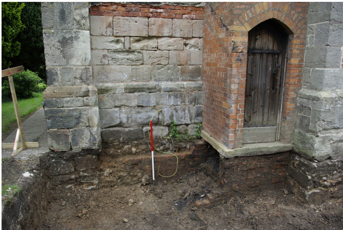
Figure 30 Exposed tower base Looking north. 1m scale
