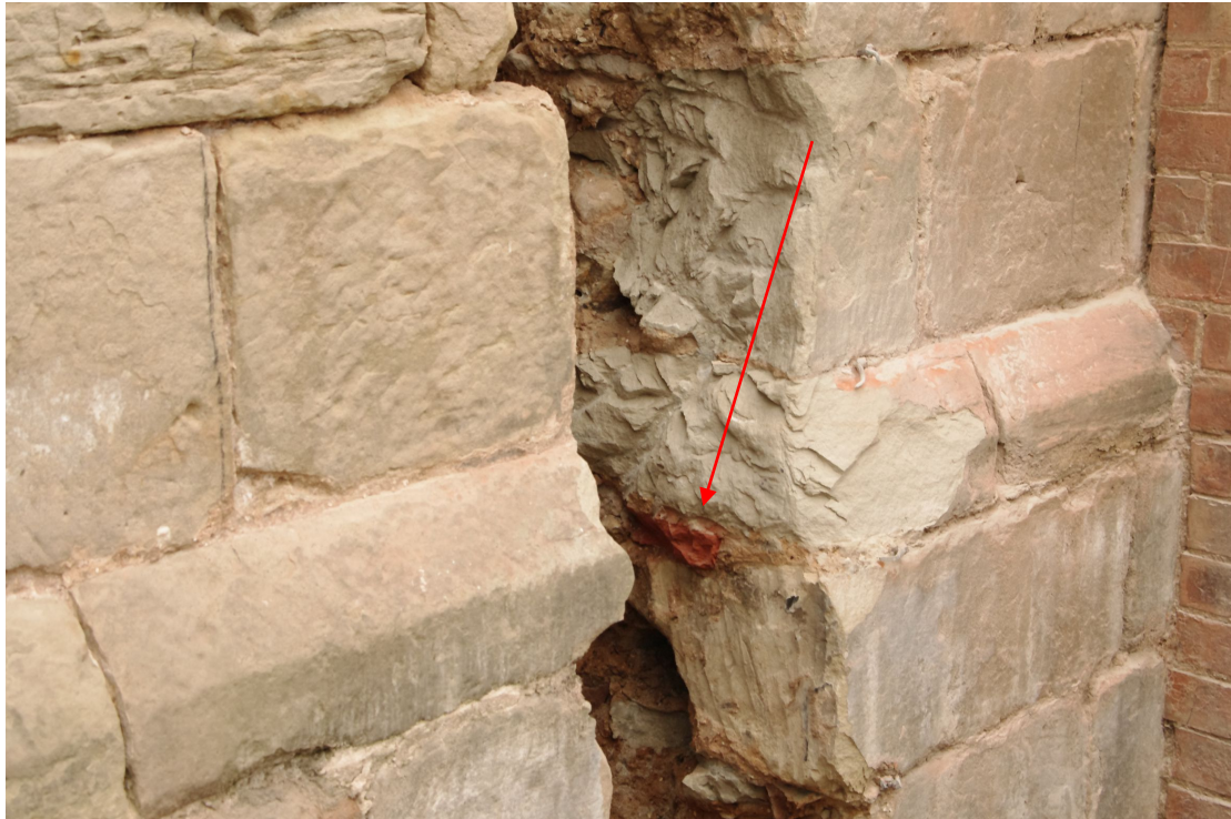
Figure 52 Fragment of brick within the stone matrix of the tower wall The red arrow points towards the brick fragment
