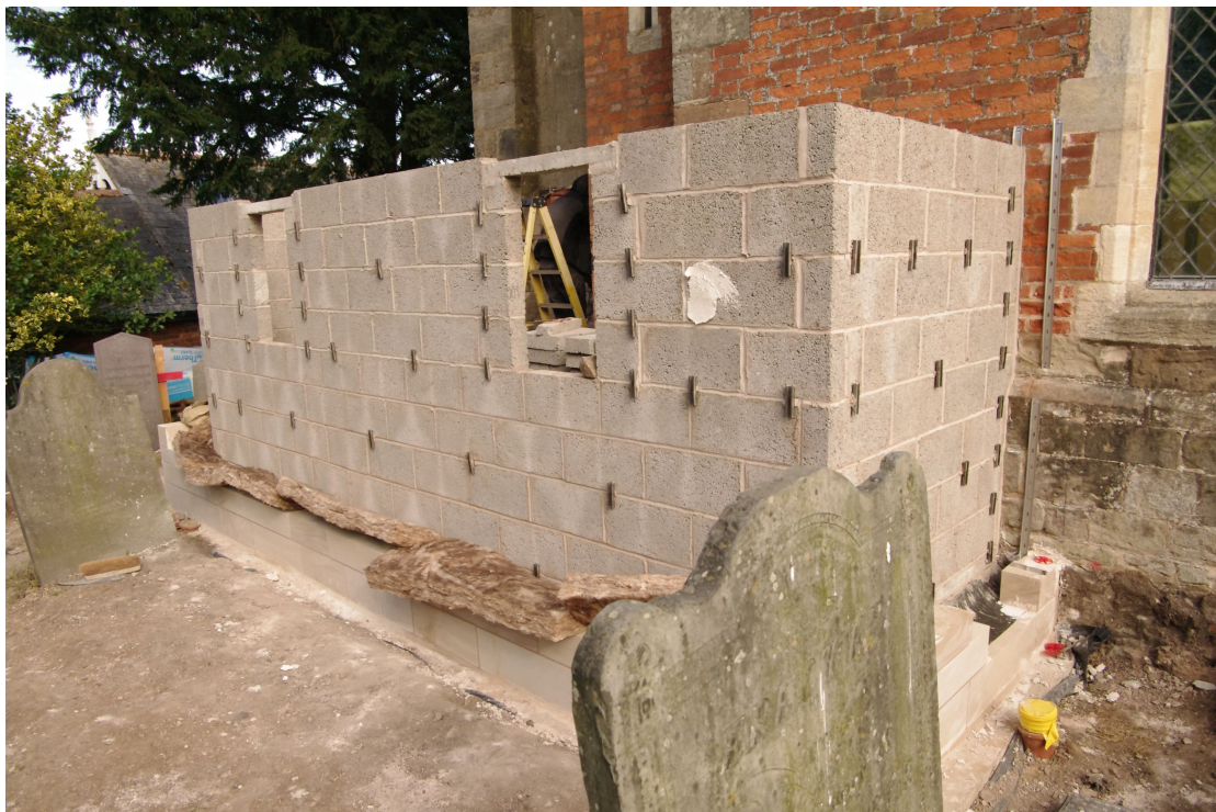
Figure 53 Partially complete extension Looking north-west
