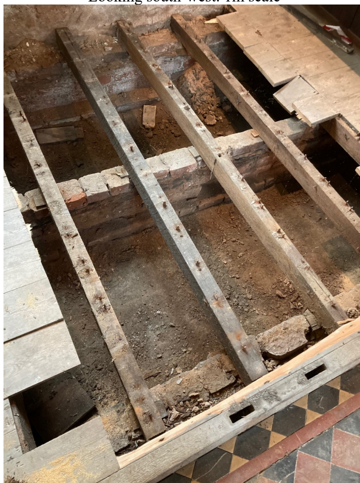
Figure 36 Pew platform being removed Picture taken by Ackroyds
