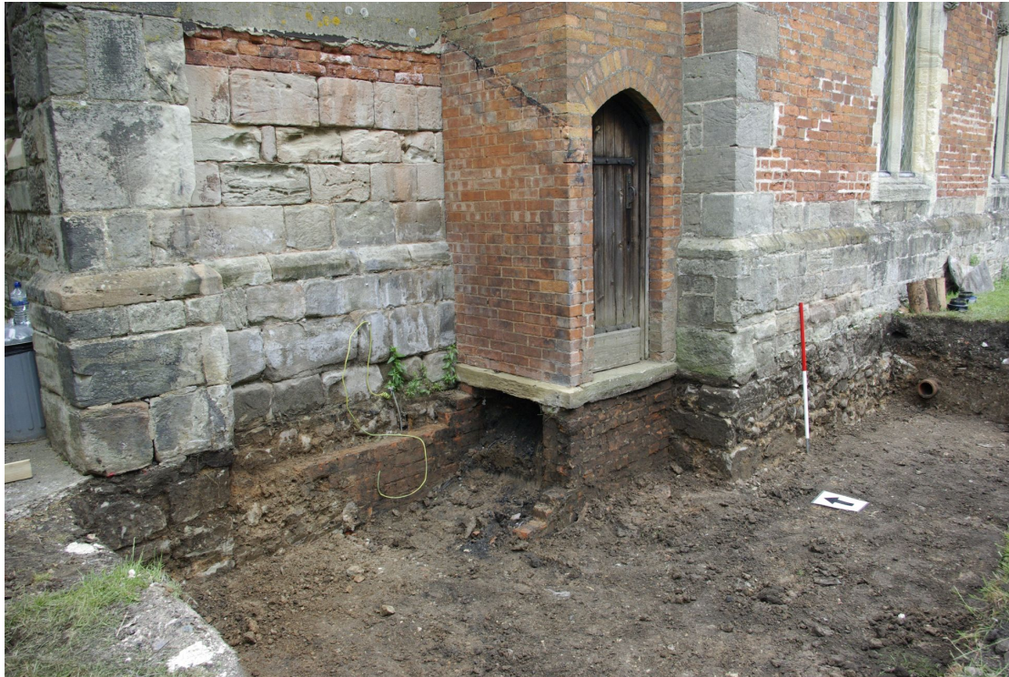
Figure 29 Exposed base of belfry access tower Looking north-east. 1m scale
