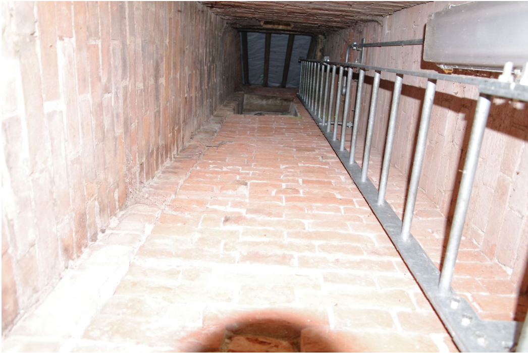
Figure 15 View up to the clock chamber and belfry access tower Looking north. The brickwork in the centre of the picture is part of the tower buttress. Note the infill of brick and later added wall on left. This indicates that the original tower access was within the main body of the tower – see Nichols illustration Fig. 3 and Fig. 16 below. This later access is probably from the 1867 remodelling
