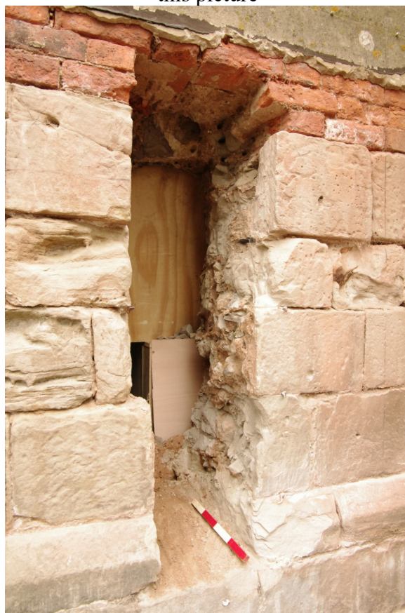
Figure 47 Slot through tower wall Looking north-east from outside. 0.4m scale
