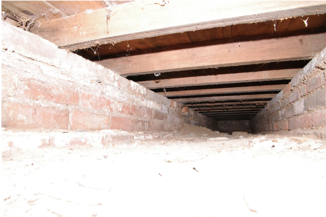
Figure 39 View beneath pew platforms Looking east
