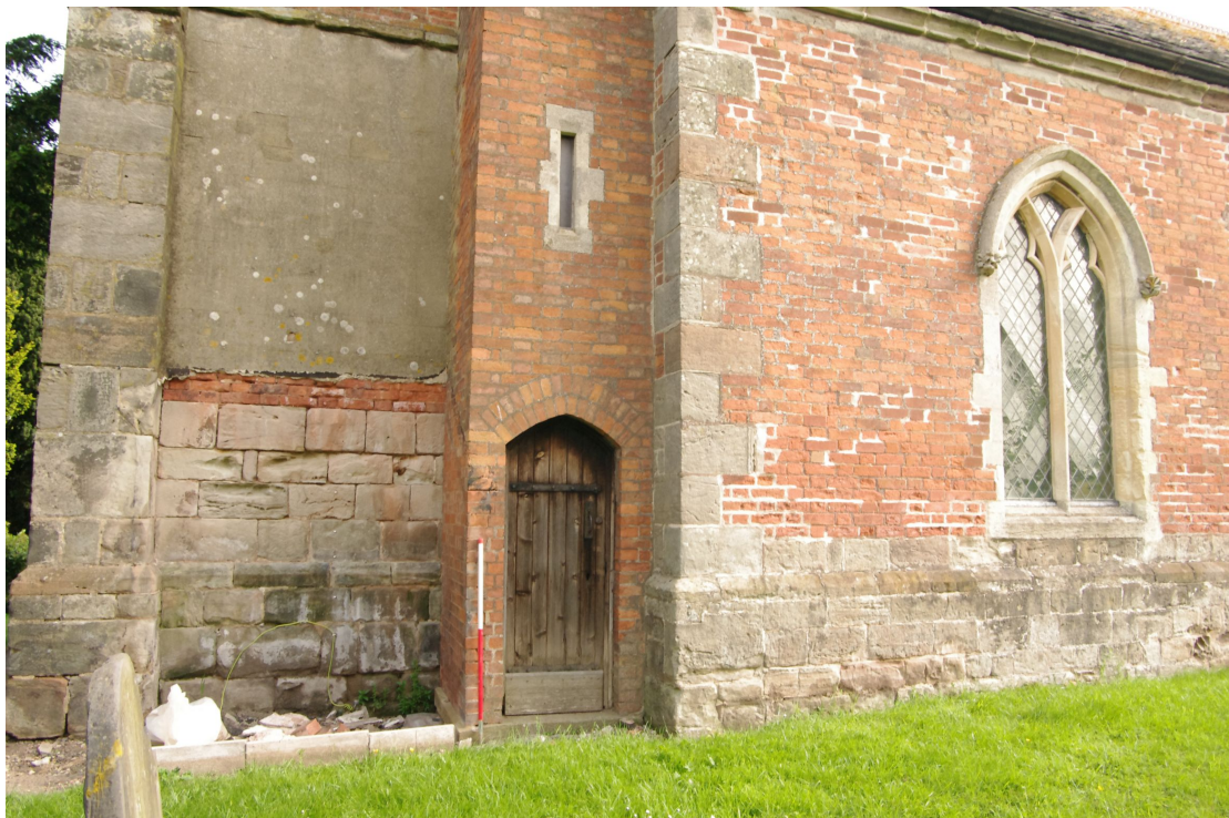
Figure 12 Location of proposed extension Looking north-east. 1m scale. Note the marks left by the demolished lean-to shed which had a roofline following the three courses of brick between the render and the stonework on the tower wall. The lean-to extended out as far as the brick-built clock and belfry access tower
