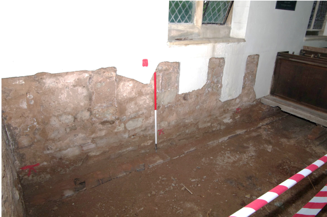
Figure 41 Exposed stonework on north wall Looking north-east. 1m scale
