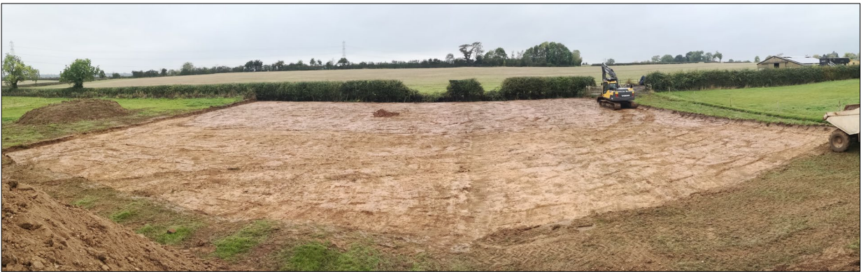
Figure 9: Cont'd, after stripping, looking west.
