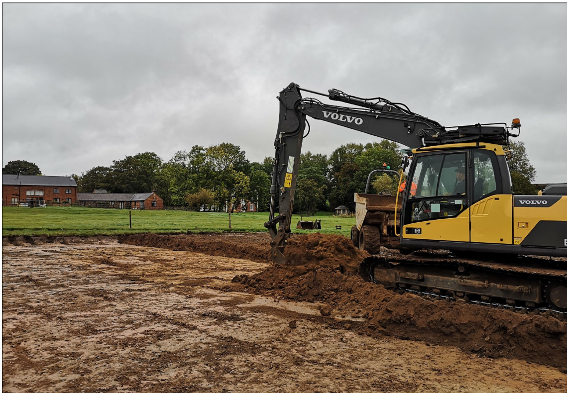
Figure 7: Soil strip, looking north-east towards The Manor
