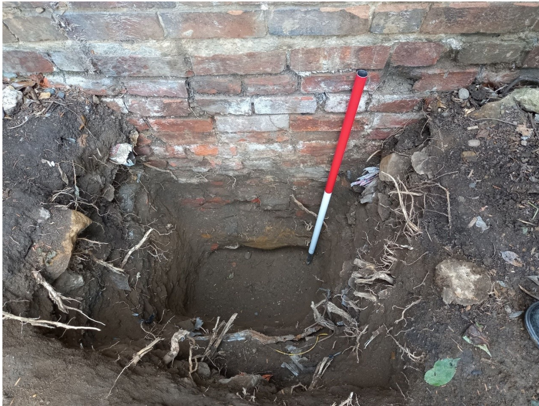
Figure 9 Re-excavated Test-pit 1 Looking north. 1m scale
