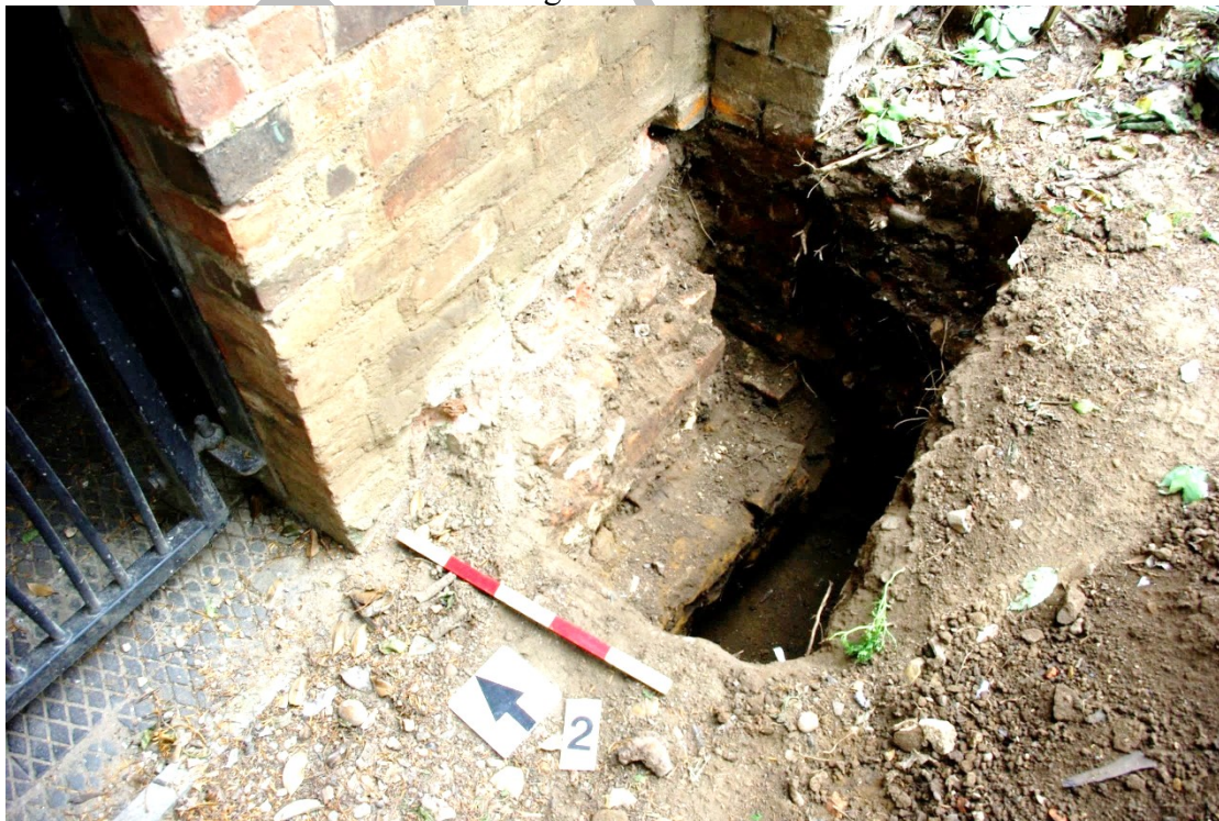
Figure 10 Re-excavated Test-pit 2 Looking north-east. 0.5m scale
