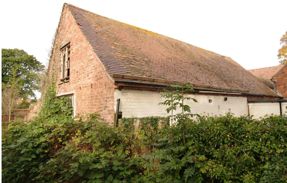
Figure 49 South barn, south facing gable end and east elevation
