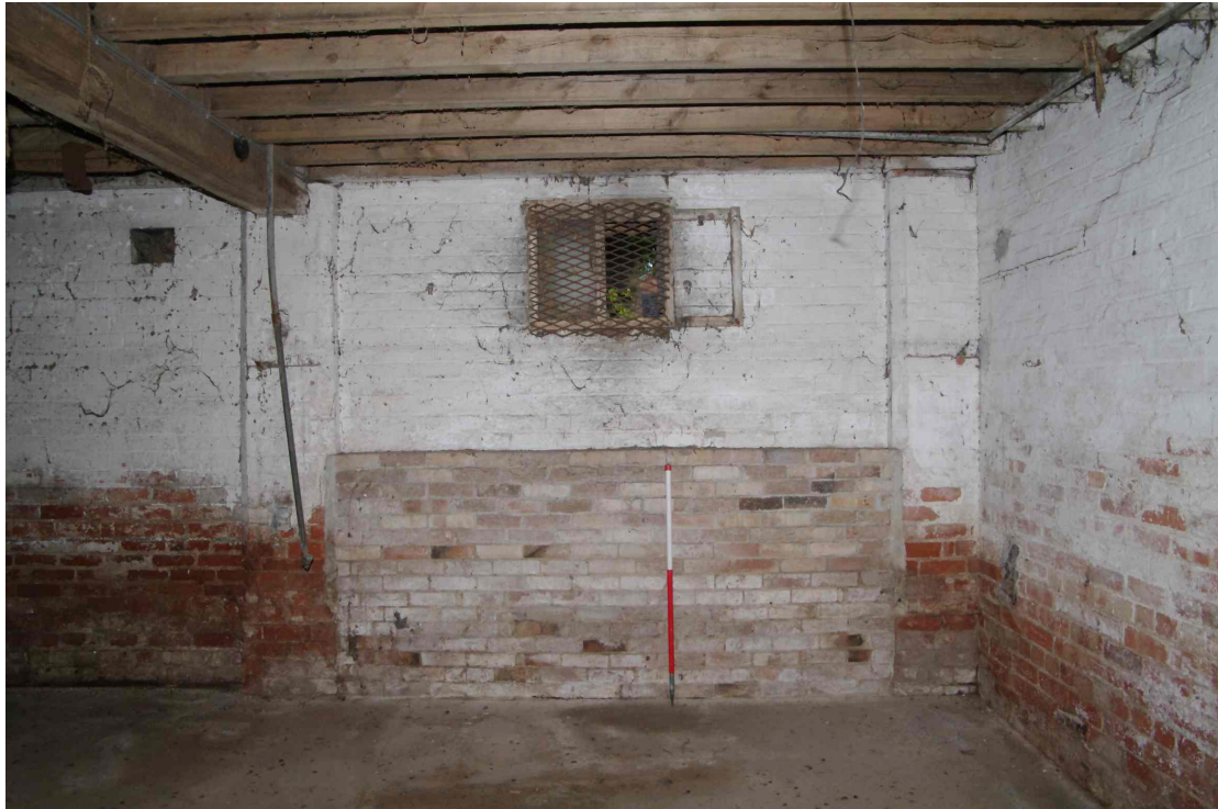
Figure 31 North barn, ground floor. North wall Looking north at window shown in Figure 18. 1m scale The brickwork masks the outer timber frame
