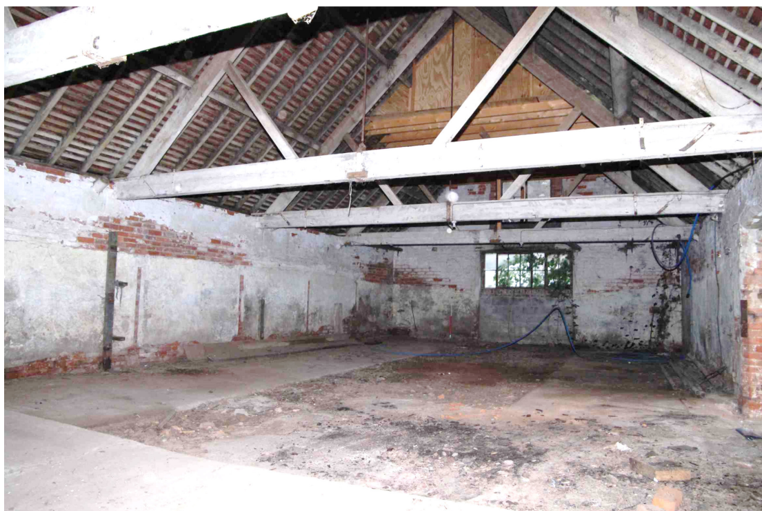
Figure 50 South barn, general view
