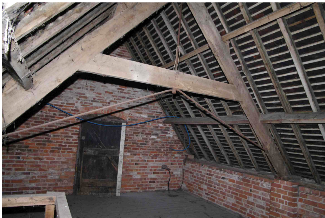
Figure 33 North barn, first floor Looking north-west towards hayloft door
