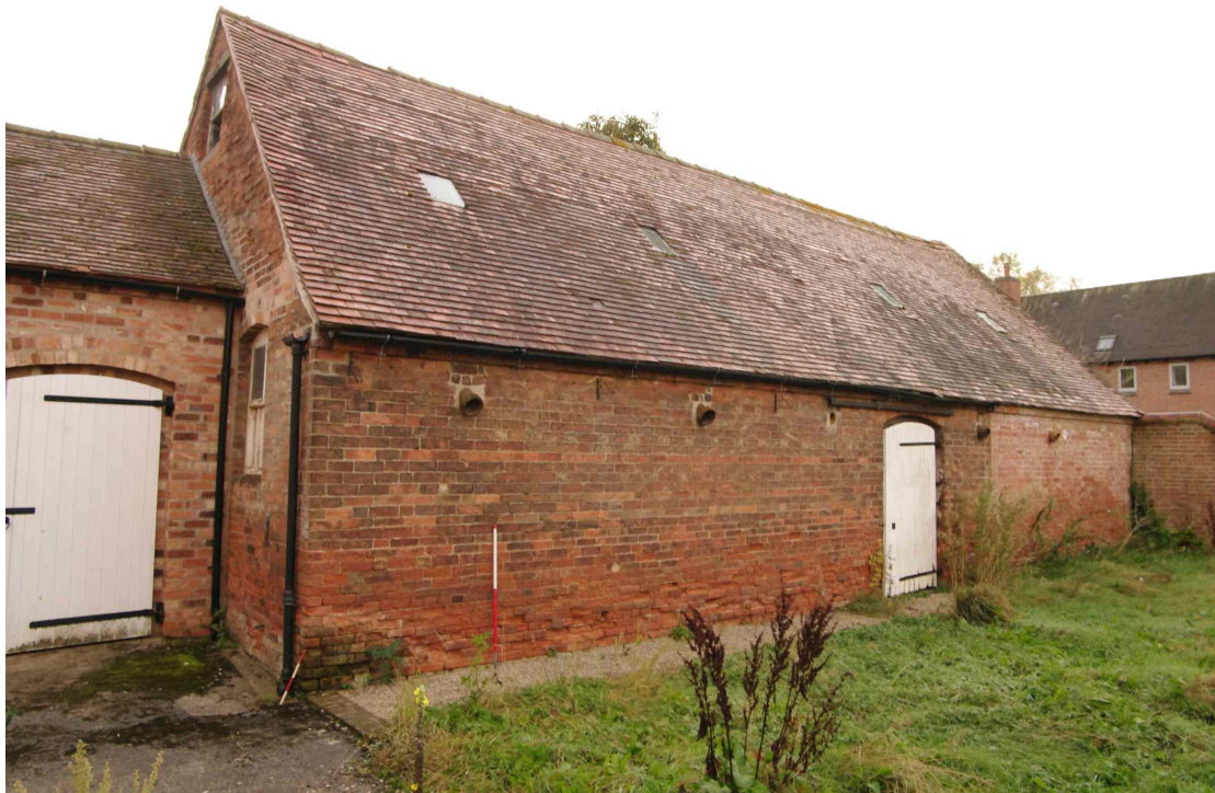
Figure 42 West facing elevation of the south barn
