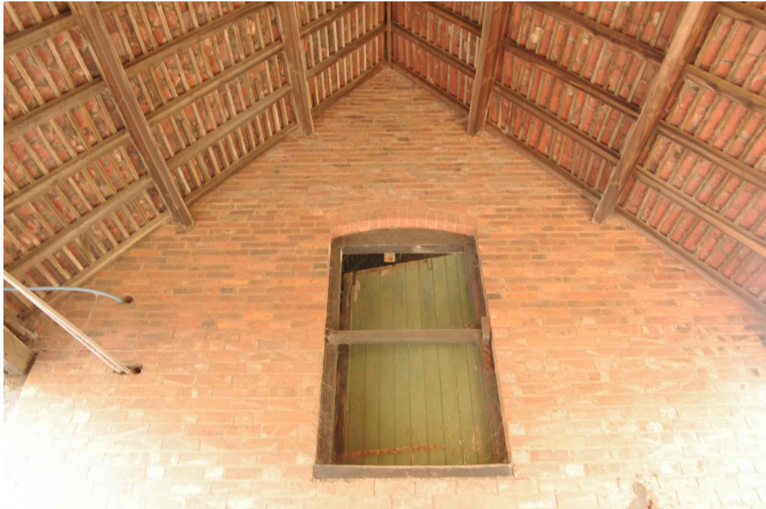
Figure 21 Hayloft door on west facing gable under covered entrance Looking east
