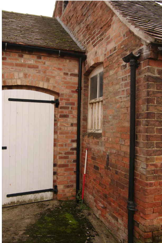
Figure 37 Junction of middle and south barns Looking south-east. 1m scale
