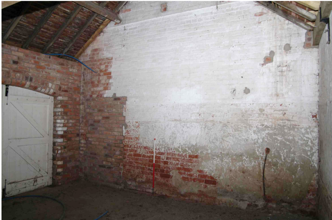
Figure 39 Middle barn north end wall
