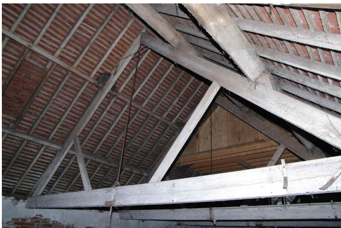
Figure 52 South barn roof structure
