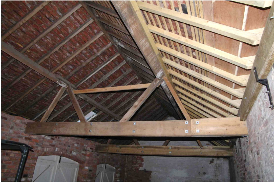
Figure 41 Middle barn roof structure
