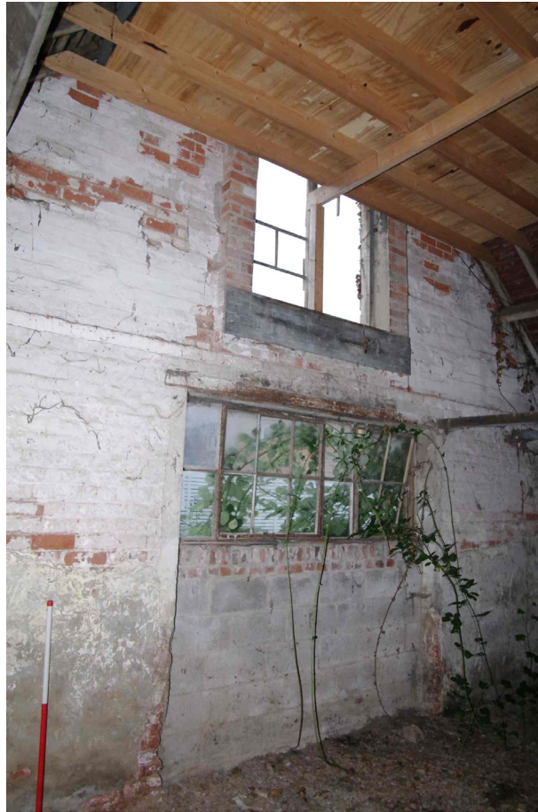
Figure 53 South barn, southern end wall
