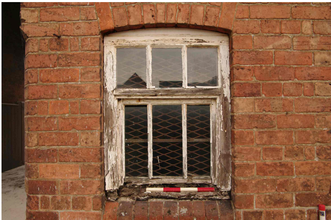
Figure 24 Window on south facing elevation of northern barn Looking north. 0.4m scale. Note chamfered brick corner on left
