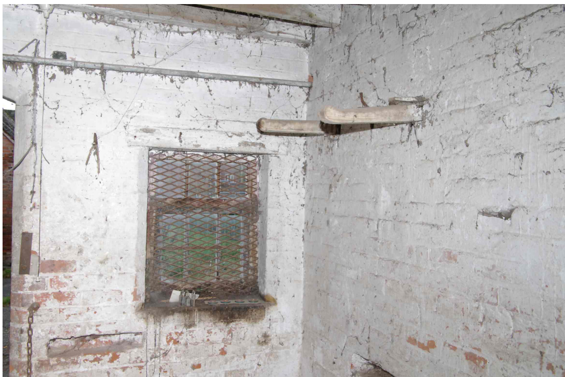
Figure 30 North barn, ground floor. Window detail Looking south-west. Note saddle trees
