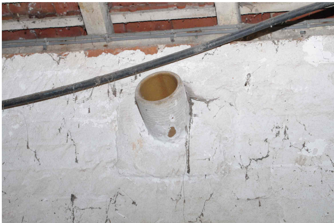
Figure 55 South barn, internal vent detail See also Figure 44
