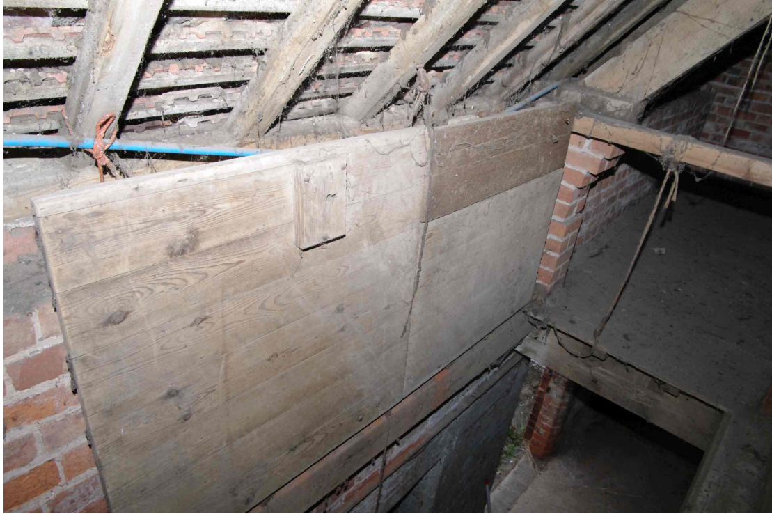
Figure 35 North barn first floor, stair hatch Looking south-west. The hatch is made from a re-used door which retains its wooden lock case
