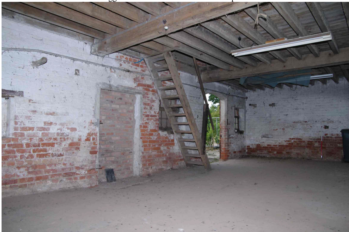
Figure 28 General view of north barn ground floor Looking south-west
