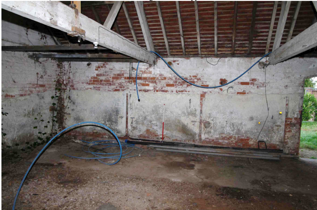
Figure 54 South barn, west wall
