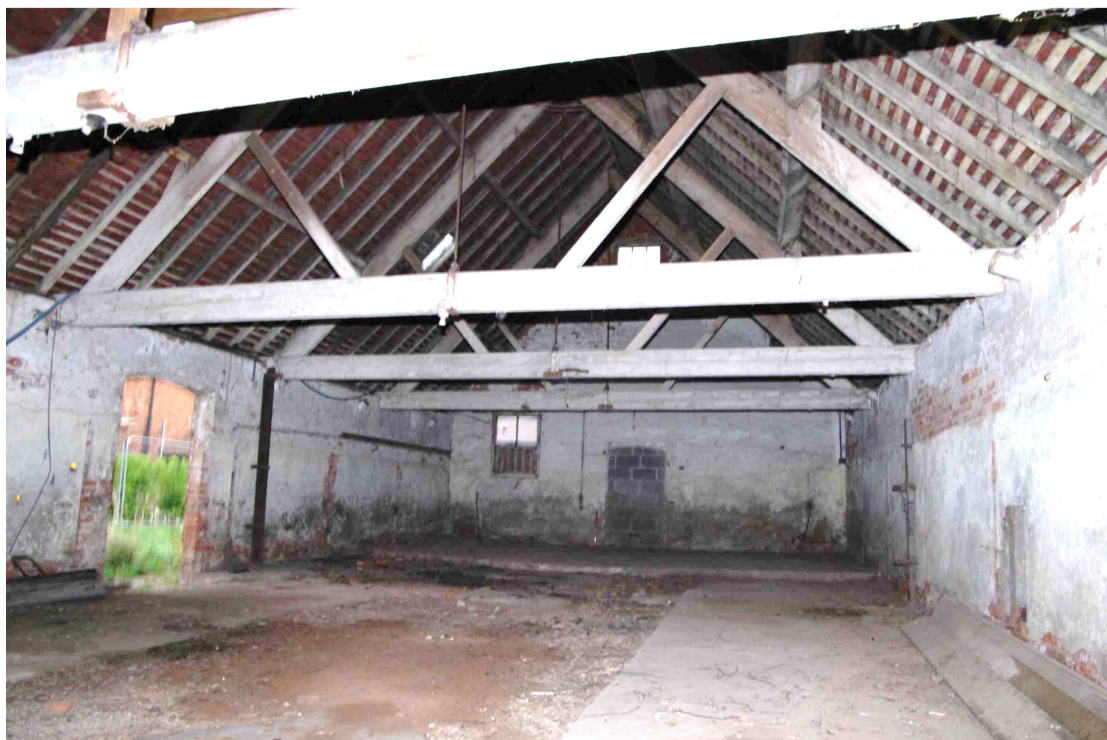
Figure 51 South barn, general view
