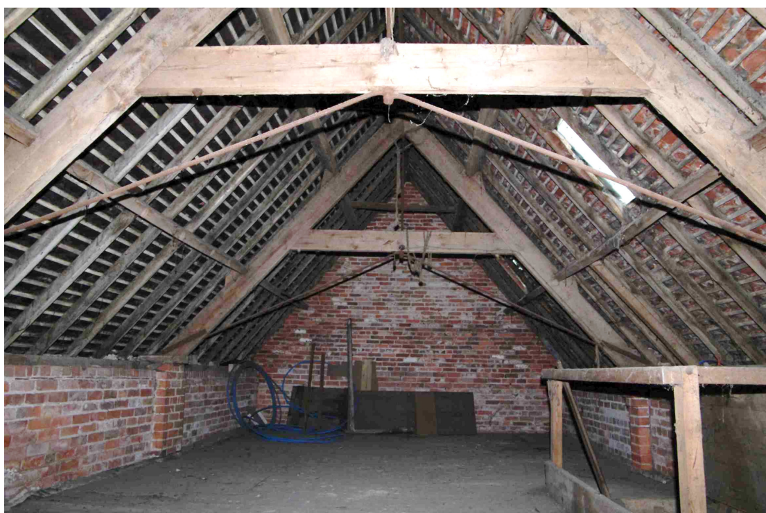
Figure 34 North barn, first floor Looking east. The bolted roof structure suggests a mid to late 19th century date
