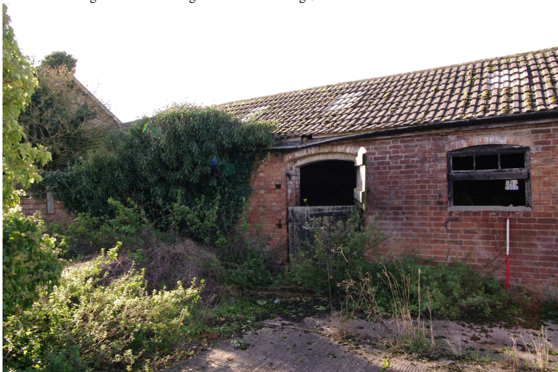
Figure 36 Building 5 north-east facing elevation. Southern end Looking south-east. 1m scale
