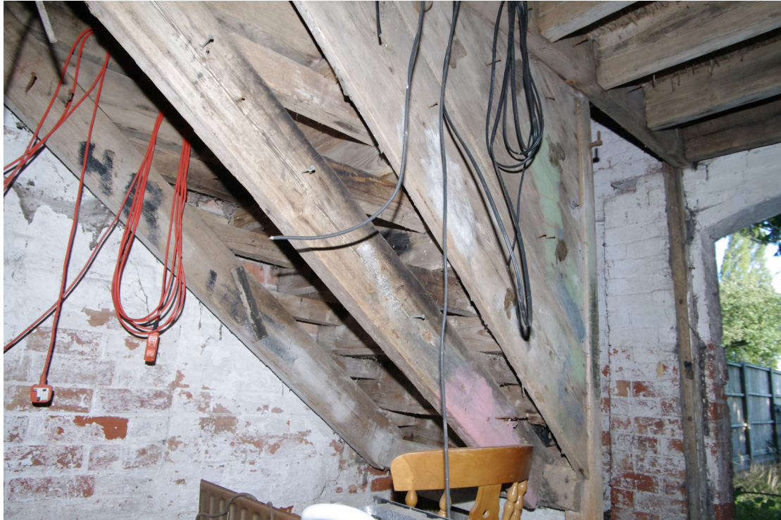
Figure 80 Building 7. Room 2 stair detail Looking north-east
