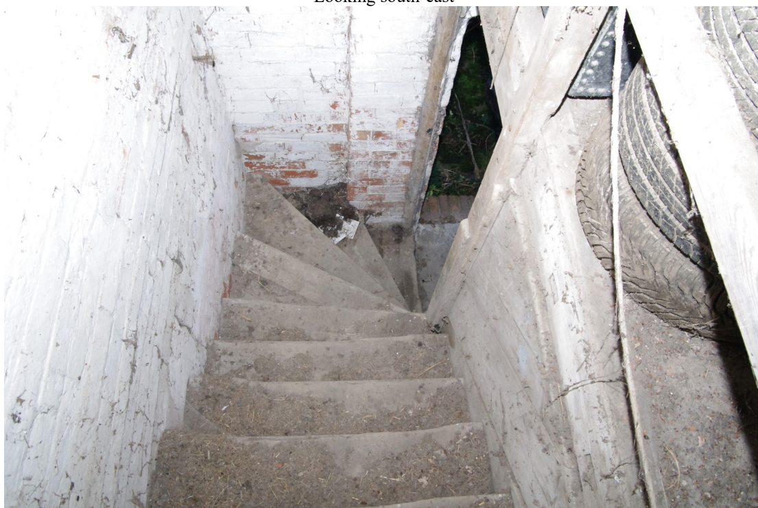
Figure 93 Building 7. Room 10 Looking south-west down the stairs to Room 2
