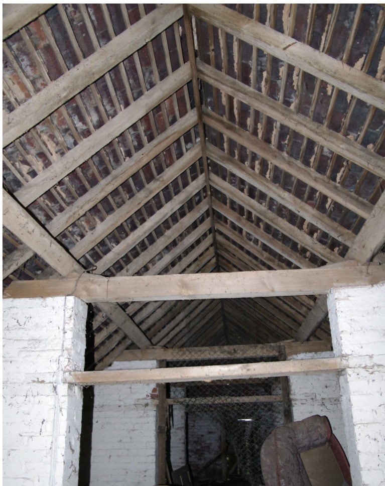
Figure 92 Building 7. Room 10 roof structure Looking south-east
