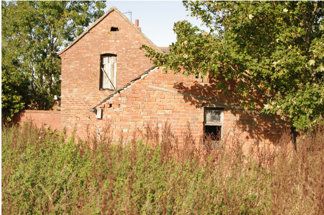
Figure 72 Building 7 south-east facing gable ends Looking north-west
