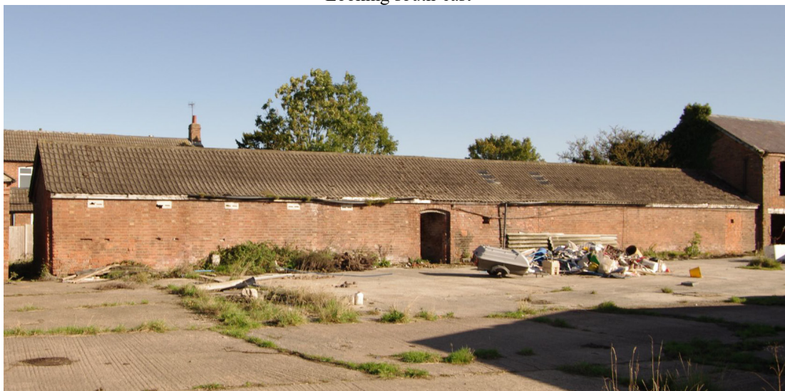
Figure 38 Building 5 south-west facing elevation Looking east
