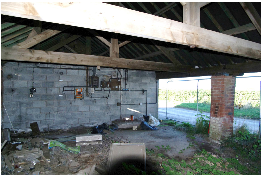
Figure 15 Building 1, internal view Looking north-west towards modern blockwork
