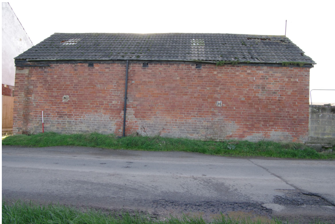
Figure 27 Building 4 north-west facing elevation
