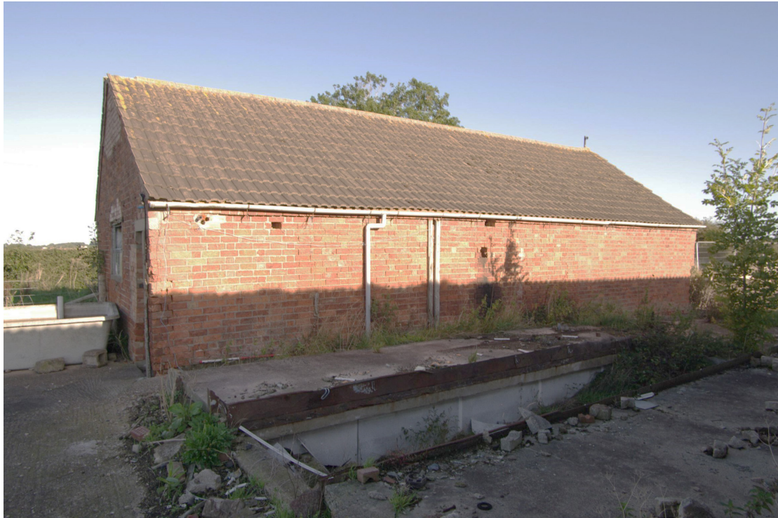
Figure 13 Building 1 south-east facing elevation Looking north.
