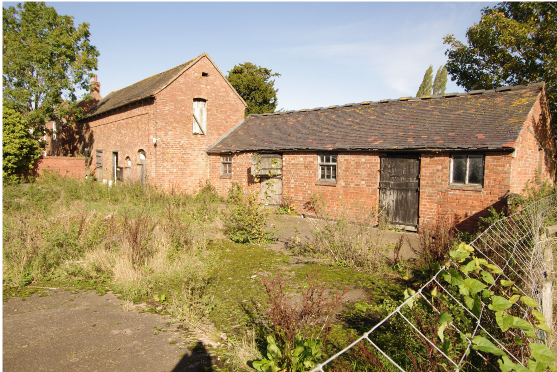
Figure 66 Building 7 south-west facing elevation Looking north-east
