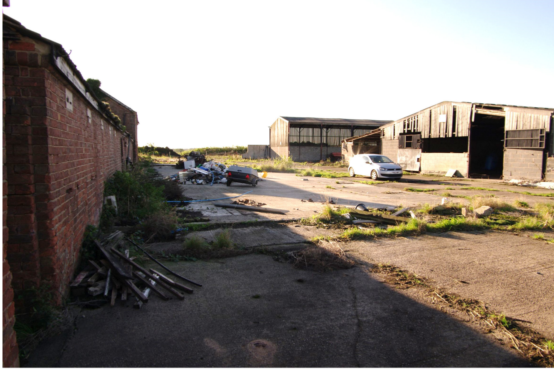
Figure 19 Buildings 2 and 3 Looking south. Building 2 on extreme right, Building 5 on left
