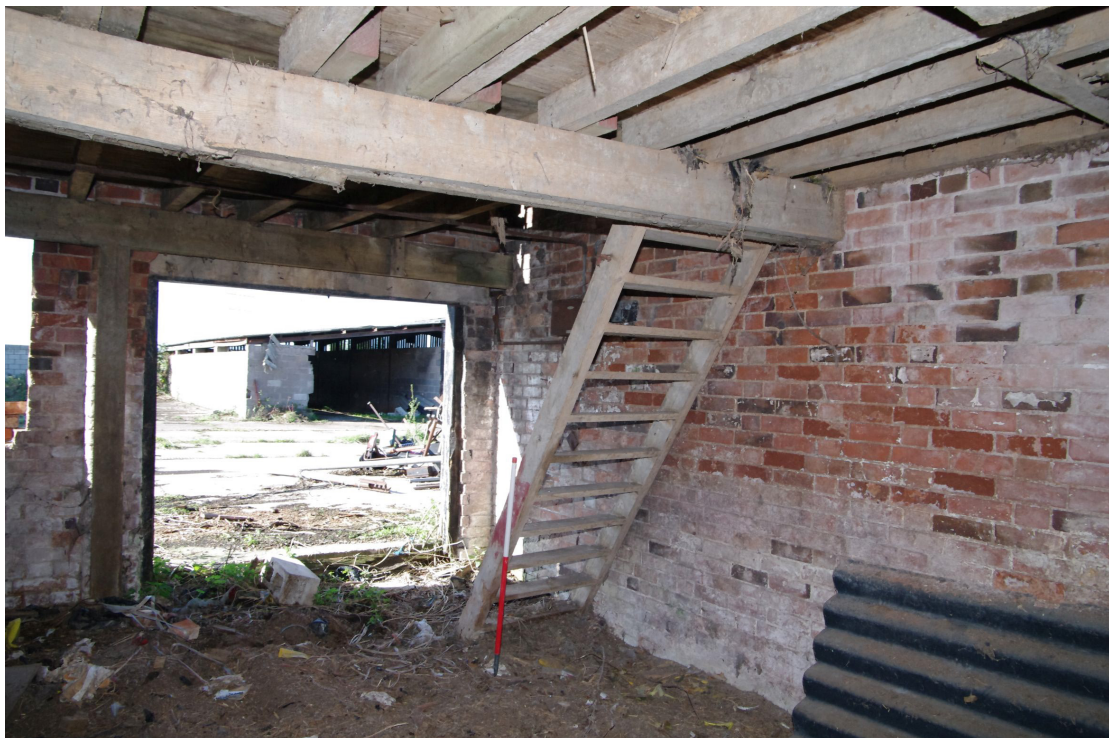
Figure 56 Building 6. Ground floor room on north side Looking west. 1m scale
