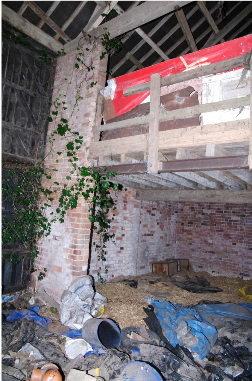
Figure 63 Building 6 ground floor area beneath mezzanine floor to south Looking south-east
