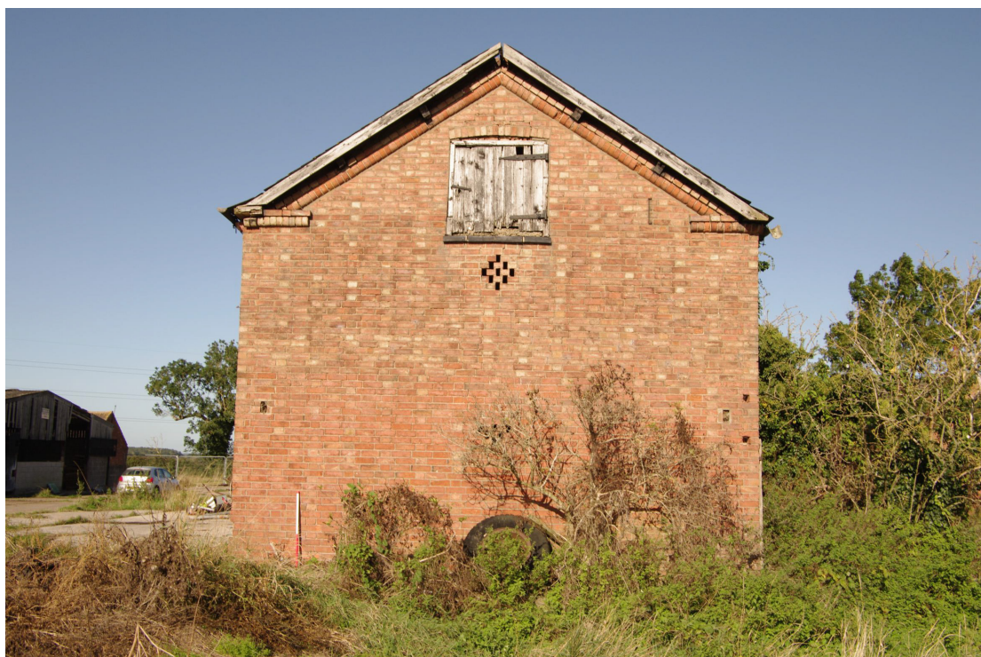
Figure 54 Building 6 south-east facing gable end Looking north-west. 1m scale
