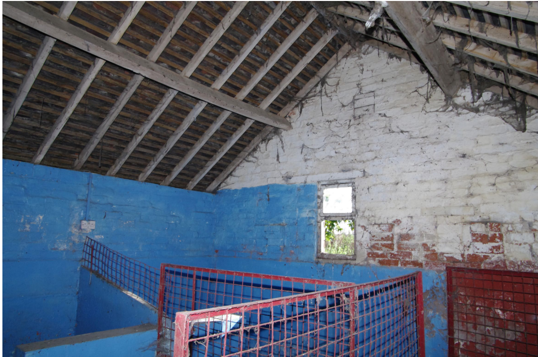
Figure 90 Building 7. Room 9 Looking south-east
