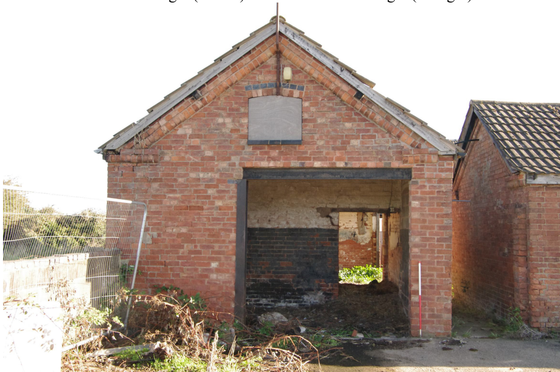
Figure 26 Building 4 south-west facing elevation Looking north-east. The large opening to the left of the 1m scale is modern and has a steel lintel
