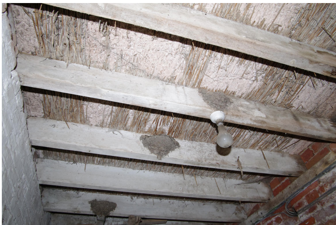
Figure 86 Building 7. Room 7 ceiling detail
