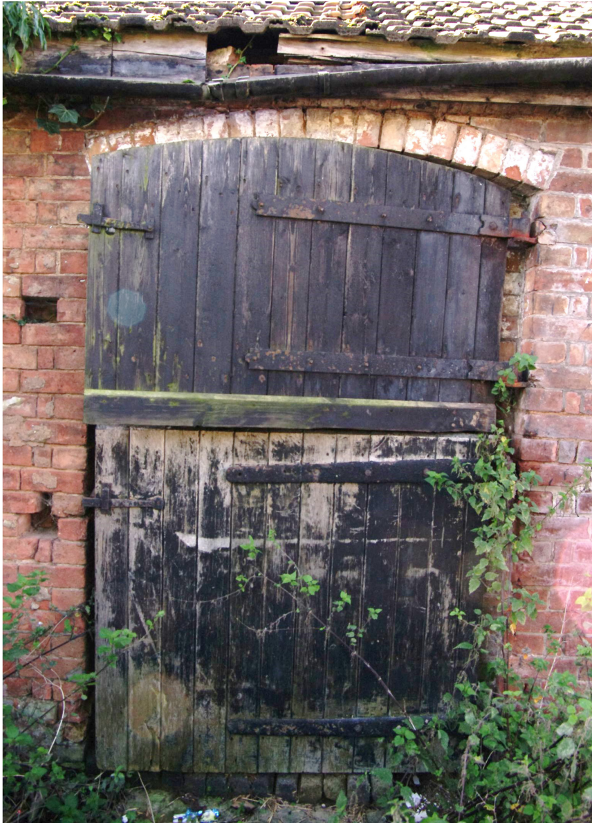
Figure 37 Building 5 north-east facing elevation. Door detail Looking south-east
