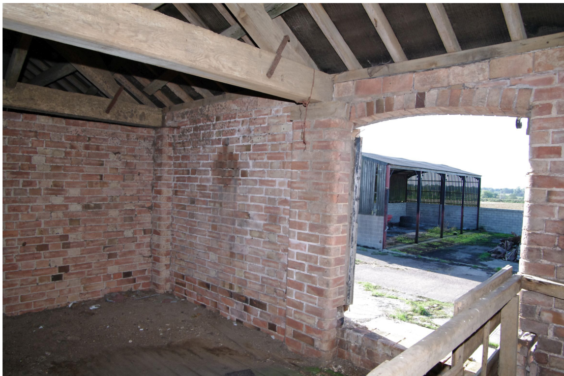
Figure 58 Building 6. First floor room on north side Looking south-west. Part of the wall on the left was open to the central area of the threshing barn but has been blocked with brickwork. Building 3 can be seen through the window
