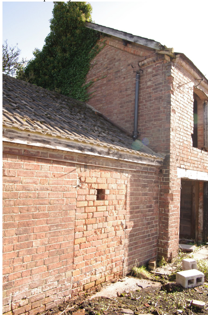
Figure 52 Building 6 north-west facing gable
