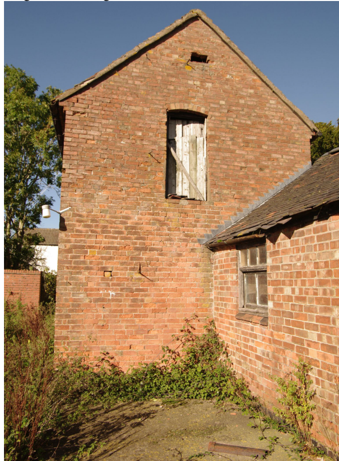
Figure 69 Building 7. South-east facing gable end of two storey range Looking north-west
