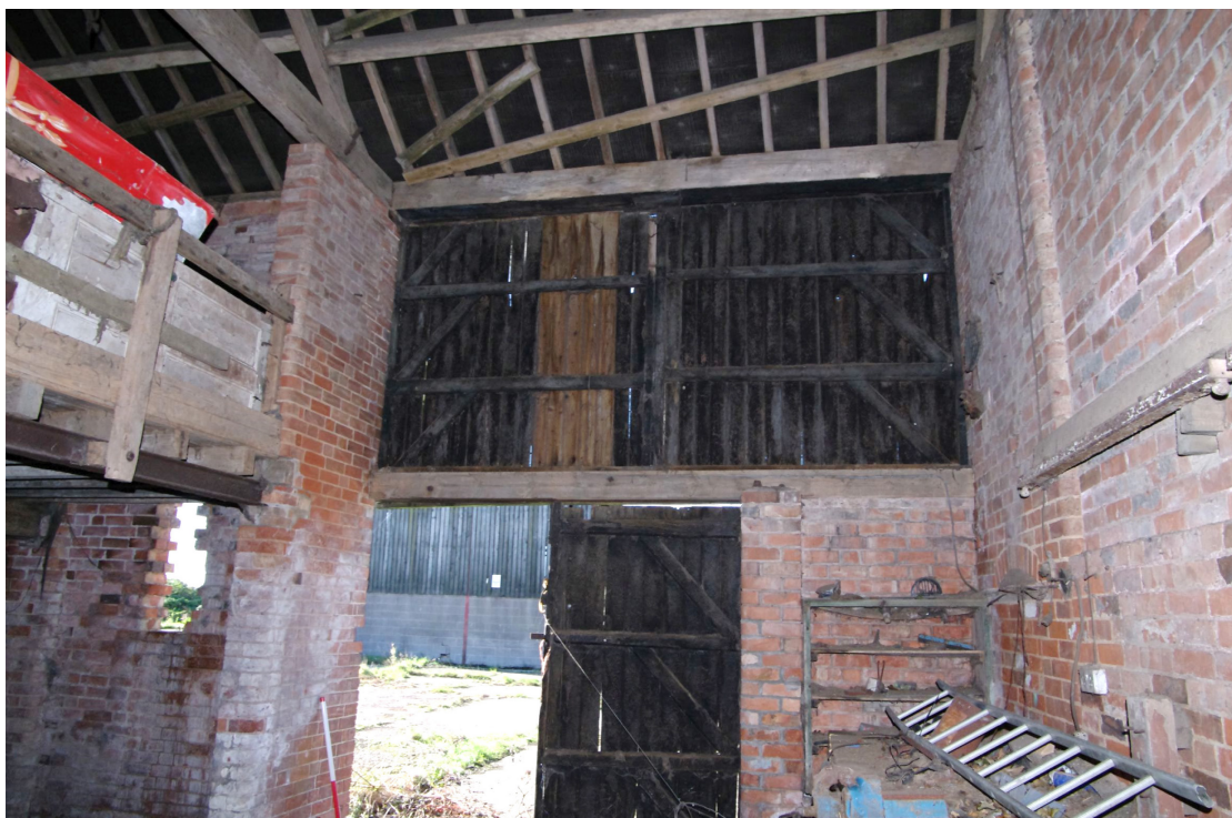
Figure 62 Building 6 central area and former full-height doorway Looking south-west
