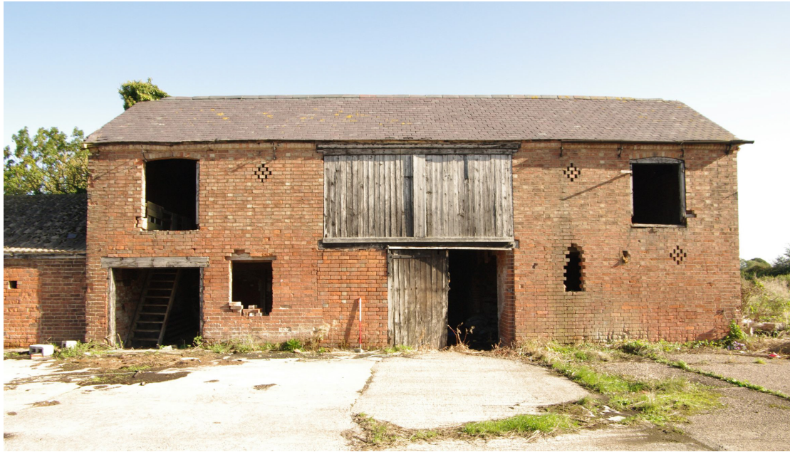
Figure 51 Building 6 south-west facing elevation
