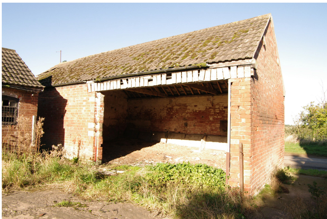
Figure 24 Building 4 south-east facing elevation and north-east gable end Looking north-west. The purlins extend beyond the gable end showing where they continued across to the farmhouse. Dadlington Lane to right
