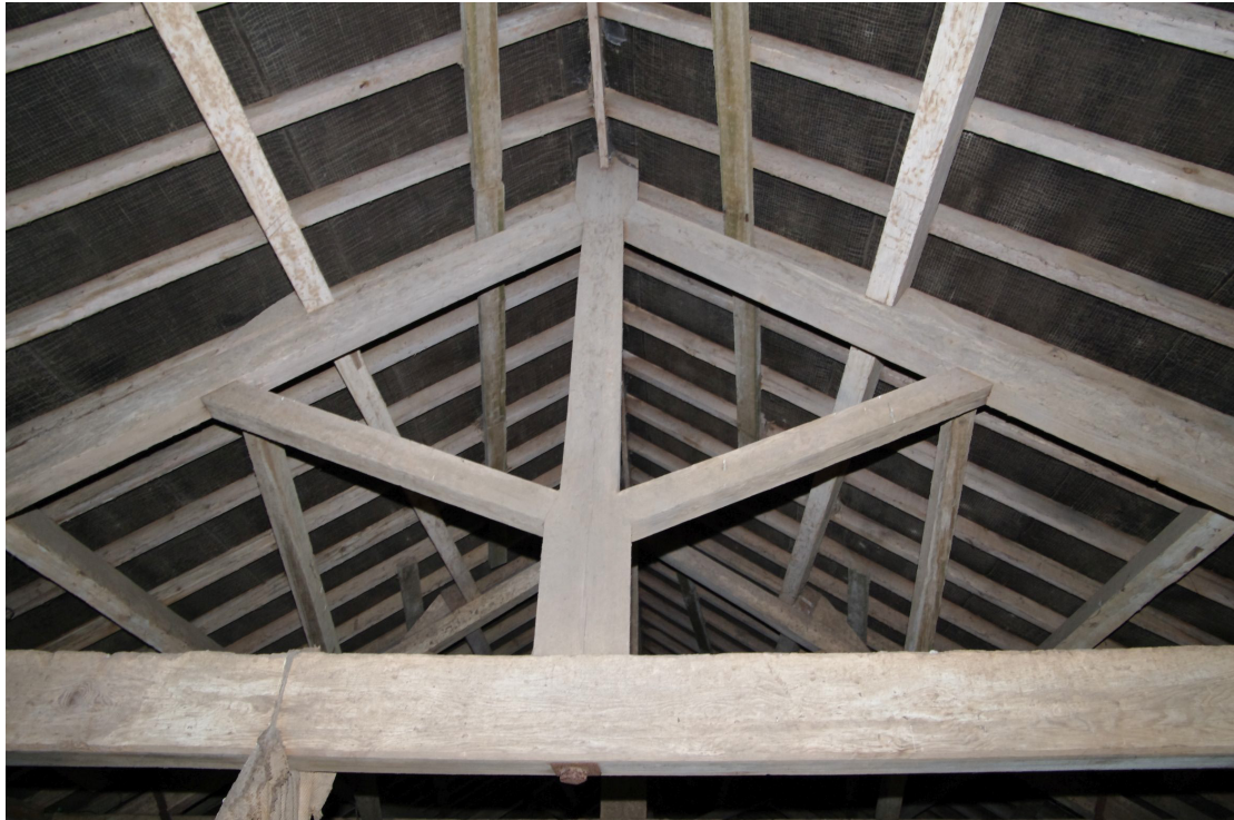
Figure 59 Building 6 roof structure Looking south-east from first floor room
