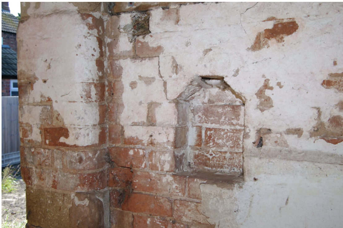
Figure 30 Lamp/candle niche in Building 4 Looking south-east. Main doorway to left
