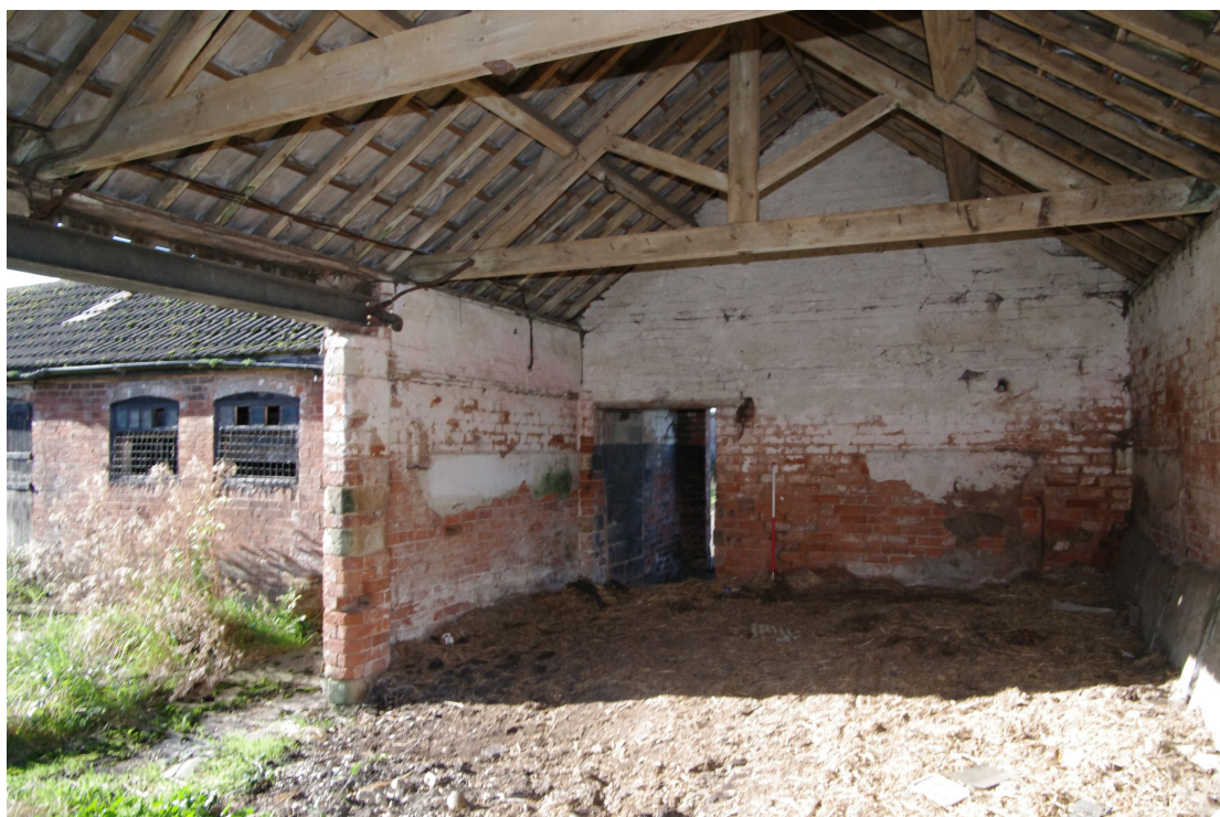
Figure 28 Internal view of Building 4
