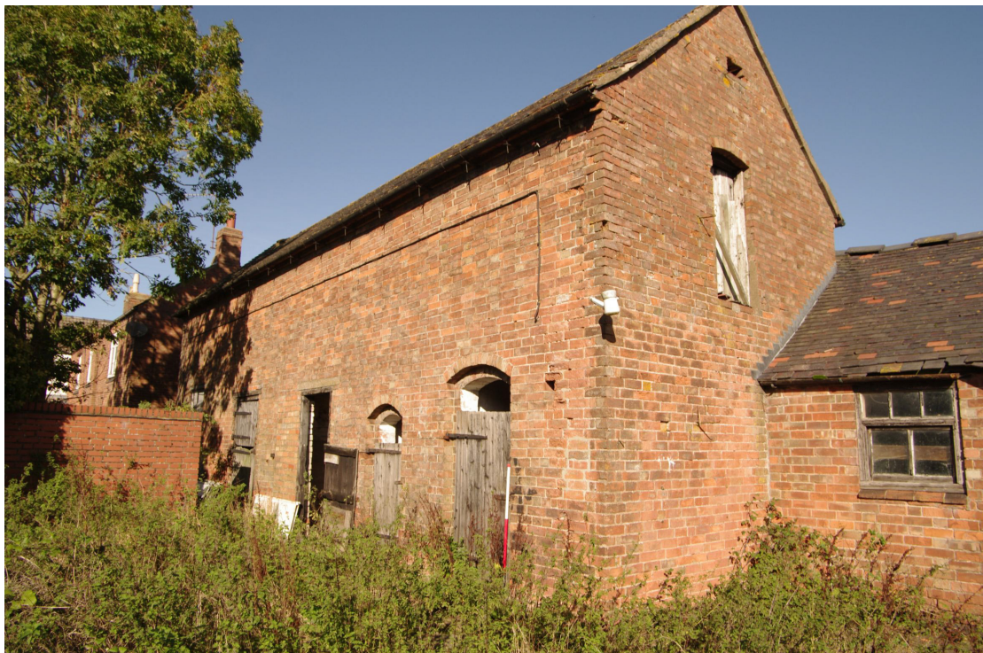
Figure 67 Building 7 south-west facing elevation of two storey range Looking north-east
