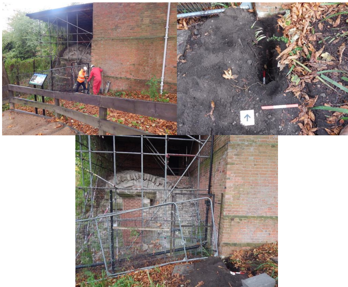
Figure 4: General view of external test pit
