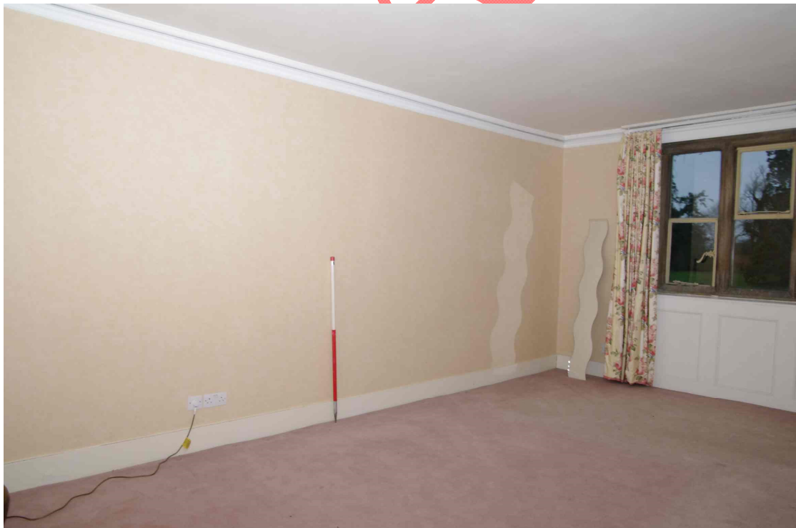
Figure 17 Dressing room and adjoining wall to the bathroom
