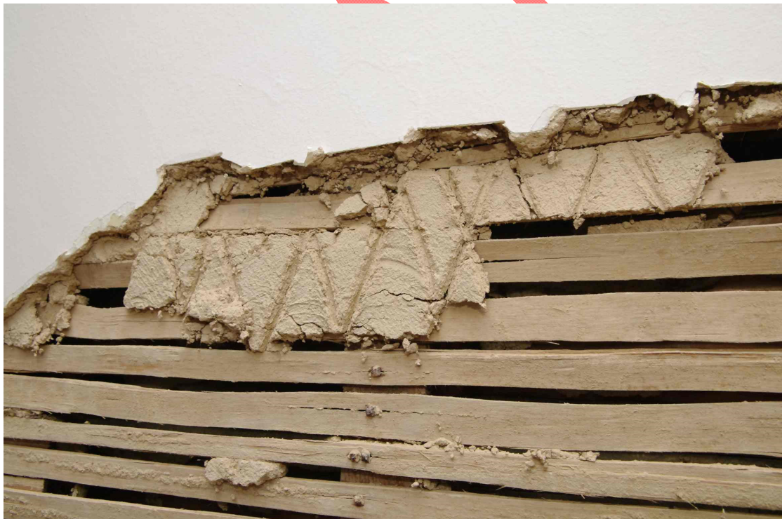
Figure 21 The two layers of plaster on the bathroom wall
