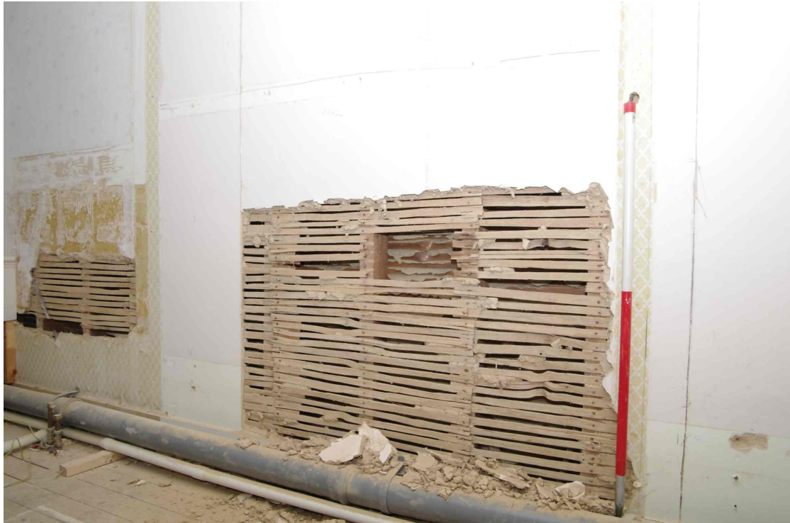
Figure 20 Initial removal of plaster in the bathroom Looking north-east. 1m scale
