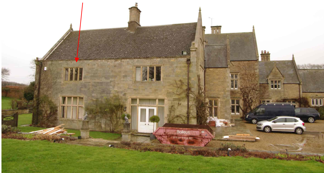
Figure 9 West facing elevation Looking north-east. Bathroom window is arrowed
