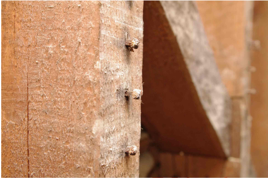
Figure 22 Nail detail used to hold laths
