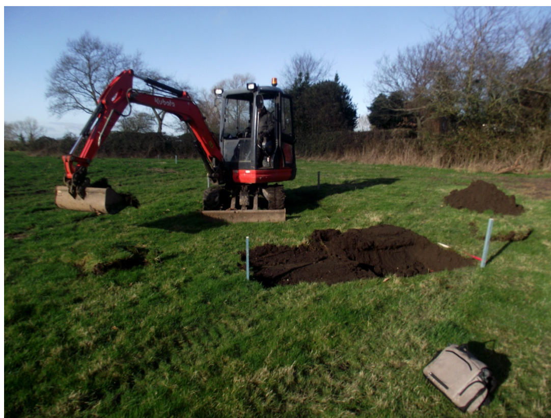
Figure 3: Excavation of wheel stand pits
