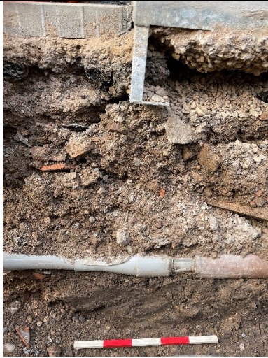
Figure 13: Deposit (4) under service pipe.
