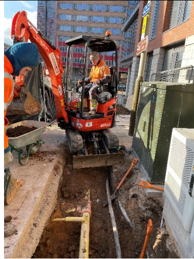
Figure 14: Working shot of digger.
