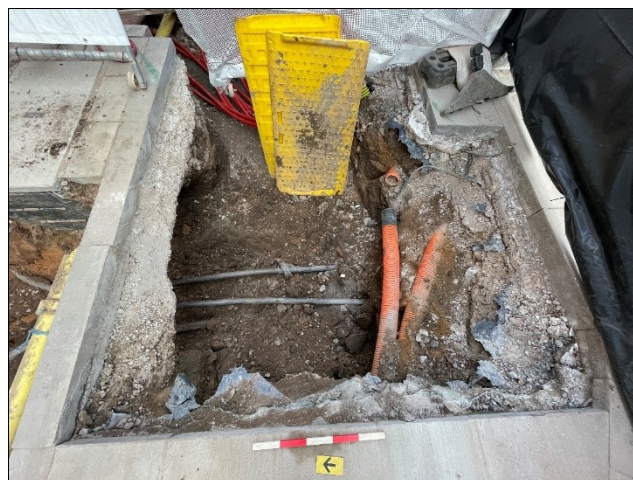
Figure 5: Area prior to the watching brief looking east.
