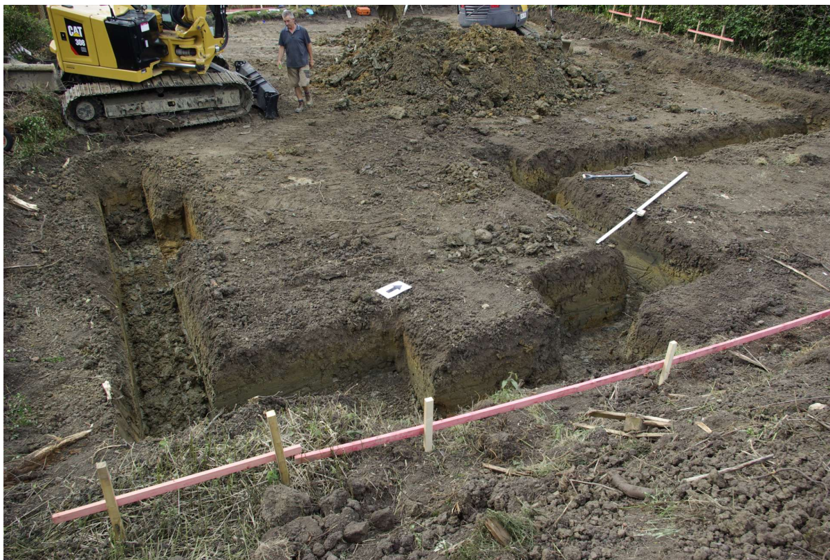
Figure 8 Post-excavation of the foundation trenches Looking north-west.
